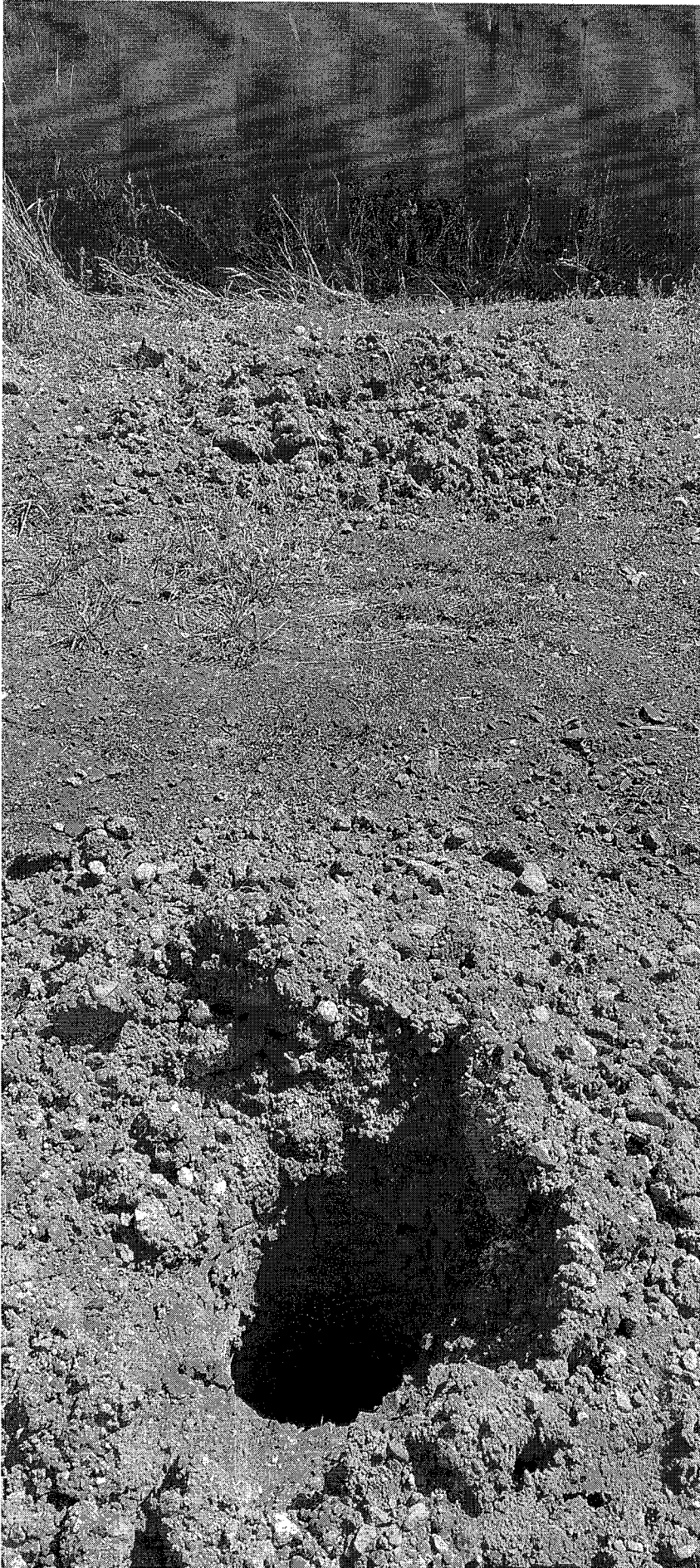
Condition # 7 Foundation Sona tube holes / office Building
