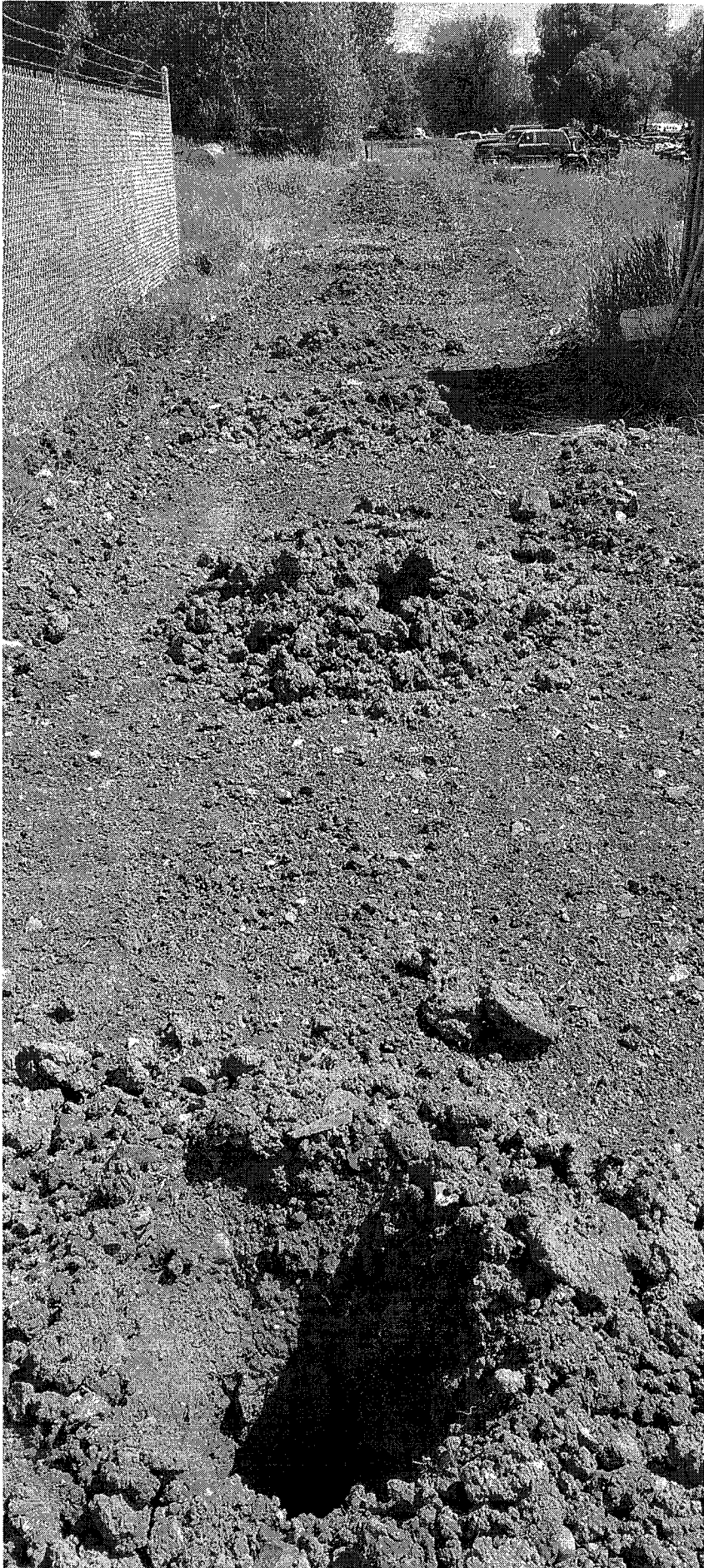
Condition #1 Post holes / Fence line
