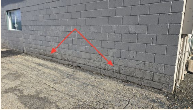
failing paint
