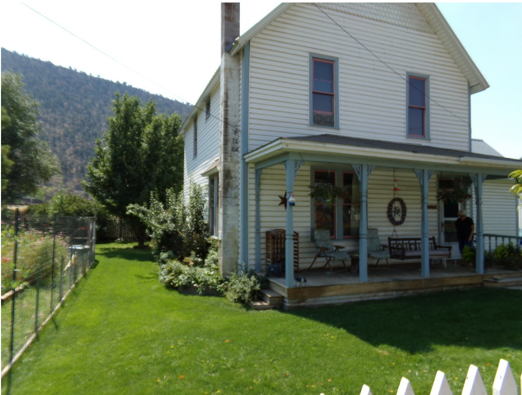
Photo Number: 5GF.5897_2 Description: Looking at the east and primary (north) elevations of the building. Date: 9/6/2022 View: Southwest
