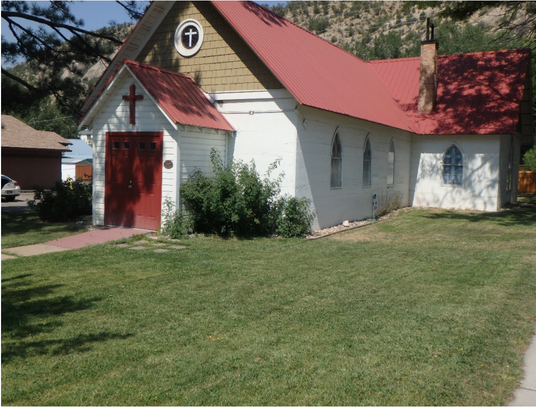
Photo Number: 5GF.2368_1 Description: Looking at the primary (south) and east elevations of the building. Note the historic brick masonry chimney; exposed rafter tails under the eaves; and the gothic arch window units. Date: 9/6/2022 View: Northwest
