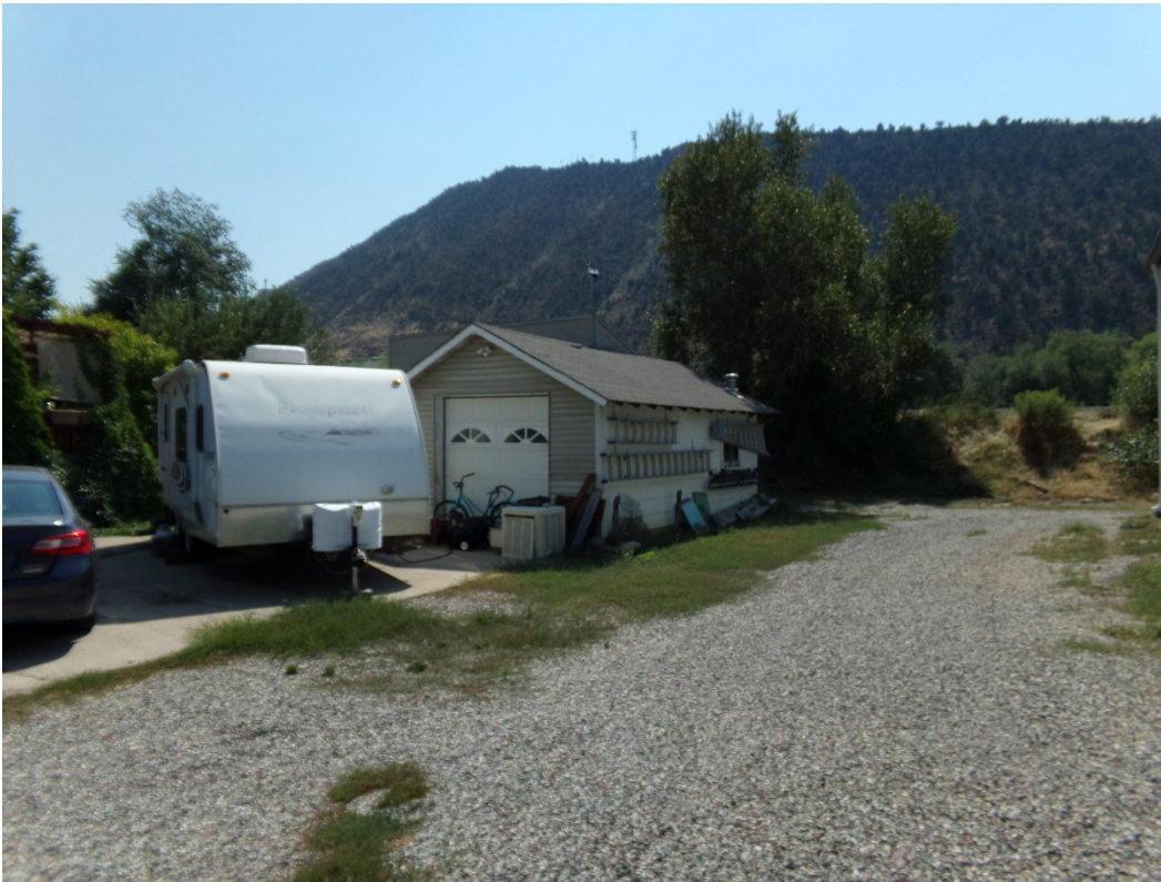
Photo Number: 5GF.5897_5 Description: Looking at the primary (north) and west elevations of the detached garage. Date: 9/6/2022 View: Southeast
