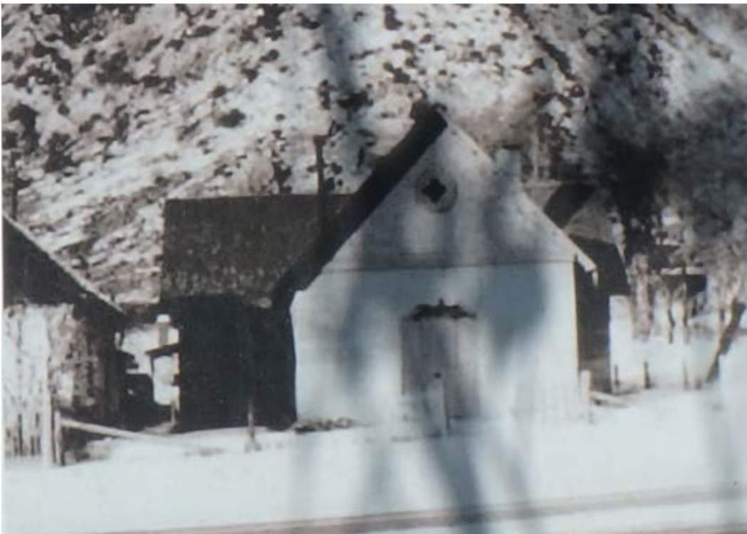
Historic Photo 1 Description: Looking at the primary (south) elevation of the church. Note that the front gable bay was not extant at the time, yet the oxeye, brick masonry chimney, and wood shingles in the gable end are extant. Date: Unknown; likely early-Twentieth Century Source: "New Castle Museum on the Street" sign along primary (south) elevation of the church
