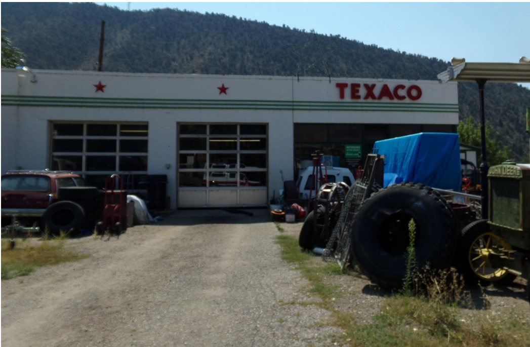
Photo Number: 5GF.5903_1 Description: Looking at the primary (north) elevation of the building from West Main Street. Note the rolled glazed doors in front of the service bays. Date: 9/6/2022 View: South
