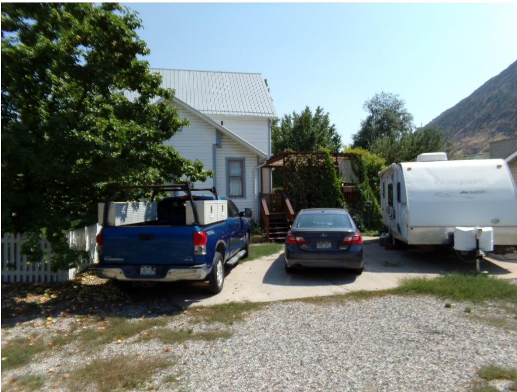
Photo Number: 5GF.5897_4 Description: Looking at the west elevation of the building. Note that the deck is along the south elevation. Date: 9/6/2022 View: East
