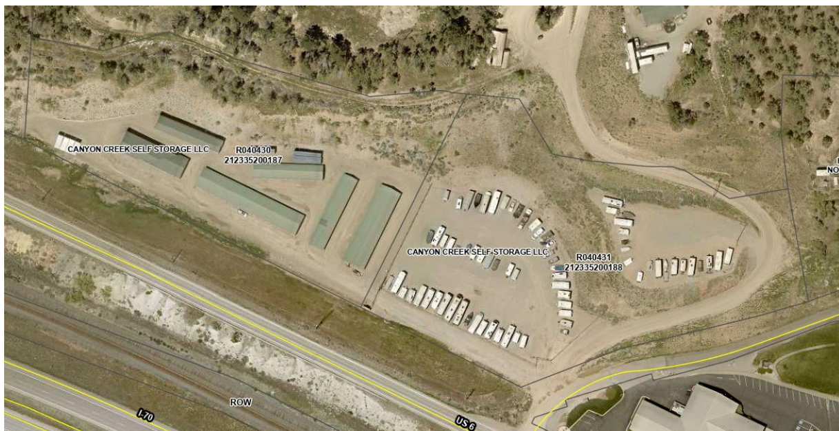
Canyon Creek Self Storage
