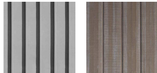
Standing Seam Roof Vertical Siding 2
