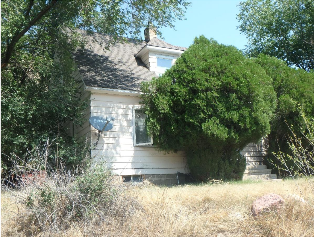
Photo Number: 5GF.5924_2 Description: Looking at the west and primary (south) elevation of the building. Date: 9/6/2022 View: Northeast
