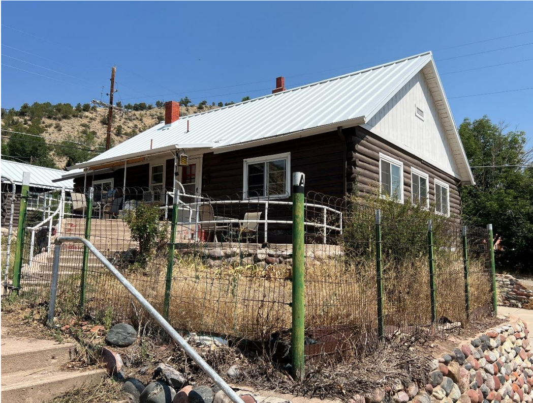
Photo Number: 5GF.5932_2 Description: Looking at the primary (west) and south elevations of the building. Date: 9/6/2022 View: Northeast
