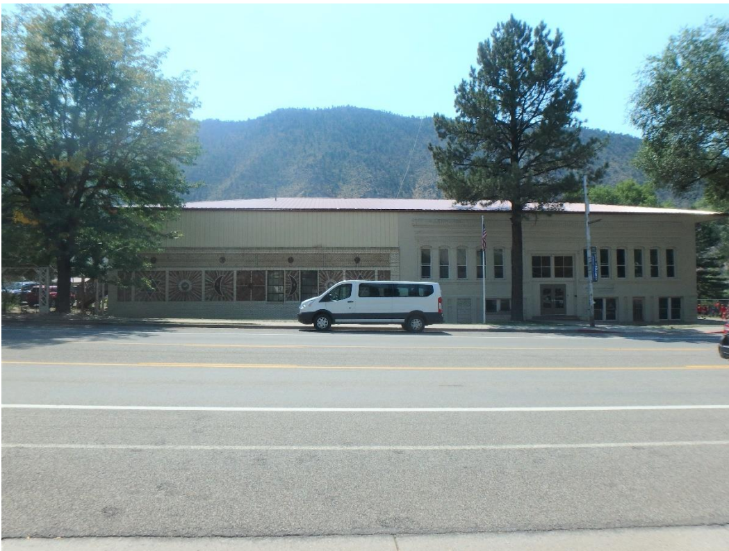
Photo Number: 5GF.2369_2 Description: Looking at the primary (north) elevation of the building. Date: 9/6/2022 View: South
