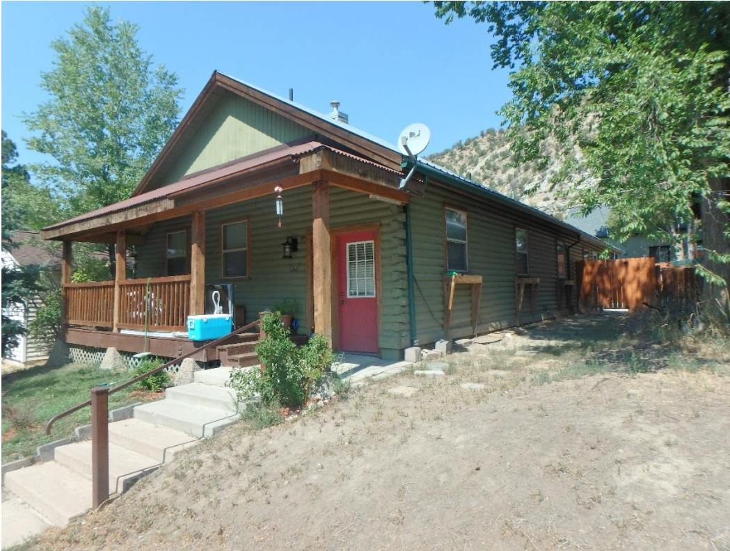
Photo Number: 5GF.5922_2 Description: Looking at the primary (south) and east elevations of the building. Date: 9/6/2022 View: Northwest
