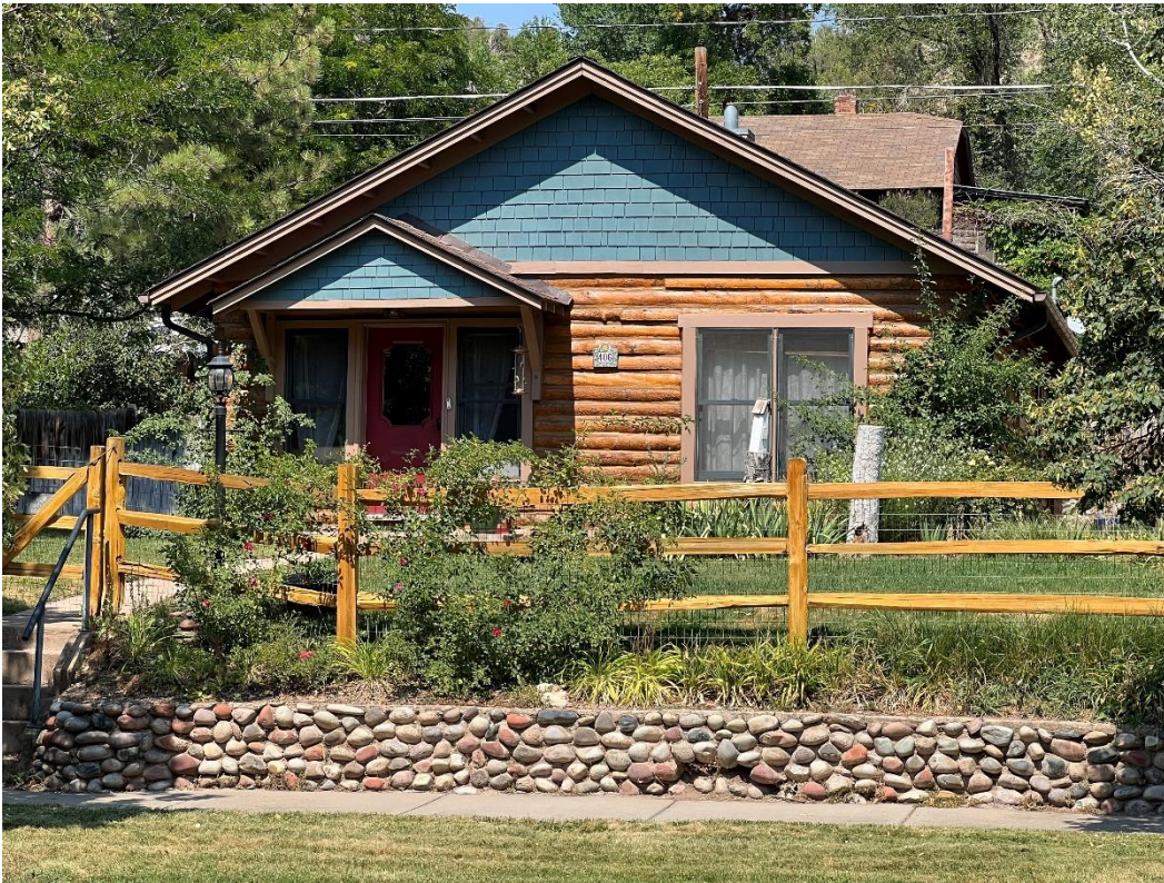
Photo Number: 5GF.5935_1 Description: Looking at the primary (south) elevation of the building. Note the decorative stone masonry wall, and the post and rail fencing. Date: 9/6/2022 View: North
