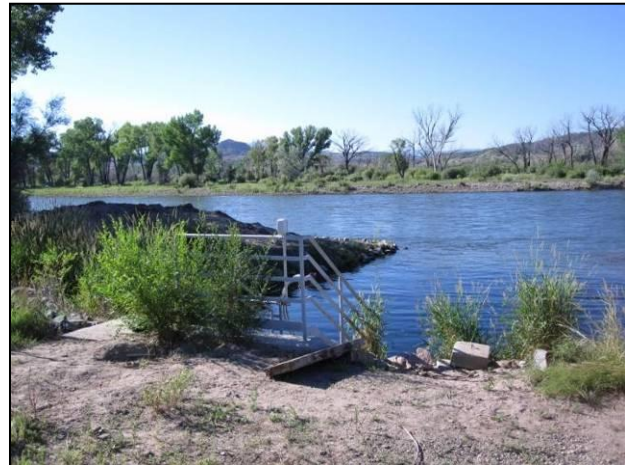
Figure 7: Town of Silt Colorado River Intake
