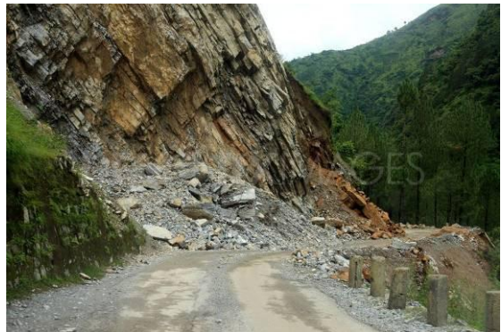
Figure 29: Landslide on Roadway. Source: www.demotix.com/news
