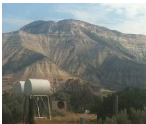
Figure 35: Residential aboveground storage tanks near Town of Parachute
