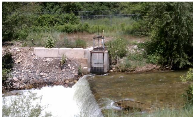
Figure 5: East Elk Creek Intake
