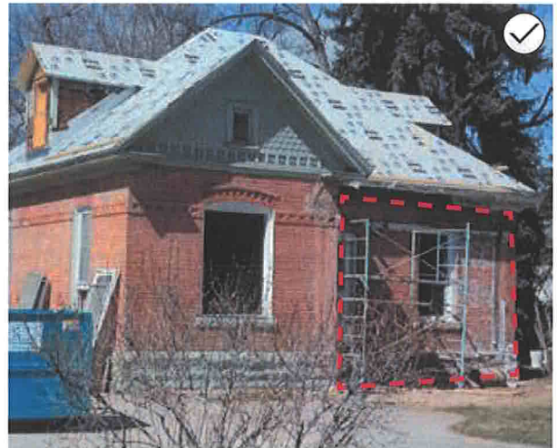
60. Minimize damage to historic structures when demolishing non-contributing additions or features. A non-historic addition was removed from the façade illustrated at left, allowing the original exterior to be repaired. A non-historic porch was carefully removed from the front of the house illustrated at right.
