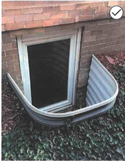
19. Locate a new basement egress window to be as inconspicuous as possible.
