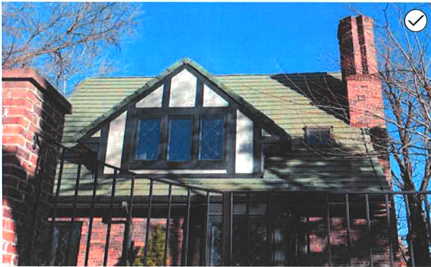
29. Match roof replacement materials to the historic roof materials whenever possible.
