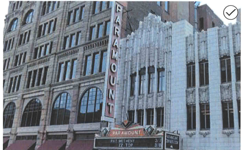
55. Preserve the overall rhythm and arrangement of windows on a historic commercial building façade.
