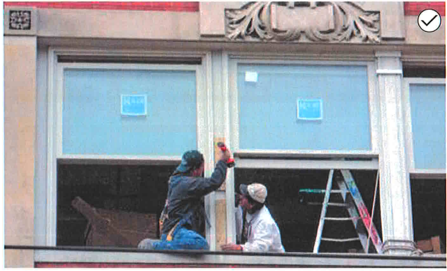
21. When replacement of an original window is necessary, match the replacement design to the original.
