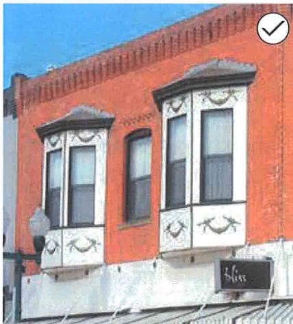
11. Preserve significant stylistic and architectural features, such as bay windows and masonry detailing.
