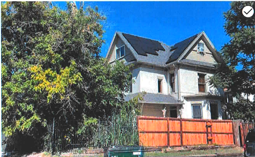
40. Solar panels are placed to avoid obscuring distinctive roof features.
