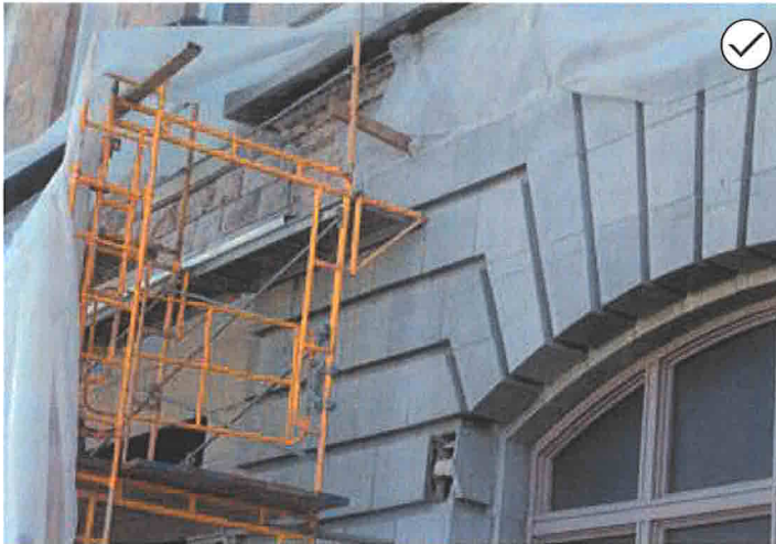
60. Minimize damage to historic structures when demolishing non-contributing additions or features. A non-historic addition was removed from the façade illustrated at left, allowing the original exterior to be repaired. A non-historic porch was carefully removed from the front of the house illustrated at right.
