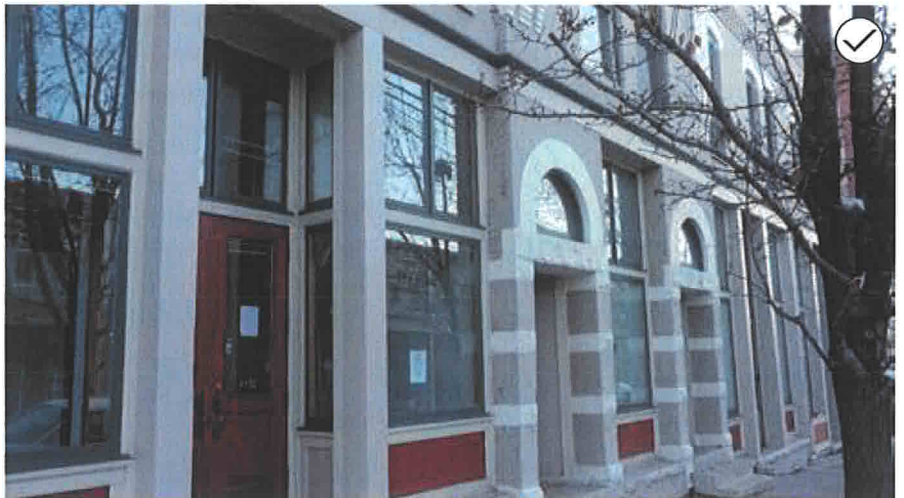
50. If necessary, replace windows with thermal pane glass, similar in appearance to the original, on a historic storefront.
