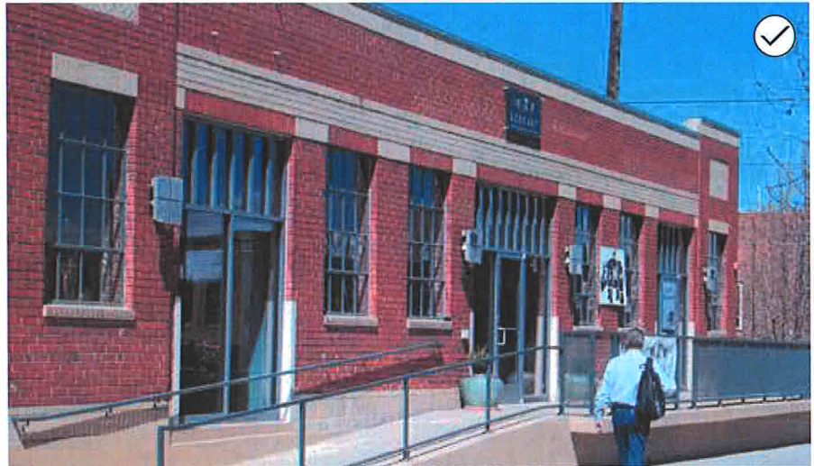
62. Select uses that are compatible with the original historic character of the building.
