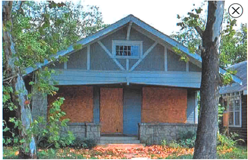
59. When closing off a window or door opening, paint the boards or panels to match the building color (left). Avoid mounting boards or panels on the exterior (right).
