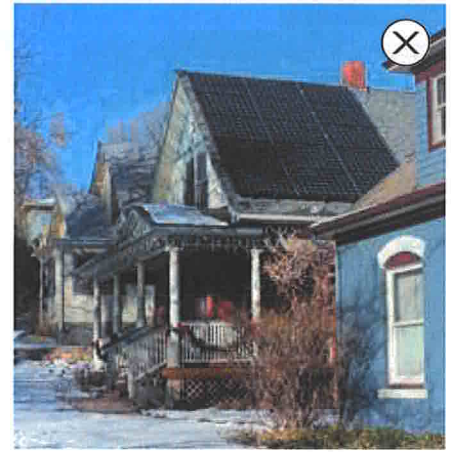
39. On a side-facing roof plane of a primary structure, minimize visual impacts by locating solar collectors at least 3 feet back from the front eave. The collectors illustrated above are not setback 3 feet.
