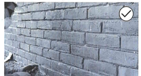
9. Re-point deteriorated masonry mortar joints.
