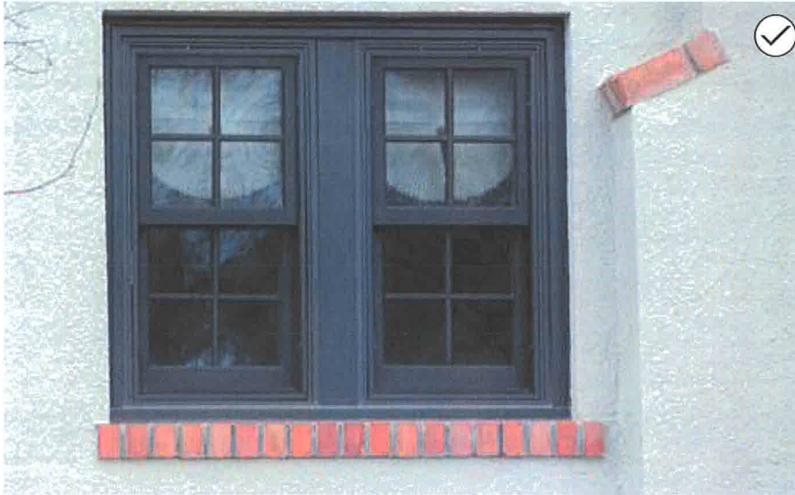
22. When replacement of an original window is necessary, match the replacement design as closely as possible.
