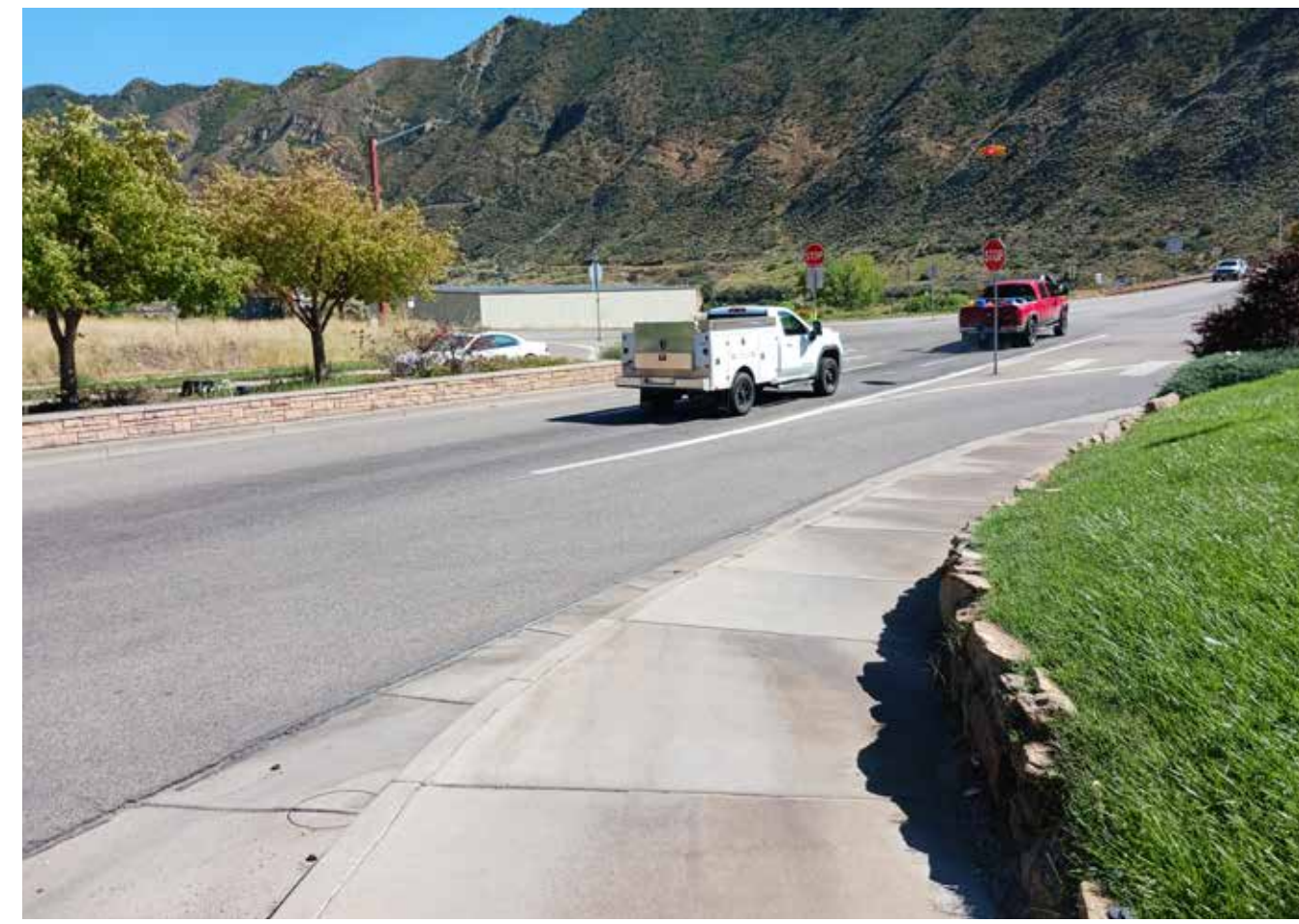
2. View of the intersection facing South.
