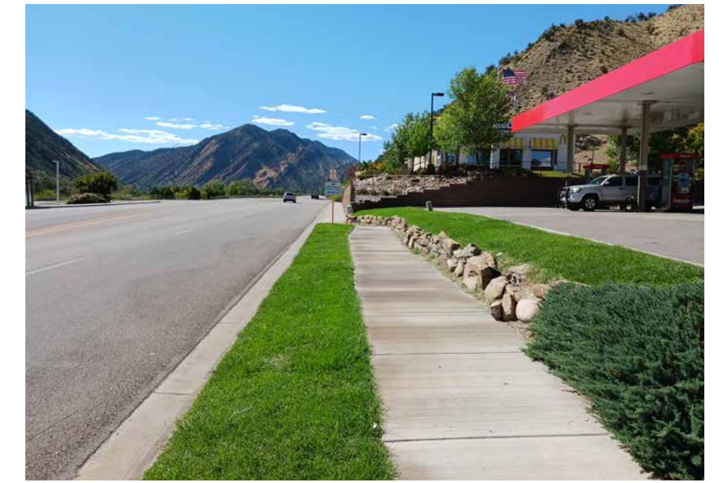
4. View of Hwy 6 facing West towards downtown New Castle.
