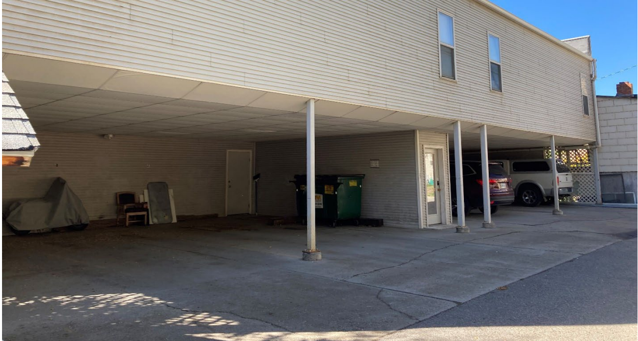
6 dwelling units in the Weller Building, downtown New Castle, CO.
