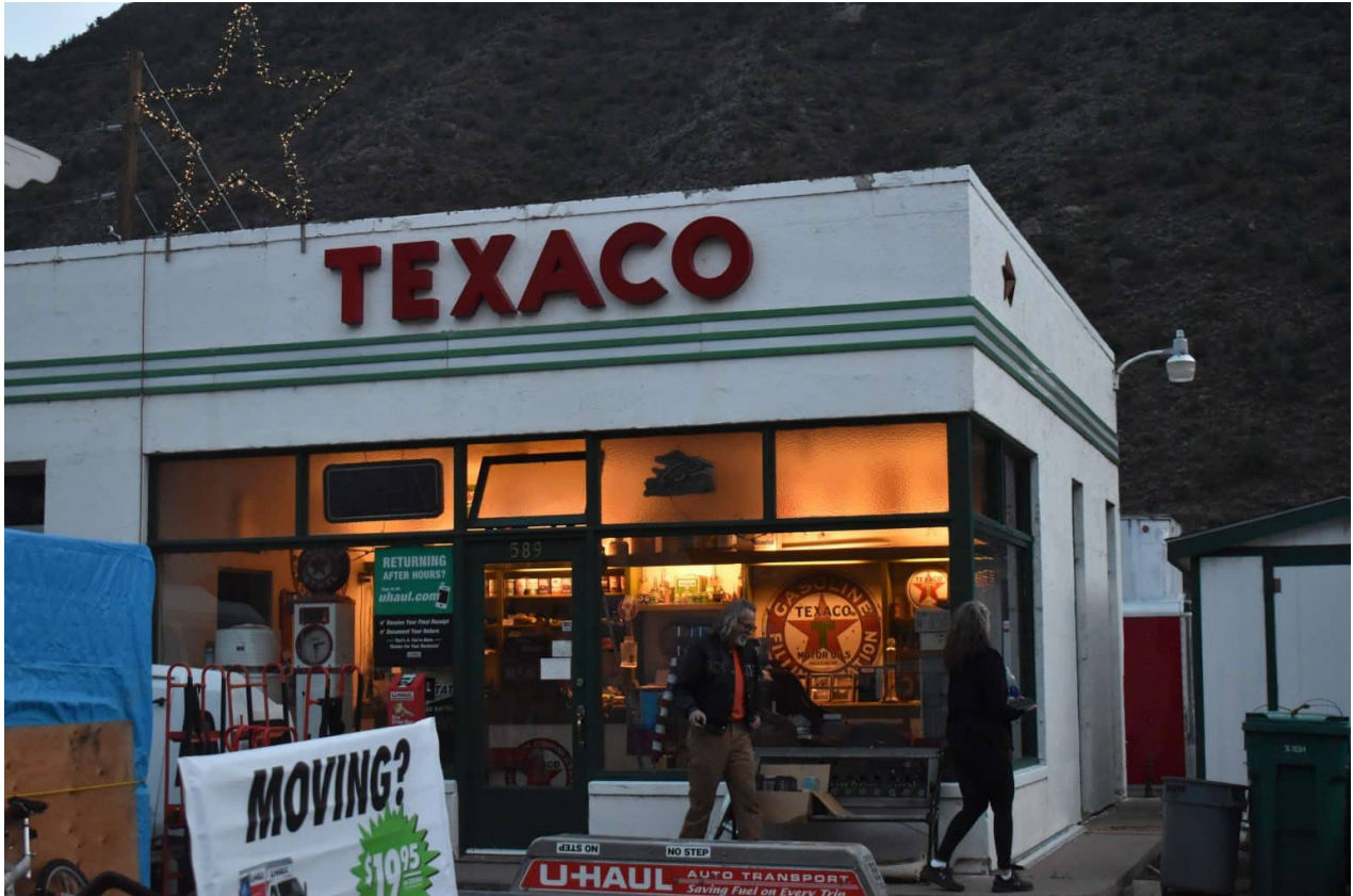
The exterior of the New Castle Garage.
