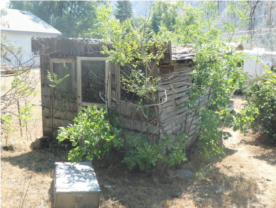
Photo Number: 5GF.5927_1 Description: Looking at the primary (north) and west elevations of the building. Note the wood shingle and horizontal weatherboard siding. Date: 9/6/2022 View: Southeast
