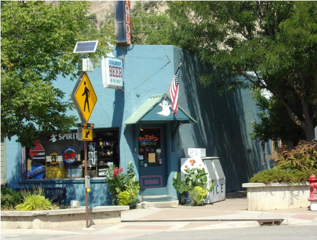
Photo Number: 5GF.2375_1 Description: Looking at the primary (south) and east elevations of the building. Date: 9/6/2022 View: Northwest
