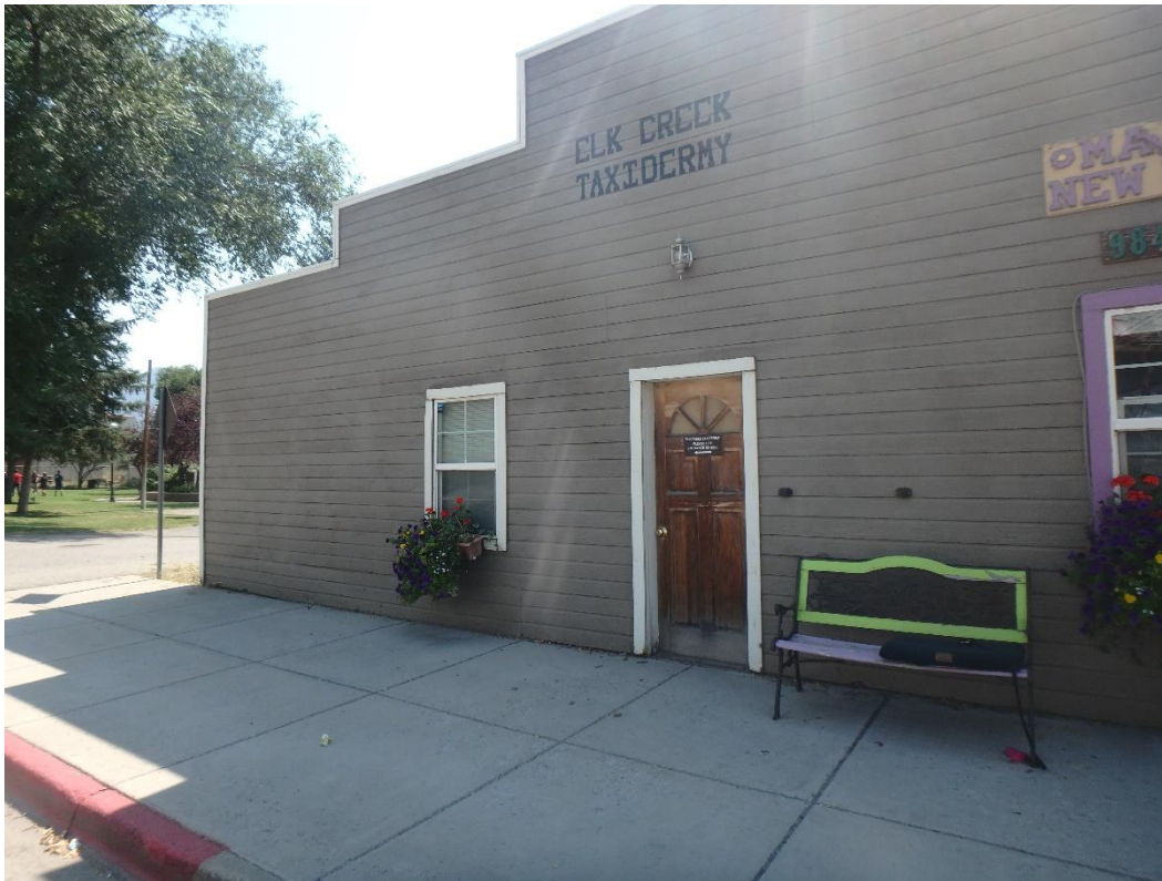
Photo Number: 5GF.5919_1 Description: Looking at the primary (north) elevation of the building. Note the false front that features a stepped parapet design. Date: 9/6/2022 View: Southeast
