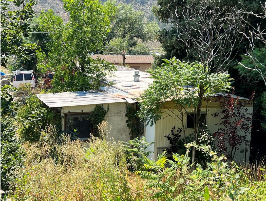
Photo Number: 5GF.5934_1 Description: Looking at the primary (east) and north elevations of the primary trailer. Date: 9/6/2022 View: Southwest
