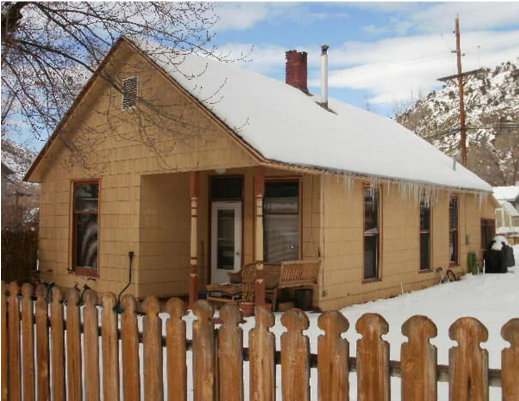
Reference Photo 1 Description: Looking at the primary (south) and east elevations of the building. This image is shortly before the alterations to the exterior envelope between 2012 and 2022. Date: circa 2009 Source: Garfield County Assessor's Office
