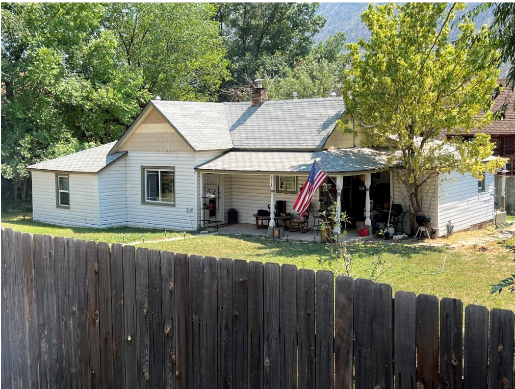
Photo Number: 5GF.5940_2 Description: Looking at the primary (north) and west elevations of the building. Date: 9/6/2022 View: Southeast
