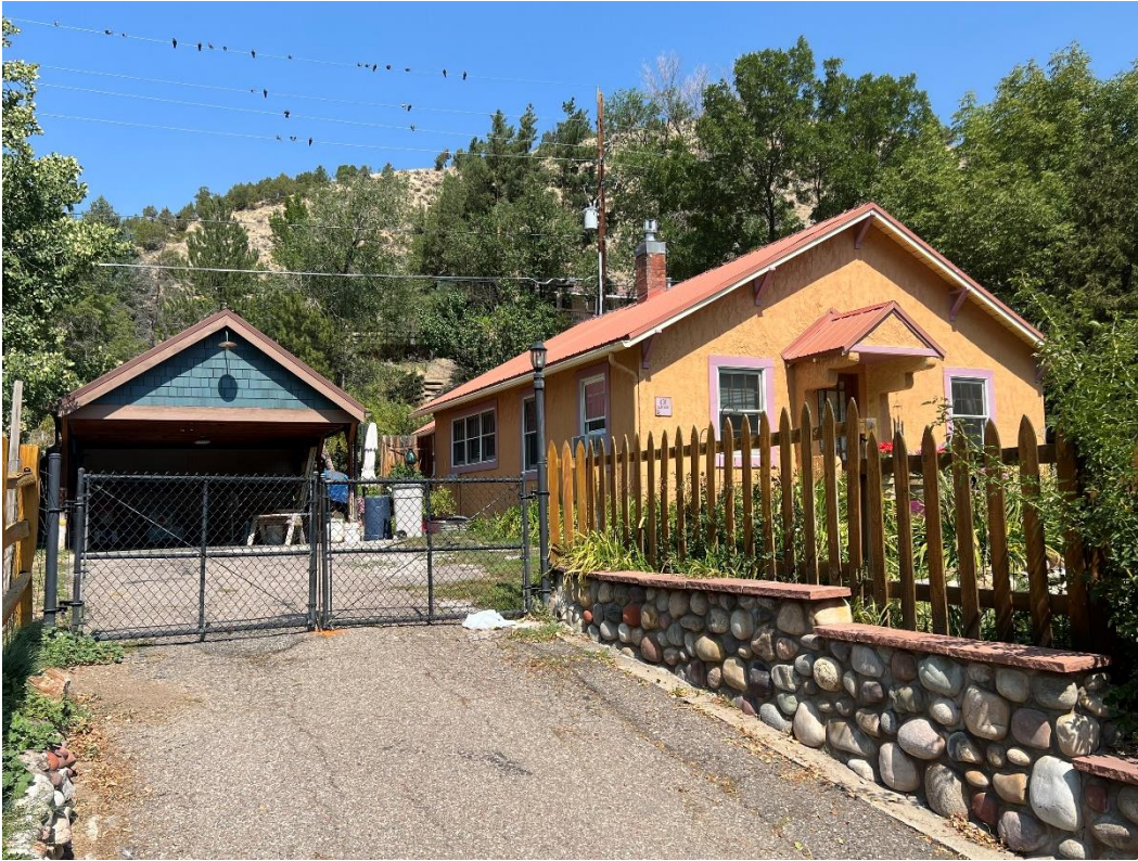
Photo Number: 5GF.5937_3 Description: Context view of the residence's west and primary (south) elevations. Note the stone masonry wall and wood picket fencing along the legal parcel boundary. Date: 9/6/2022 View: Northeast
