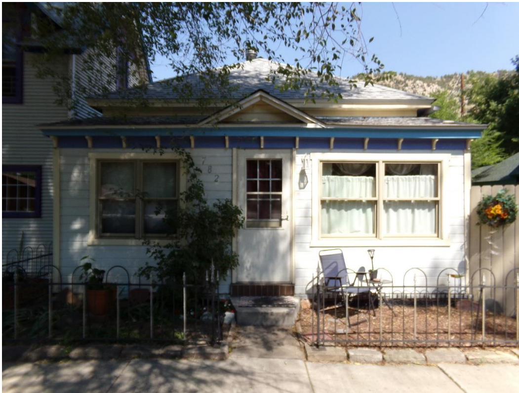
Photo Number: 5GF.5893_1 Description: Looking at the primary (south) elevation of the building. Date: 9/6/2022 View: North
