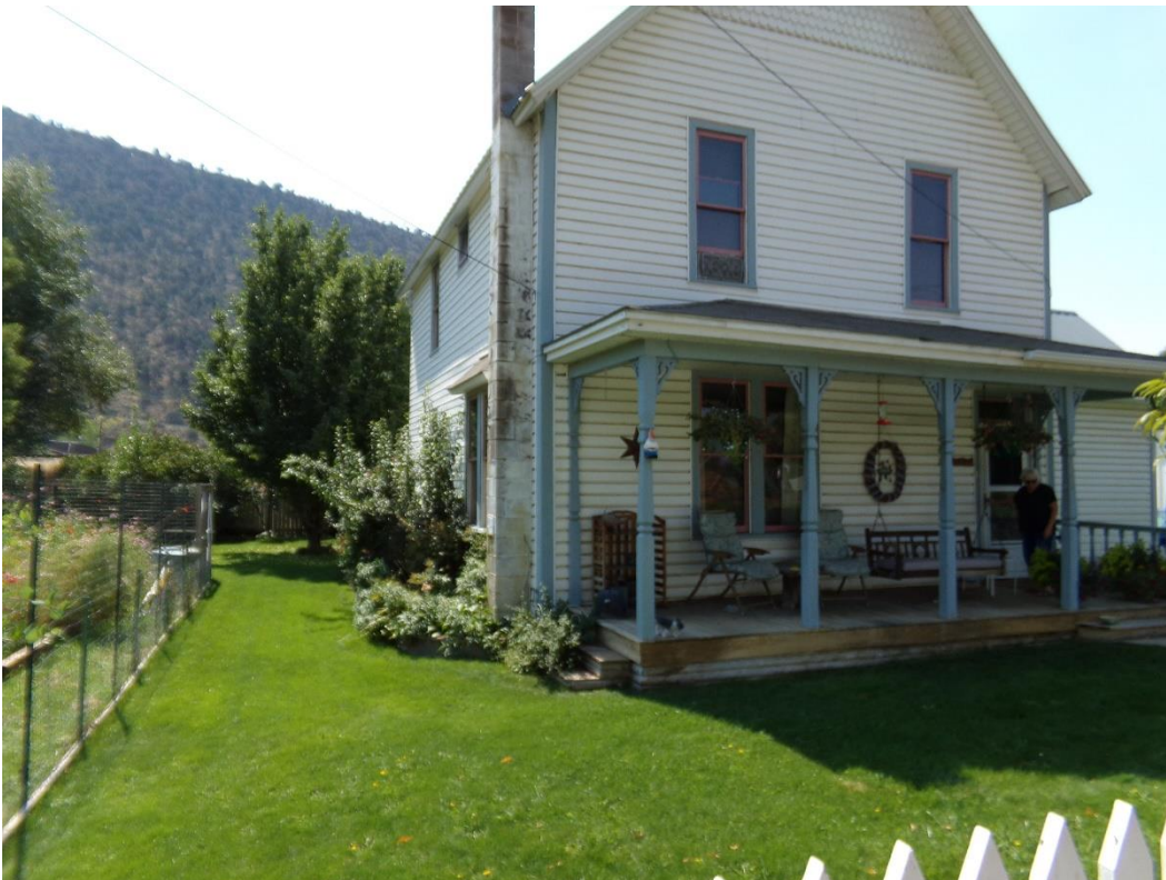
Photo Number: 5GF.5897_2 Description: Looking at the east and primary (north) elevations of the building. Date: 9/6/2022 View: Southwest
