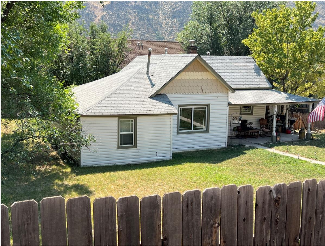
Photo Number: 5GF.5940_3 Description: Looking at the east and primary (north) elevations of the building. Date: 9/6/2022 View: Southwest
