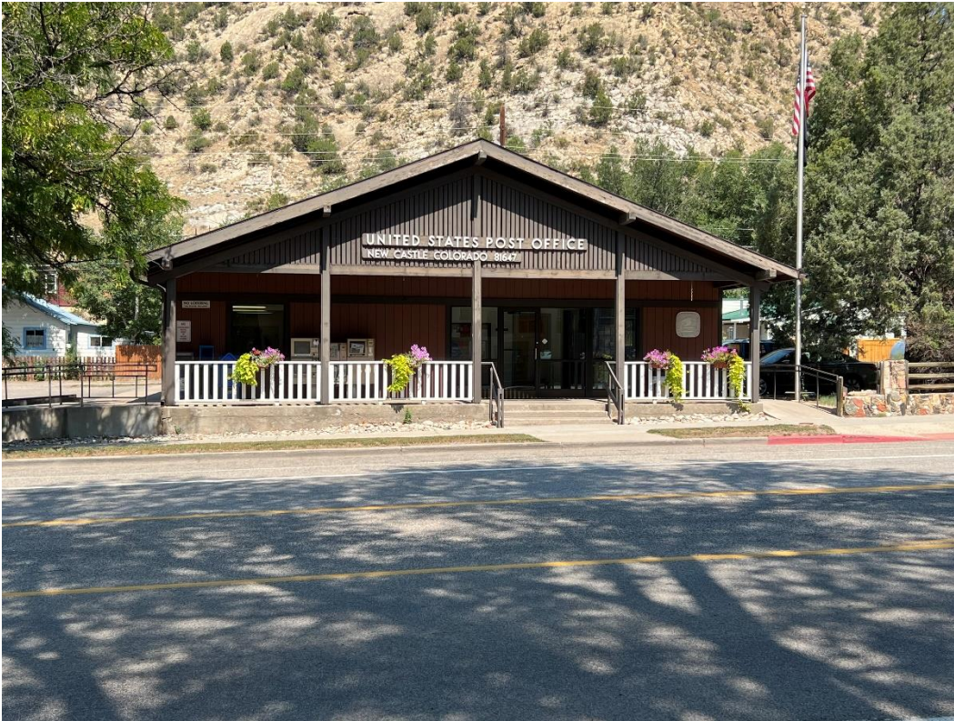
Photo Number: 5GF.5890_1 Description: Looking at the primary (south) elevation of the building. Date: 9/6/2022 View: North
