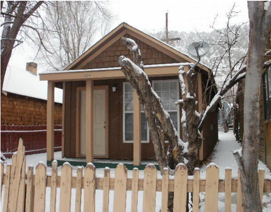
Reference Photo 1 Description: Looking at the primary (south) elevation. Date: Circa 2009 Source: Garfield County Assessor's Office
