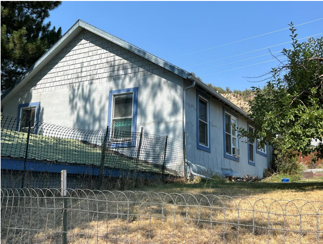
Photo Number: 5GF.5931_4 Description: Close up of the south and east elevations of the residence. Note the exposed rafter tails under the eaves that are partially obscured by the fascia board. Date: 9/6/2022 View: Northwest
