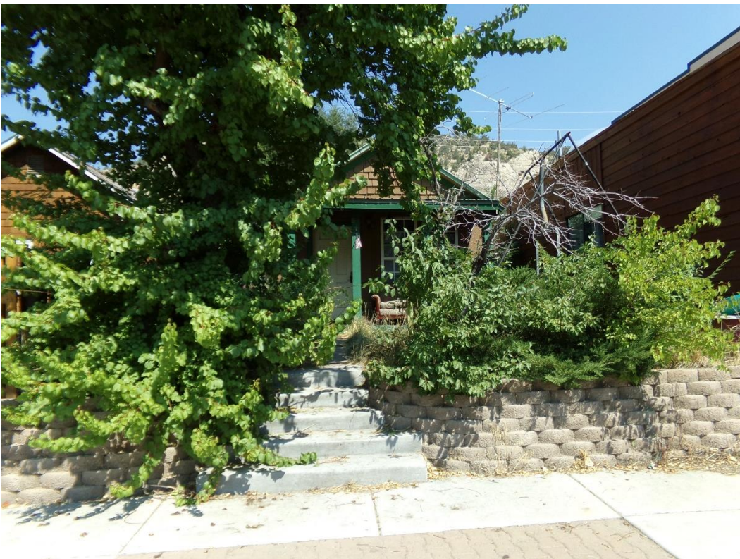
Photo Number: 5GF.5907_2 Description: Context view of the primary (south) elevation of the building. Date: 9/6/2022 View: North
