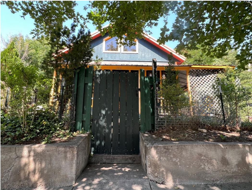
Photo Number: 5GF.5938_2 Description: Looking at the primary (south) elevation of the building. Note that much of the facade is observed by wood fencing and vegetation from the public ROW. Date: 9/6/2022 View: North
