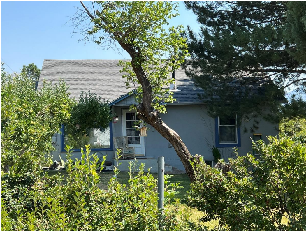
Photo Number: 5GF.5931_2 Description: Looking at the primary (west) elevation of the building. Date: 9/6/2022 View: East
