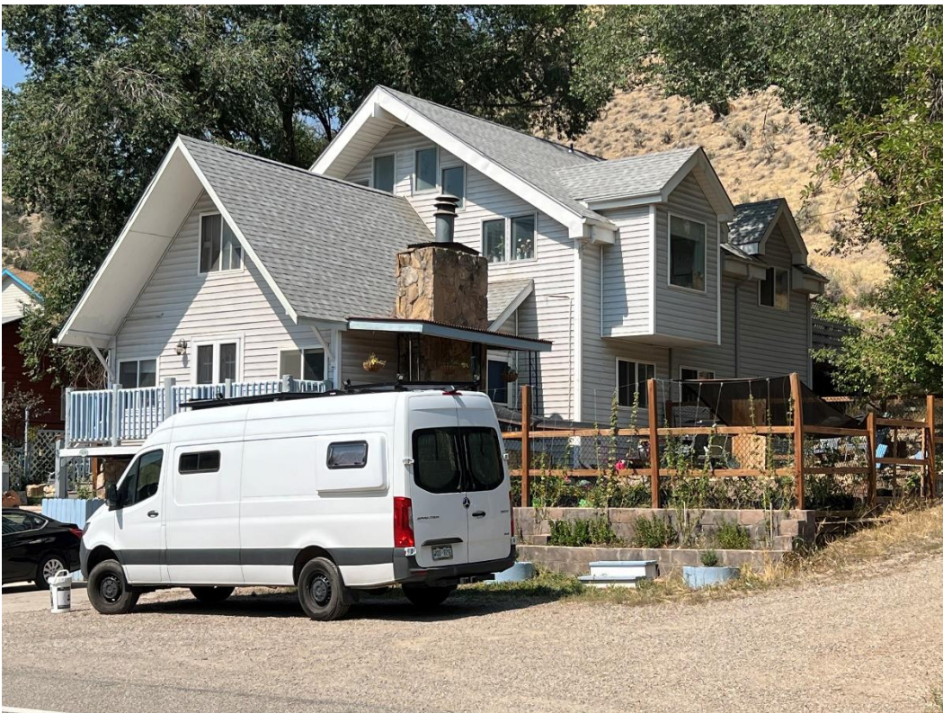
Photo Number: 5GF.5941_2 Description: Looking at the primary (south) and east elevations of the building. Date: 9/6/2022 View: Northwest
