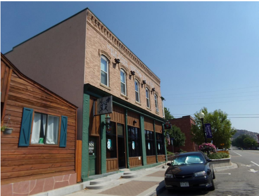
Photo Number: 5GF.1166_1 Description: Looking at the west and primary (south) elevation of the building. Date: 9/6/2023 View: Northeast
