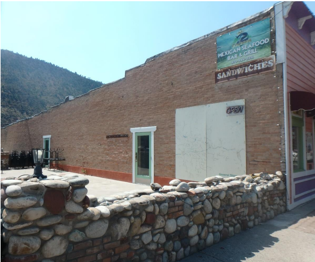
Photo Number: 5GF.2371_2 Description: Looking at the east elevation of the building. Date: 9/6/2022 View: Southwest
