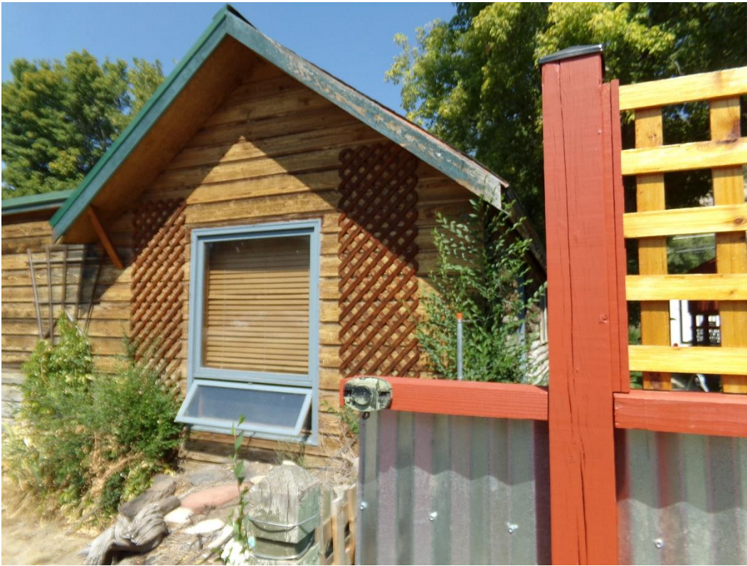
Photo Number: 5GF.5896_3 Description: Looking at the right side of the south elevation of the building. Date: 9/6/2022 View: Northwest
