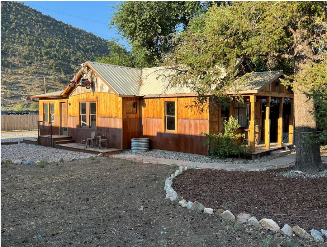
Photo Number: 5GF.5910_3 Description: Looking at the east and primary (north) elevations of the building. Date: 9/6/2022 View: Southwest
