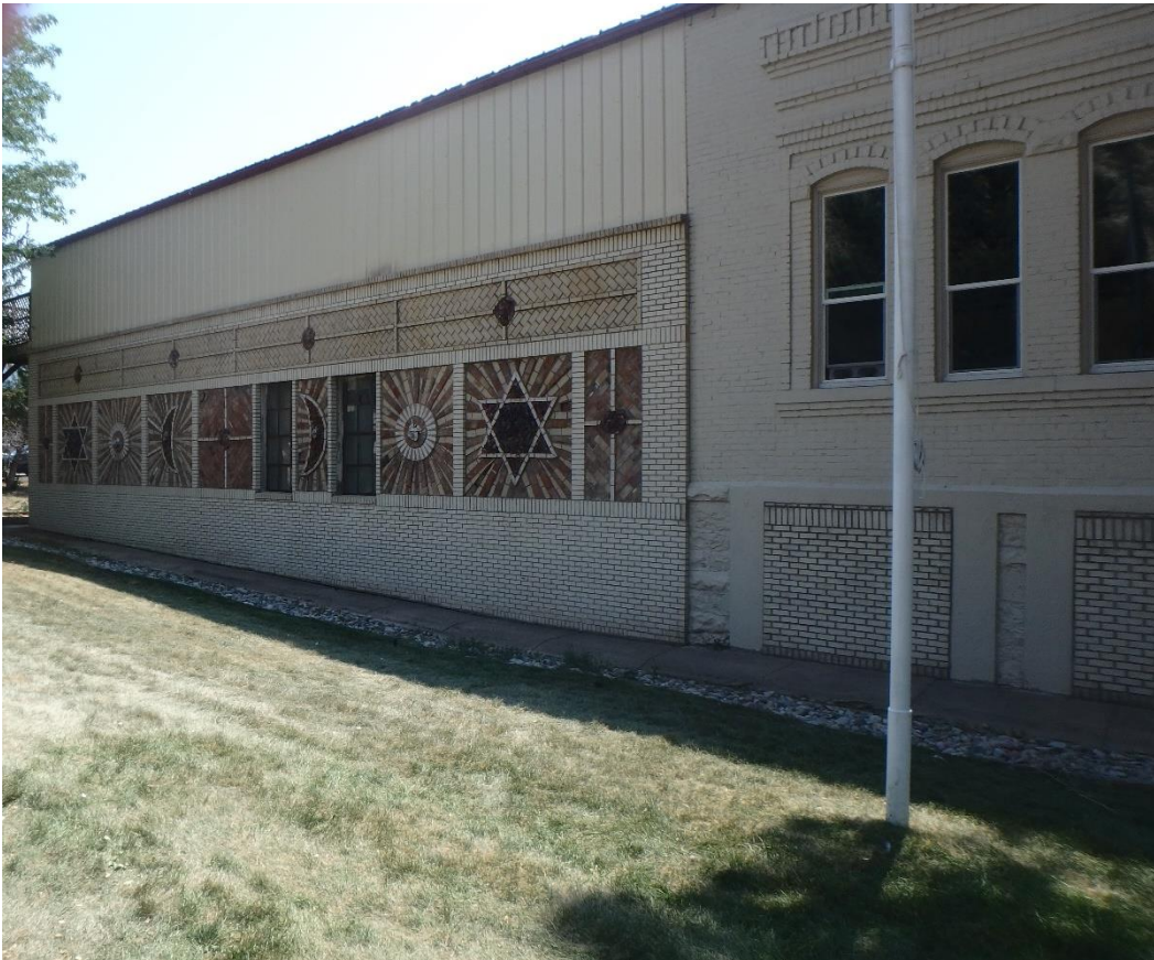
Photo Number: 5GF.2369_3 Description: Looking at the 1939 adobe brick addition to the original 1913 building. Date: 9/6/2022 View: Southeast
