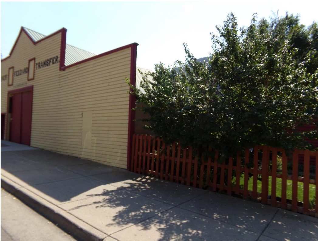
Photo Number: 5GF.2380_2 Description: Looking at the primary (north) and west elevation of the building; though, the west elevation is obscured by vegetation. Date: 9/6/2022 View: Southeast
