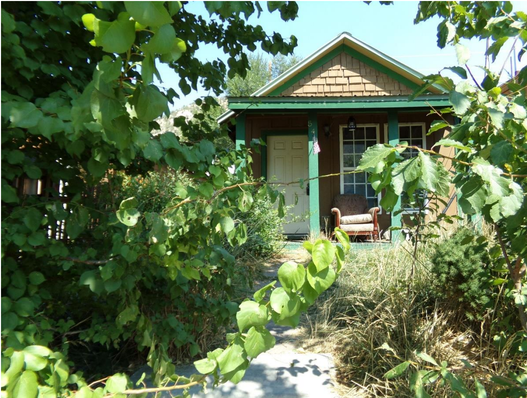
Photo Number: 5GF.5907_1 Description: Looking at the primary (south) elevation of the building. Date: 9/6/2022 View: North
