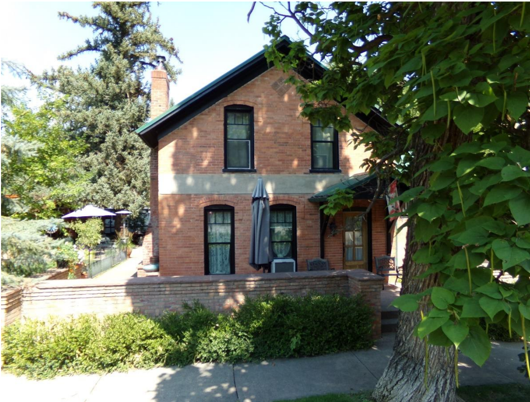
Photo Number: 5GF.5891_1 Description: The primary (south) elevation of the building. Date: 9/6/2022 View: North
