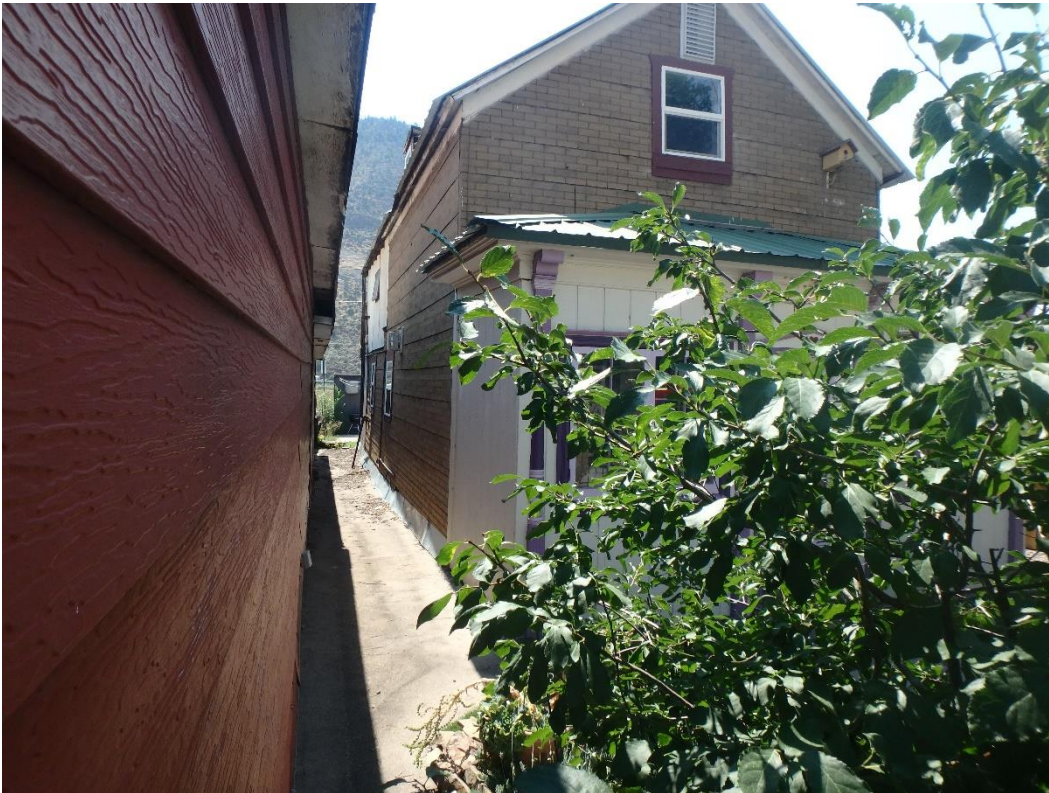
Photo Number: 5GF.2370_3 Description: Looking at the east and primary (north) elevations of the building. Date: 9/6/2022 View: Southwest
