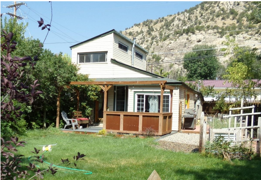
Photo Number: 5GF.5901_2 Description: Looking at the primary (south) and east elevation of the building. Date: 9/6/2022 View: Northwest
