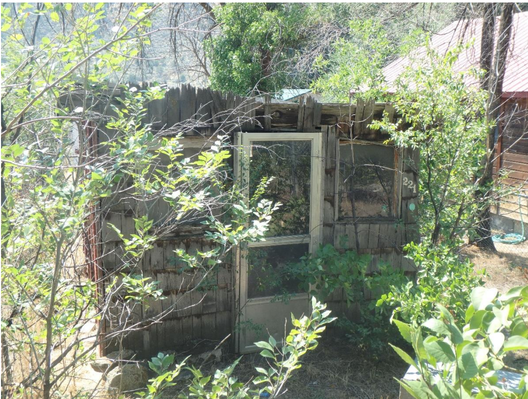
Photo Number: 5GF.5927_2 Description: Looking at the primary (north) elevation of the building. Date: 9/6/2022 View: South
