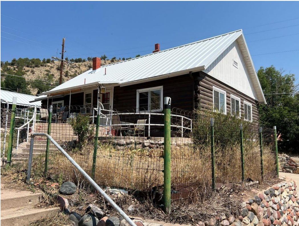
Photo Number: 5GF.5932_2 Description: Looking at the primary (west) and south elevations of the building. Date: 9/6/2022 View: Northeast
