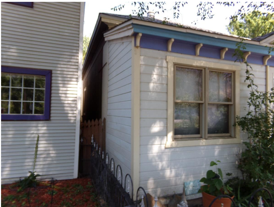
Photo Number: 5GF.5893_2 Description: Looking at the west and left side of the primary (south) elevation of the building. Date: 9/6/2022 View: Northeast
