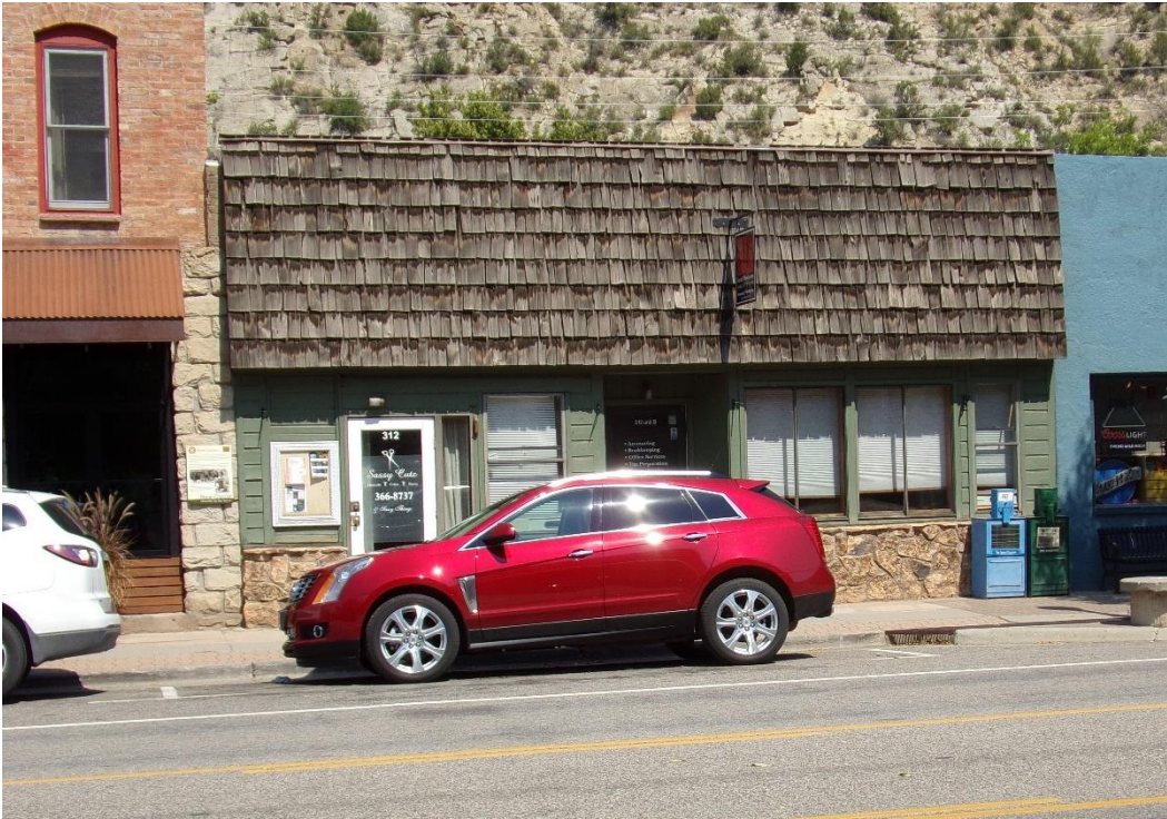
Photo Number: 5GF.2377_1 Description: Looking at the primary (south) elevation of the building. Date: 9/6/2022 View: North
