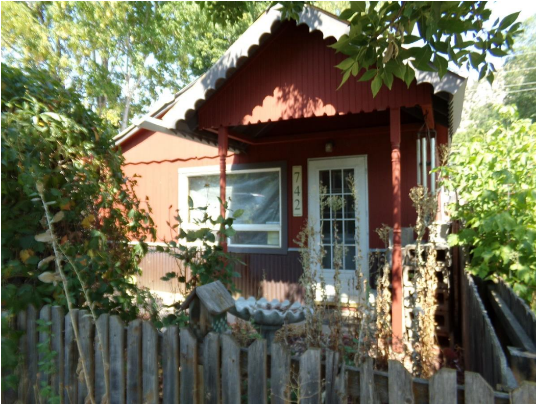
Photo Number: 5GF.5895_1 Description: Looking at the primary (south) elevation of the building. Date: 9/6/2022 View: Northwest
