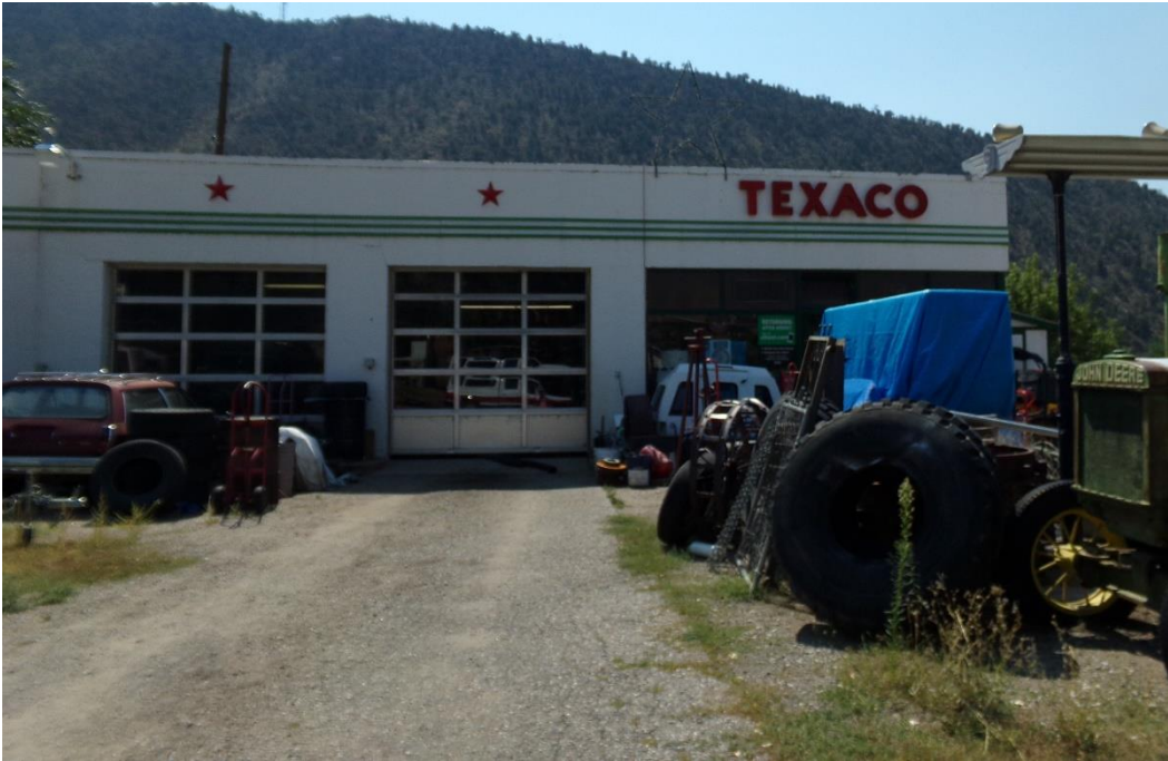
Photo Number: 5GF.5903_1 Description: Looking at the primary (north) elevation of the building from West Main Street. Note the rolled glazed doors in front of the service bays. Date: 9/6/2022 View: South
