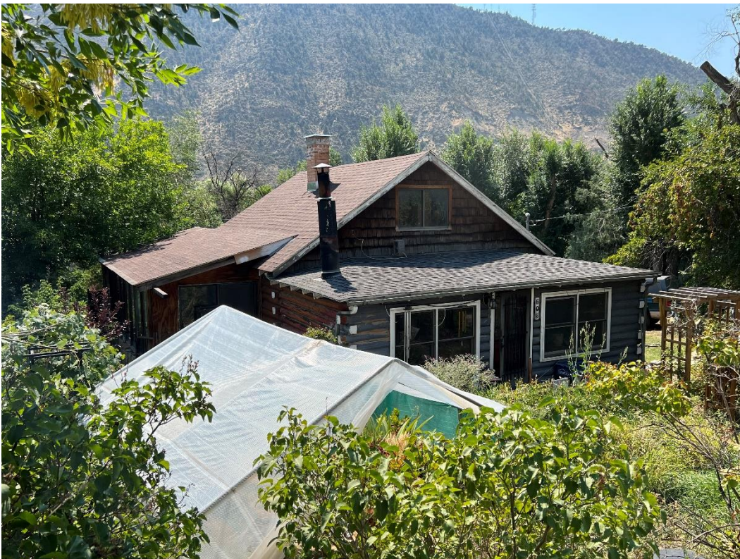
Photo Number: 5GF.5939_2 Description: Looking at the east and primary (north) elevations of the building. Date: 9/6/2022 View: Southwest
