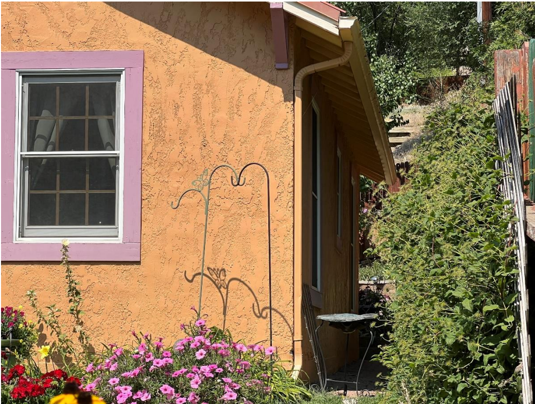
Photo Number: 5GF.5937_4 Description: Looking at the east elevation of the building. The building's proximity to the wall on the right makes it difficult to observe the entire elevation. Date: 9/6/2022 View: Northwest
