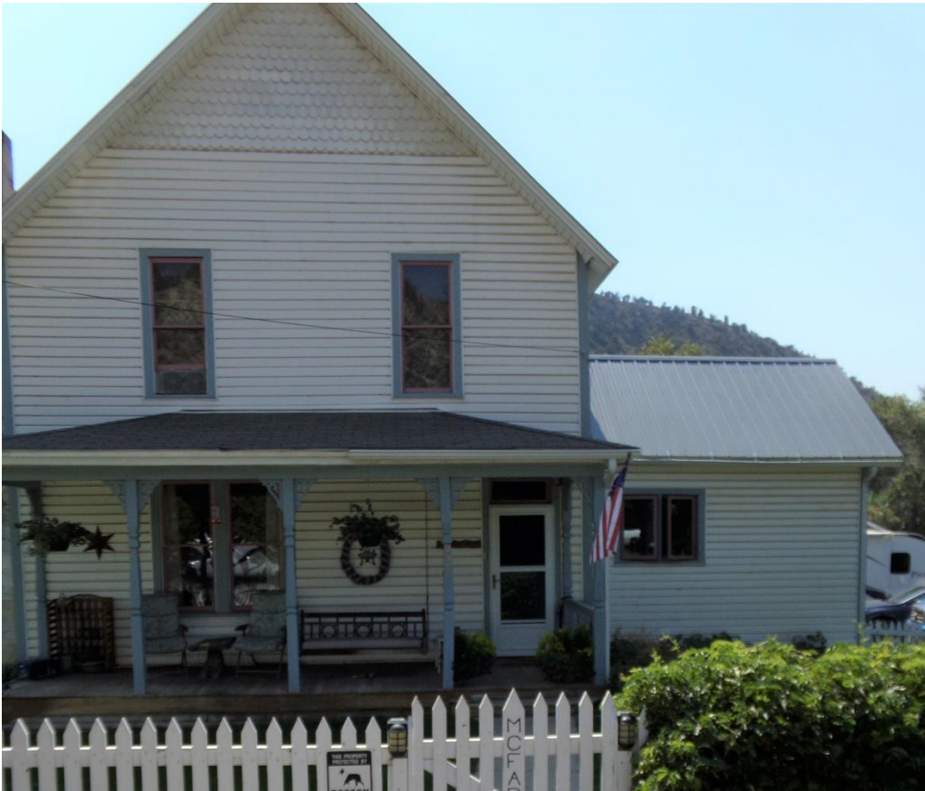
Photo Number: 5GF.5897_3 Description: Looking at the primary (north) elevation of the building. Date: 9/6/2022 View: South
