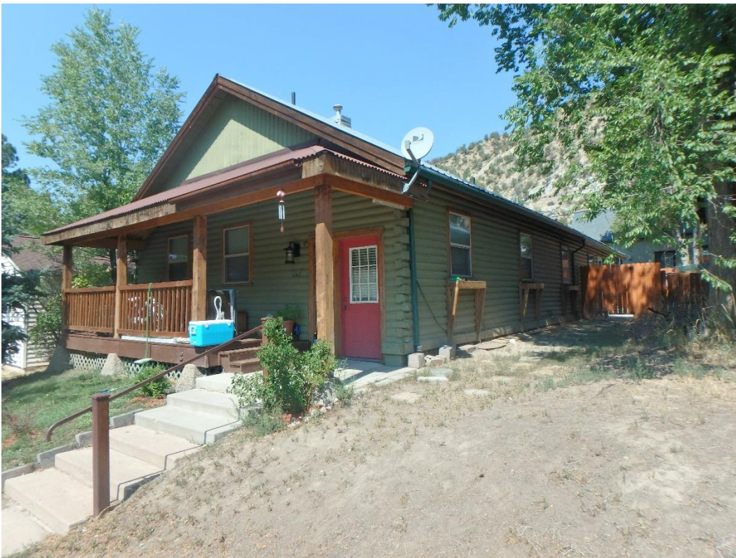
Photo Number: 5GF.5922_2 Description: Looking at the primary (south) and east elevations of the building. Date: 9/6/2022 View: Northwest
