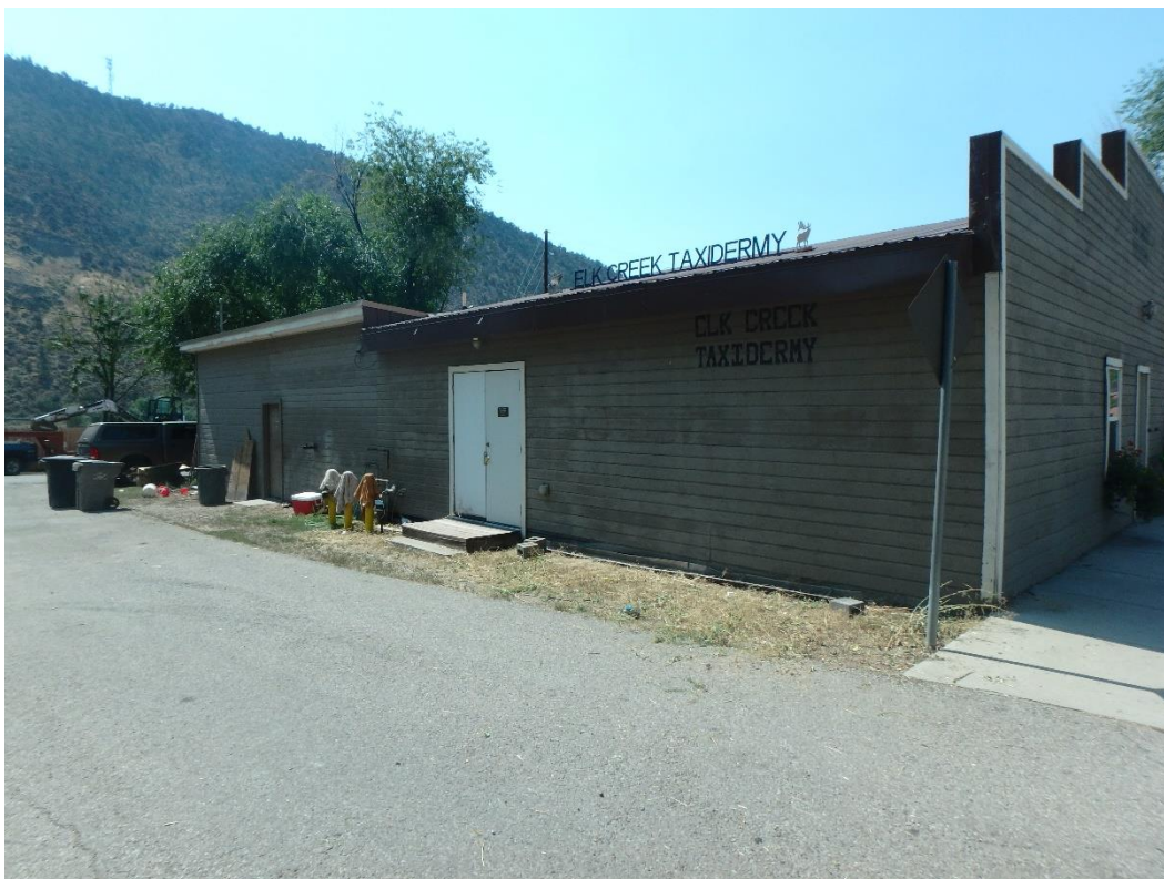
Photo Number: 5GF.5919_2 Description: Looking at the east and primary (north) elevations of the building. Date: 9/6/2022 View: Southwest
