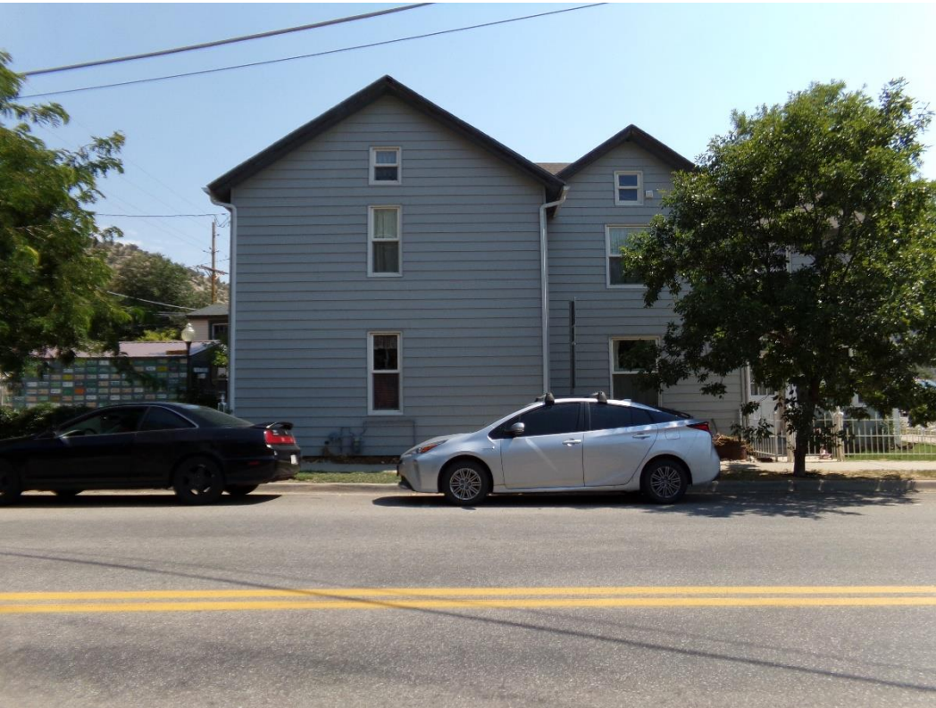
Photo Number: 5GF.5900_4 Description: Looking at the west elevation of the building. Date: 9/6/2022 View: East
