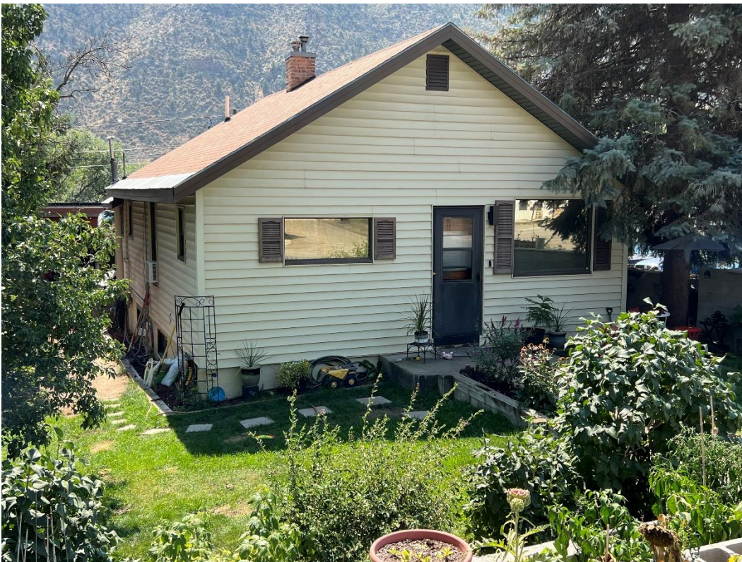
Photo Number: 5GF.5933_2 Description: Looking at the east and primary (north) elevation of the building. Date: 9/6/2022 View: Southwest
