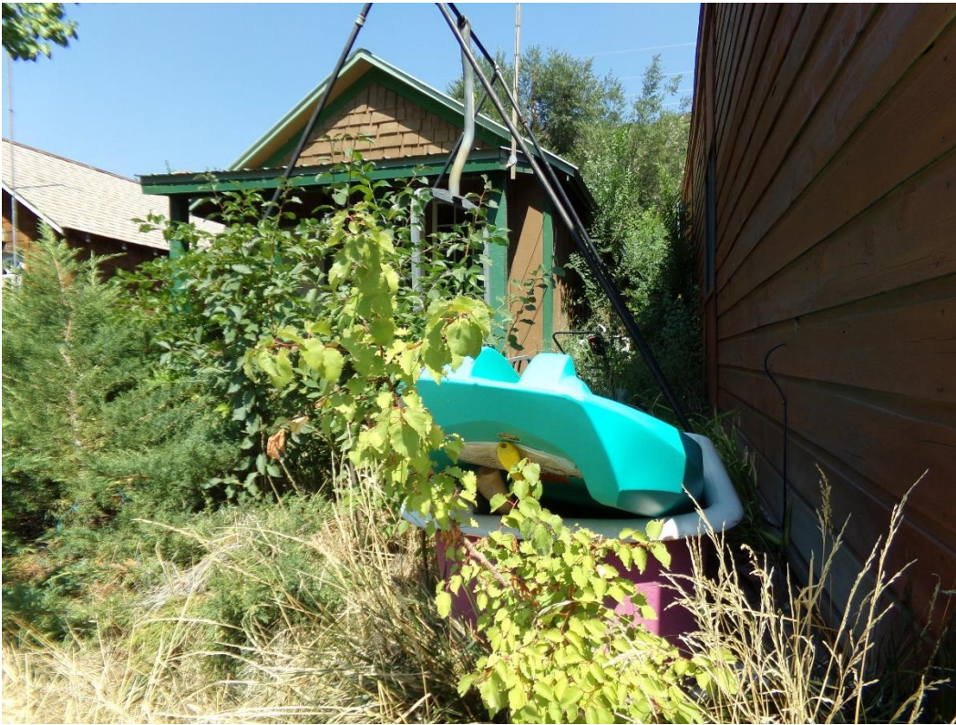
Photo Number: 5GF.5907_3 Description: Looking at the primary (south) and east elevations of the building. Date: 9/6/2022 View: Northwest
