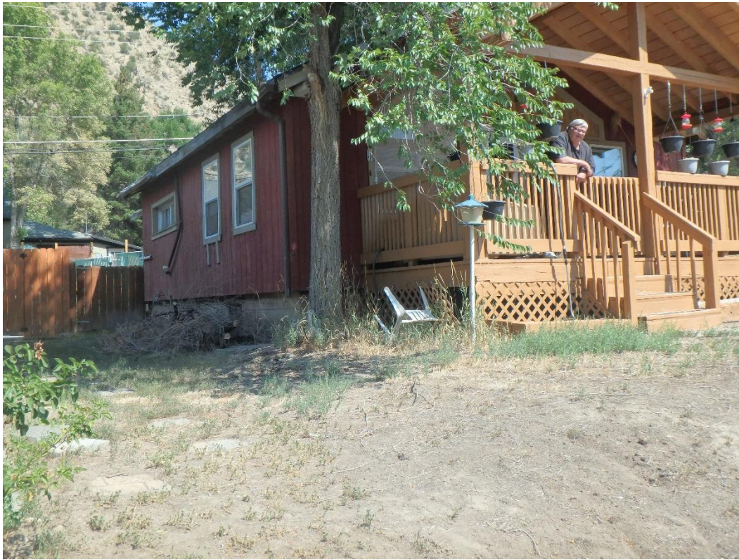
Photo Number: 5GF.5923_3 Description: Looking at the west and primary (south) elevations of the residence. Date: 9/6/2022 View: Northeast
