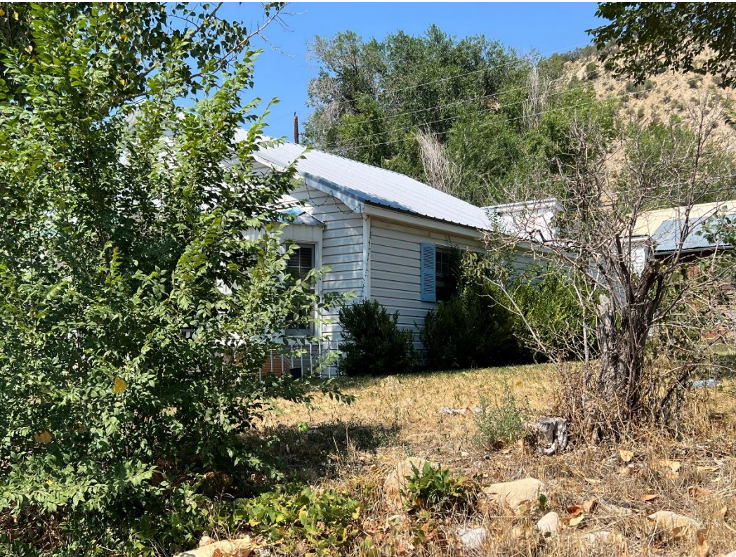
Photo Number: 5GF.5929_4 Description: Looking at the east elevation of the primary building. Date: 9/6/2022 View: Northwest
