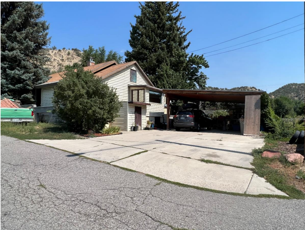
Photo Number: 5GF.5933_4 Description: Looking at the west elevation and south elevation of the building. Date: 9/6/2022 View: Northeast
