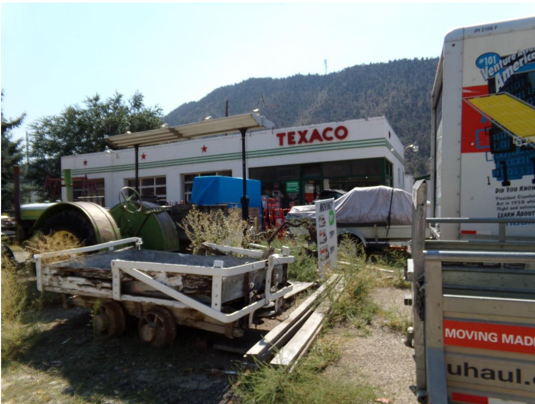
Photo Number: 5GF.5903_2 Description: Looking at the primary (north) and west elevations of the building. Note the fuel island in the foreground. Date: 9/6/2022 View: Southeast
