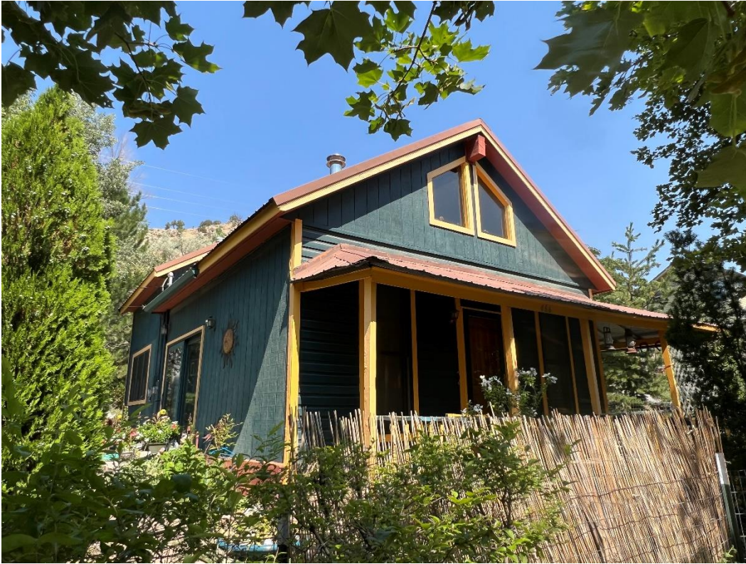
Photo Number: 5GF.5938_1 Description: Looking at the west and primary (south) elevation of the building. Date: 9/6/2022 View: Northeast
