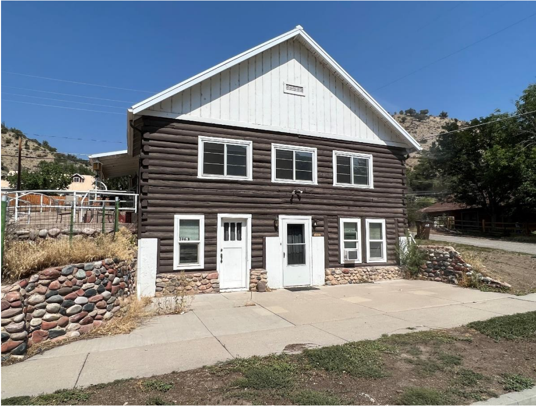
Photo Number: 5GF.5932_1 Description: Looking at the south elevation of the building. Date: 9/6/2022 View: Northeast
