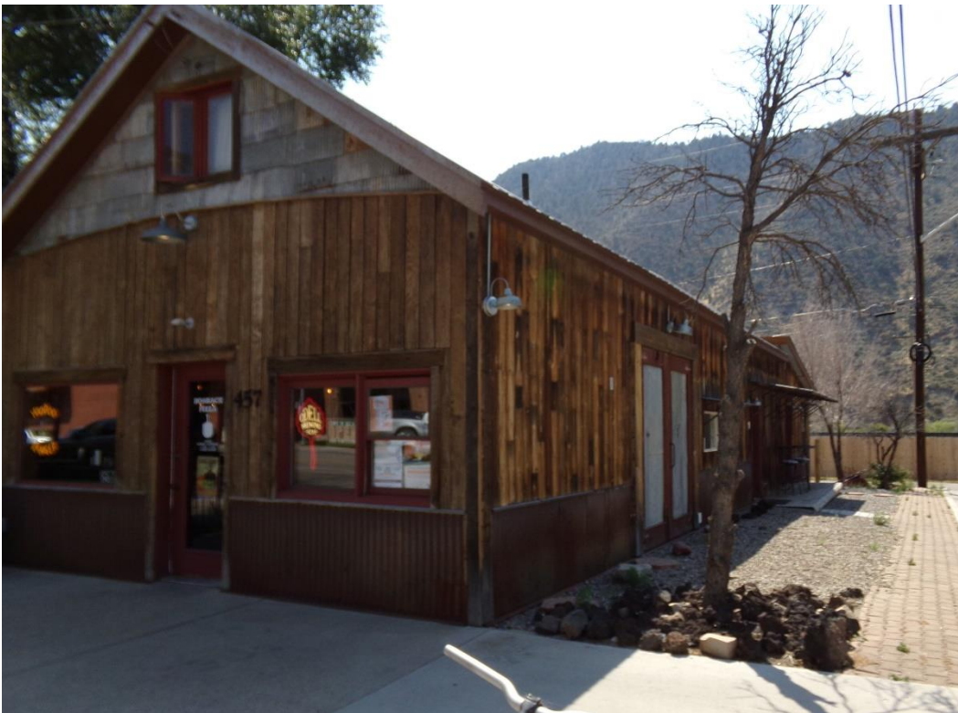
Photo Number: 5GF.5909_2 Description: Looking at the primary (north) and west elevations of the building. Date: 9/6/2022 View: Southeast
