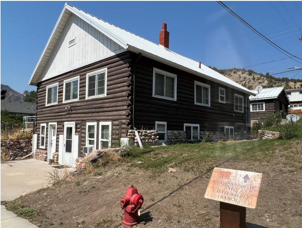
Photo Number: 5GF.5932_3 Description: Looking at the south and east elevations of the building. Date: 9/26/2022 View: Northwest
