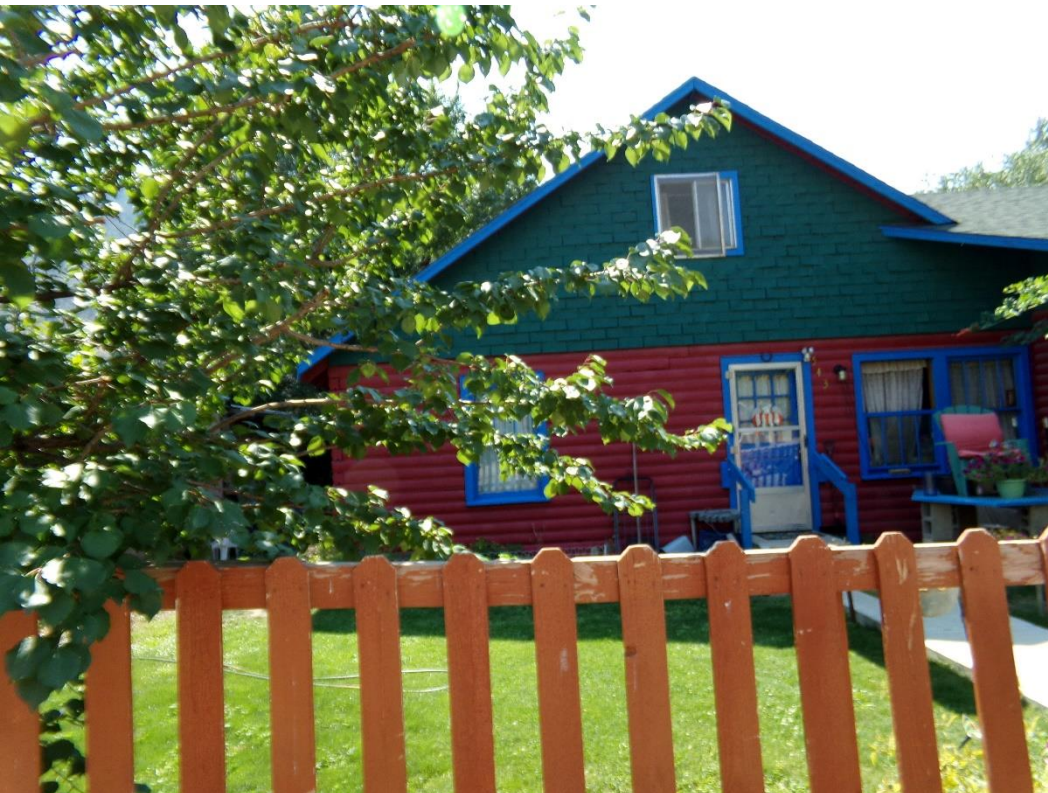
Photo Number: 5GF.5901_2 Description: Looking at the primary (north) elevation of the building Date: 9/6/2022 View: South
