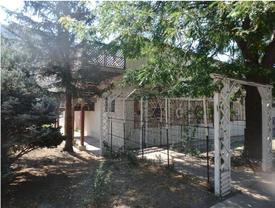
Photo Number: 5GF.2369_4 Description: Looking at the corner of the east elevation and the primary (north) elevation. Note the staircase leading to the second level addition to the building. Date: 9/6/2022 View: Southwest
