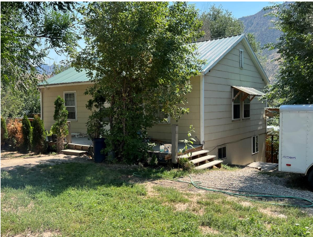
Photo Number: 5GF.5930_2 Description: Looking at the primary (north) and west elevations of the residence. Note the shed roof awning that protects the typical windows. Date: 9/6/2022 View: Southeast
