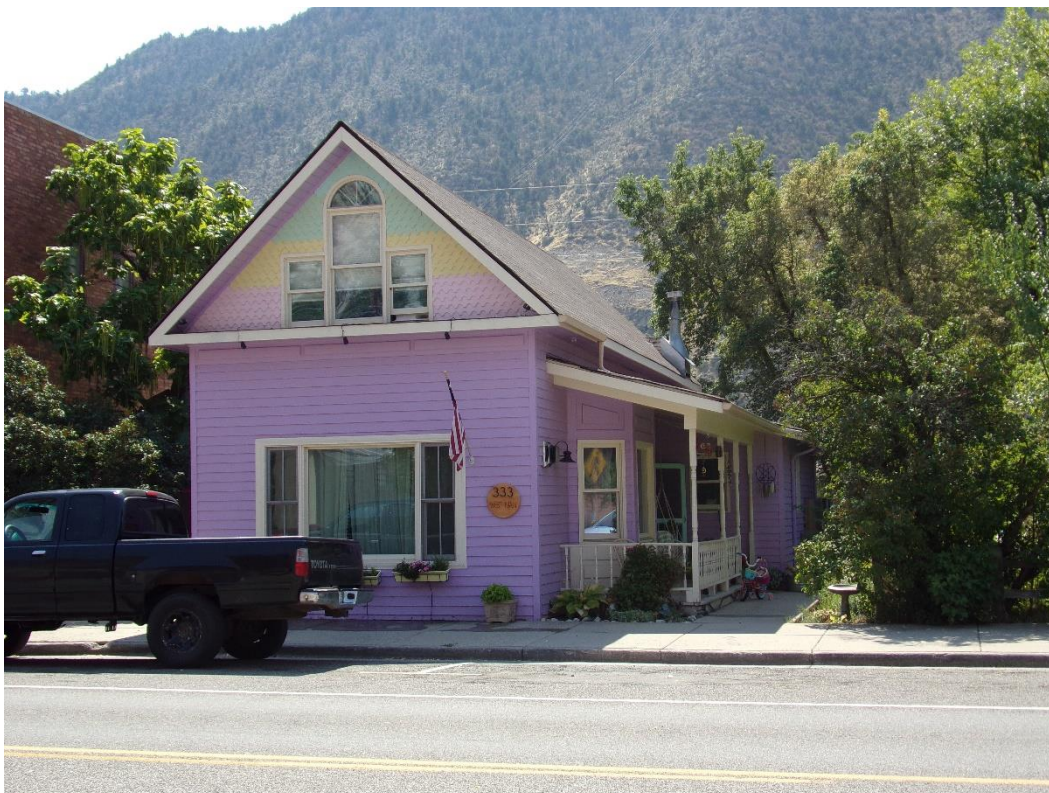
Photo Number: 5GF.5914_2 Description: Looking at the north and primary (west) elevations of the building. Date: 9/6/2022 View: Southeast
