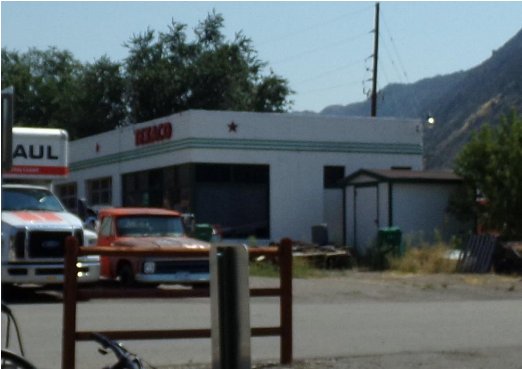
Photo Number: 5GF.5903_3 Description: Looking at the primary (north) elevation and west elevations of the building. Date: 9/6/2022 View: Southeast
