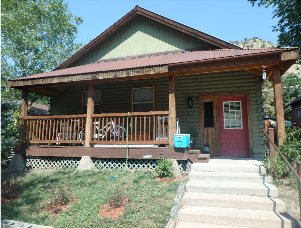
Photo Number: 5GF.5922_1 Description: Looking at the primary (south) elevation of the building. Date: 9/6/2022 View: North
