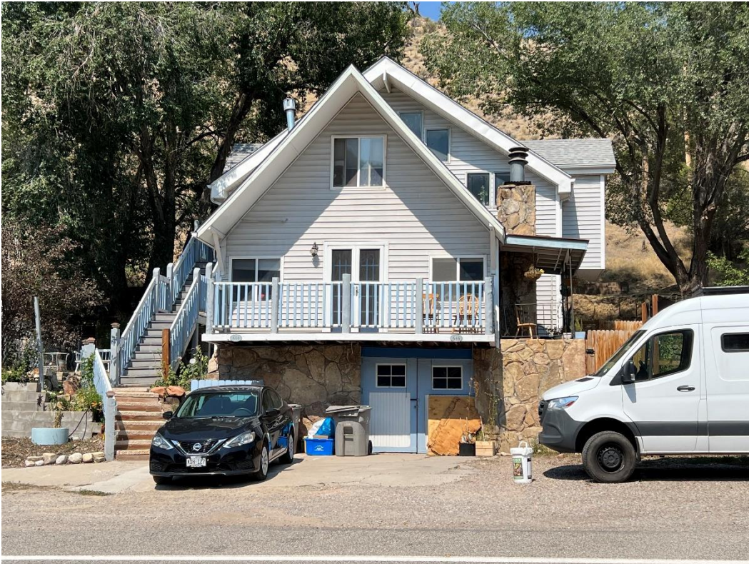
Photo Number: 5GF.5941_1 Description: Looking at the primary (south) elevation of the building. Note the front gable and the side gable projections below the front gable roofline. Date: 9/6/2022 View: North
