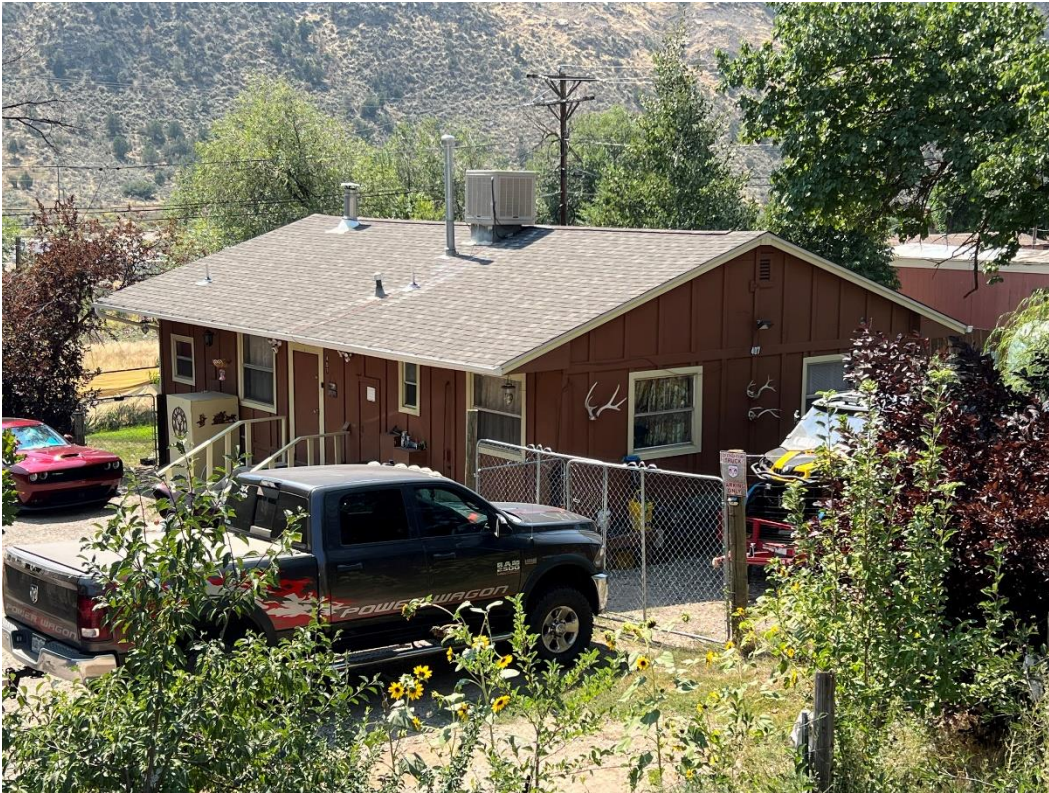
Photo Number: 5GF.5936_1 Description: Looking at the primary (east) elevation and north elevation of the building. Date: 9/6/2022 View: Southwest
