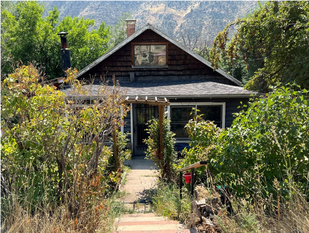
Photo Number: 5GF.5939_1 Description: Looking at the primary (north) elevation of the building. Note the wood shingles under the gable end. Date: 9/6/2022 View: South
