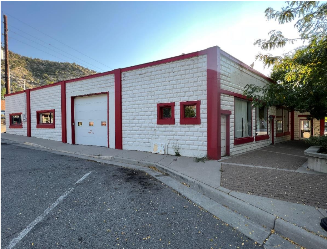
Photo Number: 5GF.2373_3 Description: Looking at the west and primary (south) elevation of the building. Date: 9/6/2022 View: Northeast
