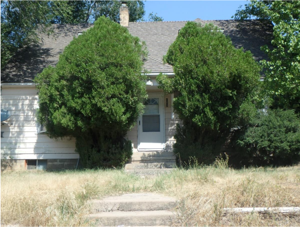
Photo Number: 5GF.5924_1 Description: Looking at the primary (south) elevation of the building. Note that the two recessed dormers are mostly obscured by the tall vegetation. Date: 9/6/2022 View: North
