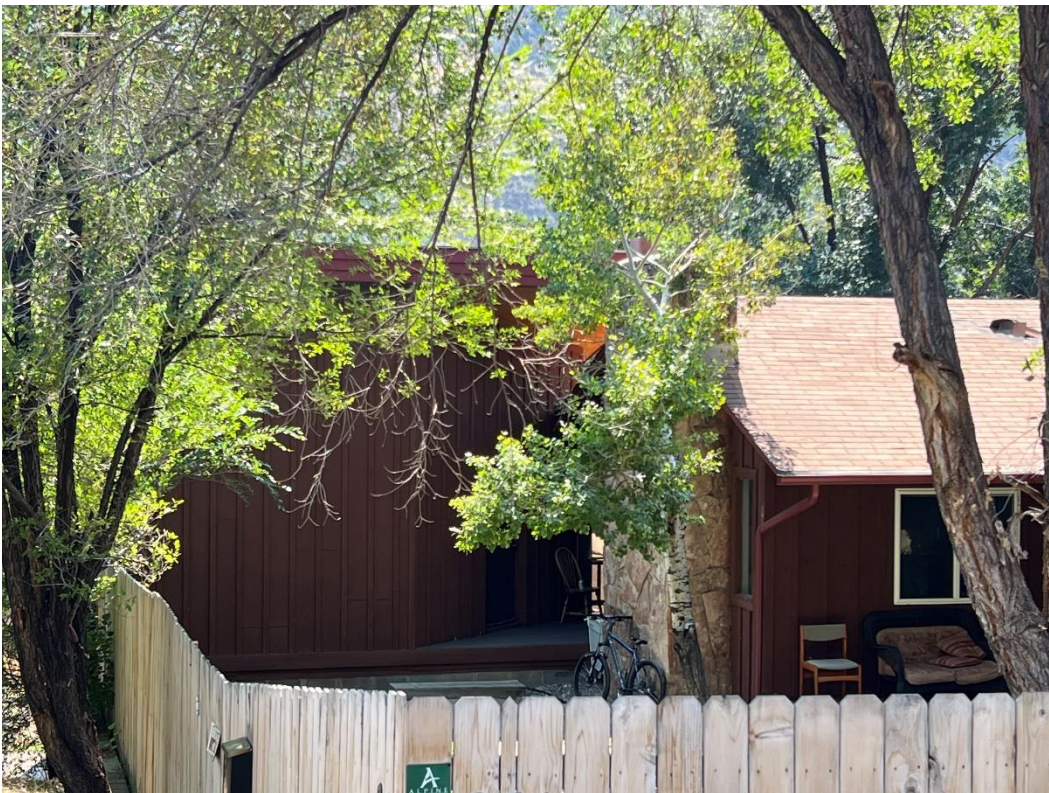
Photo Number: 5GF.5942_2 Description: Close up of the primary (east) elevation of the building. Note the stone masonry chimney. Date: 9/6/2022 View: Southwest
