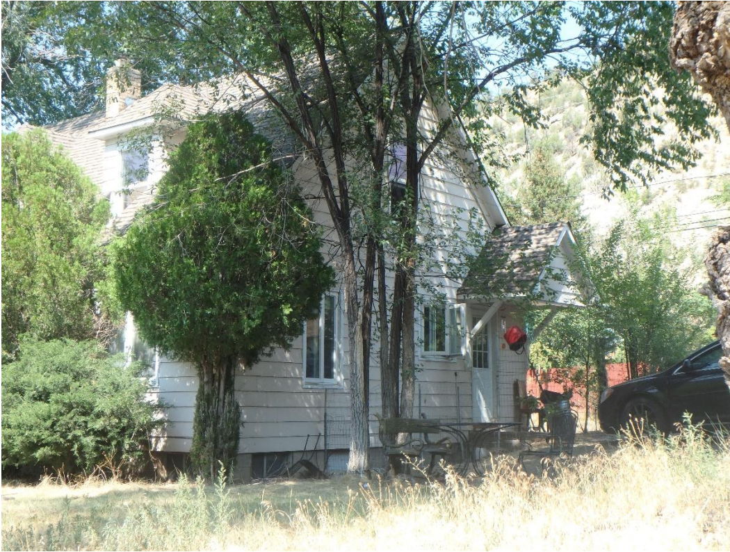
Photo Number: 5GF.5924_3 Description: Looking at the primary (south) and east elevations of the residence. Note the gable overhang that protects the secondary entryway. Date: 9//6/2022 View: Northwest
