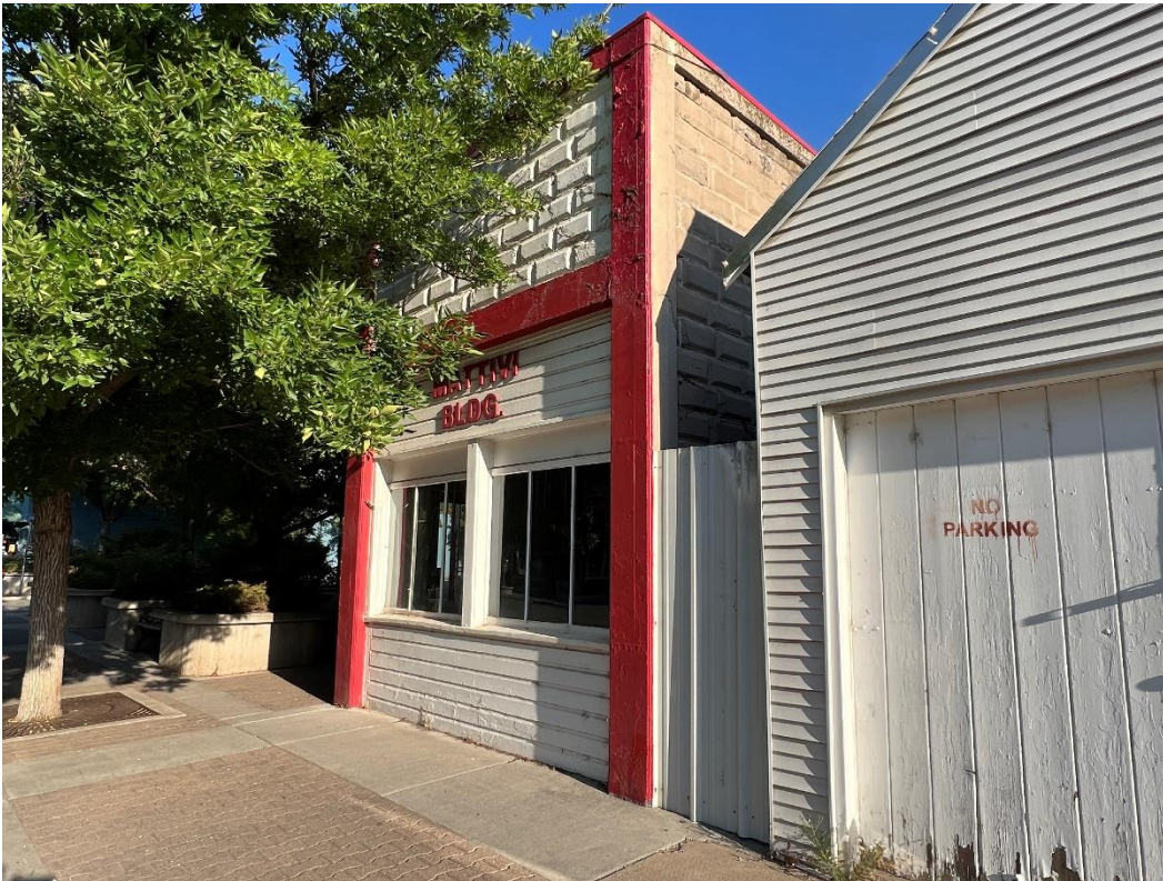
Photo Number: 5GF.2373_4 Description: Looking at the far-right side of the primary (south) and a portion of the east elevations. Note the former garage door opening that was covered by the mid to late Twentieth Century. Date: 9/6/2022 View: Northwest
