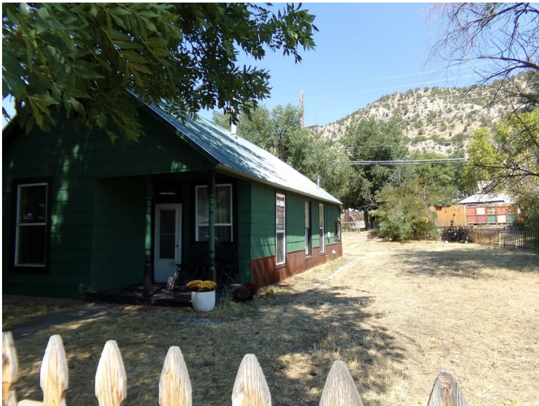
Photo Number: 5GF.5902_2 Description: Looking at the primary (south) and east elevations of the building. Date: 9/6/2022 View: Northwest
