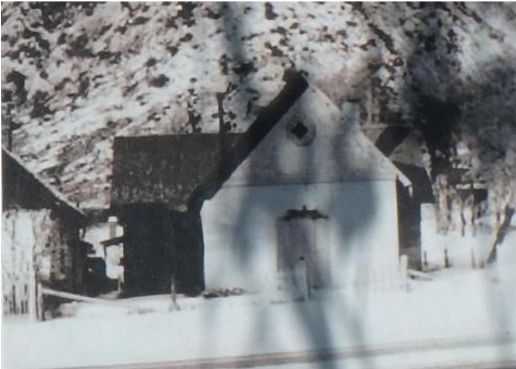
Historic Photo 1 Description: Looking at the primary (south) elevation of the church. Note that the front gable bay was not extant at the time, yet the oxeye, brick masonry chimney, and wood shingles in the gable end are extant. Date: Unknown; likely early-Twentieth Century Source: "New Castle Museum on the Street" sign along primary (south) elevation of the church
