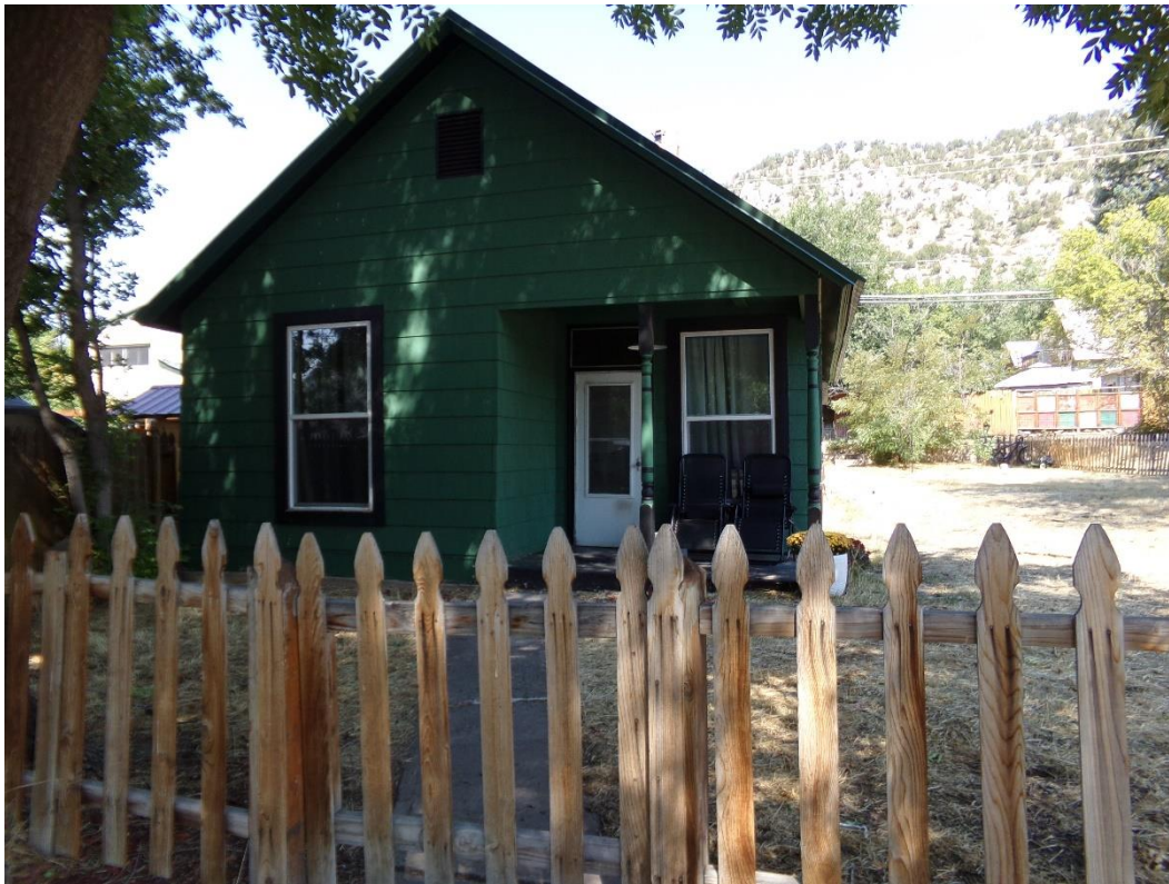
Photo Number: 5GF.5902_1 Description: Looking at the primary (south) elevation of the building. Date: 9/6/2022 View: North
