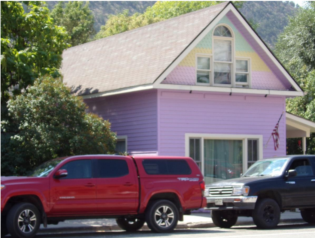
Photo Number: 5GF.5914_3 Description: Looking at the east and north elevation of the building. Date: 9/6/2022 View: Southwest
