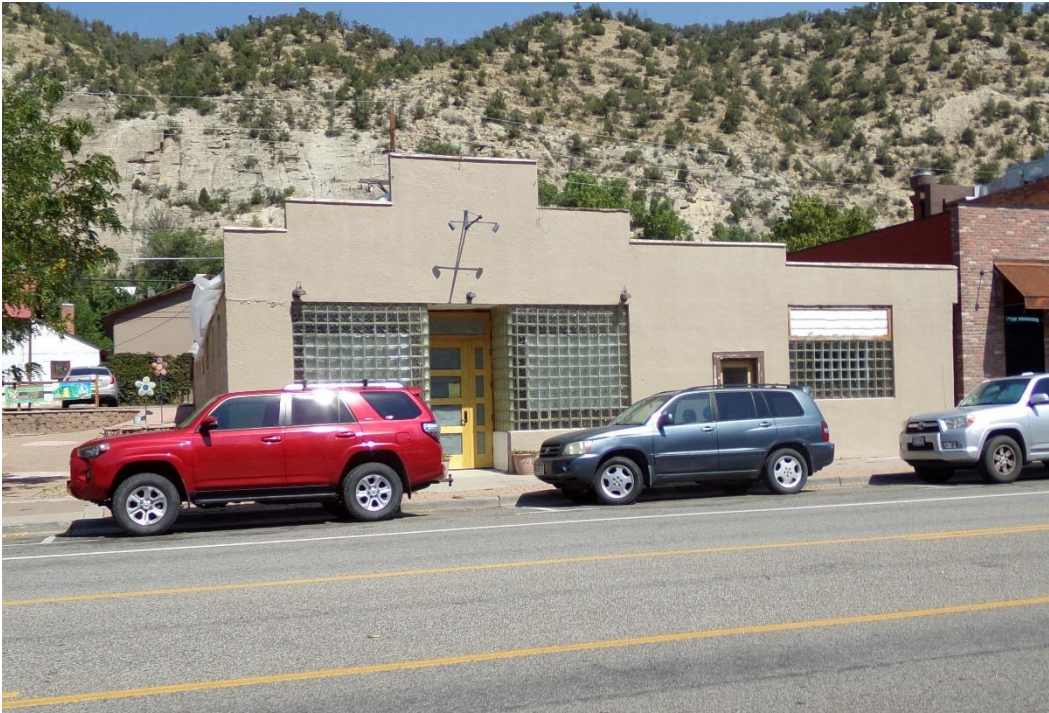
Photo Number: 5GF.5912_1 Description: Looking at the primary (south) elevation of the building. Date: 9/6/2022 View: North
