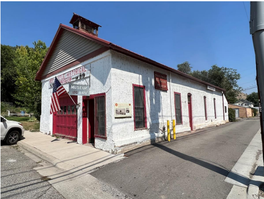
Photo Number: 5GF.1665_2 Description: Looking at the primary (west) and south elevations of the building. Date: 9/6/2022 View: Northeast
