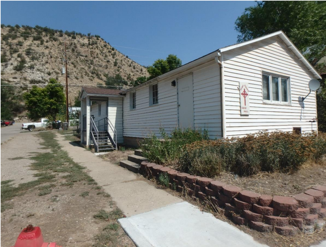
Photo Number: 5GF.5921_1 Description: Looking at the primary (west) and south elevations of the building. Date: 9/6/2022 View: Northeast
