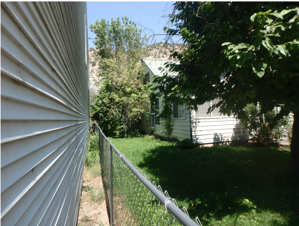
Photo Number: 5GF.5918_2 Description: Looking at the west and primary (south) elevation of the building. Note that the wall to the left is not a part of the residence. Date: 9/6/2022 View: Northeast
