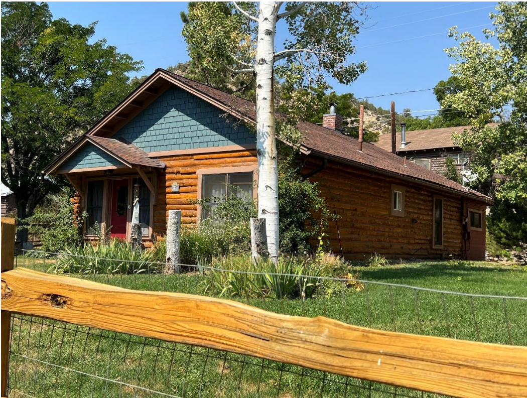
Photo Number: 5GF.5935_2 Description: Looking at the primary (south) and east elevations of the building. Date: 9/6/2022 View: Northwest
