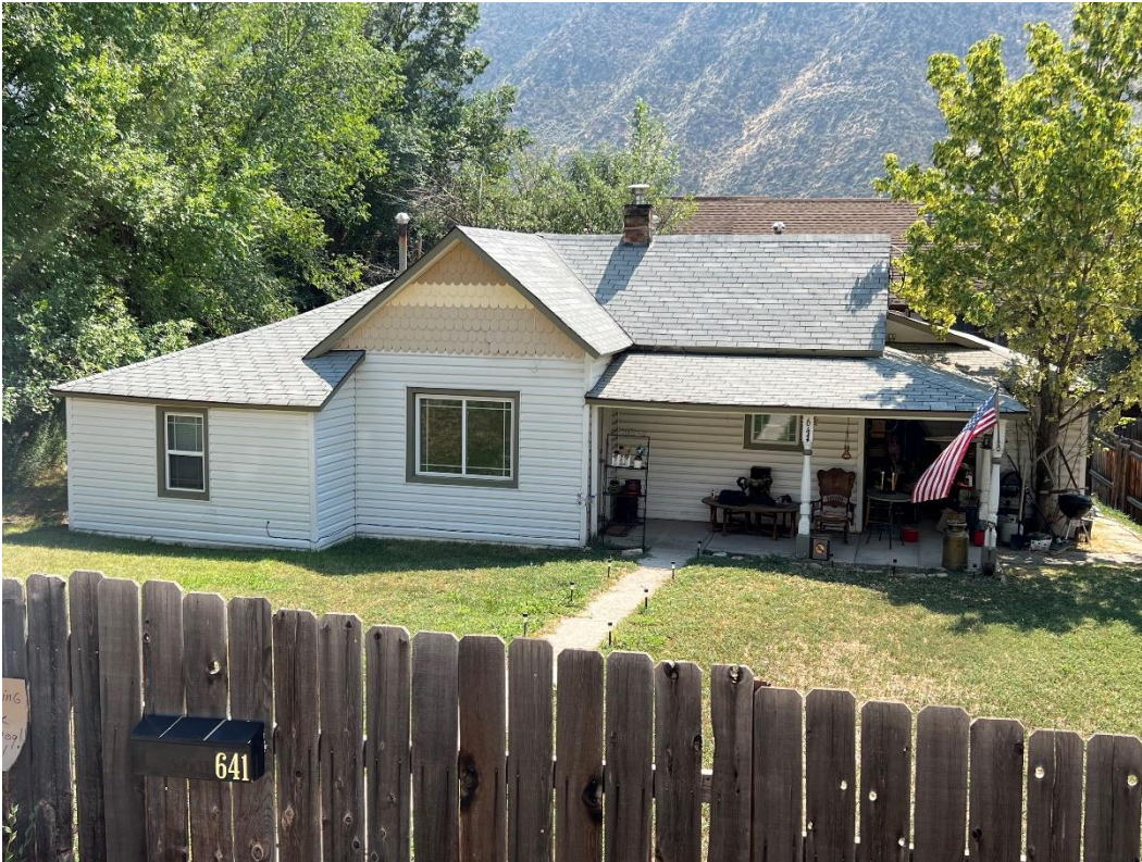
Photo Number: 5GF.5940_1 Description: Looking at the primary (north) elevation of the building. Date: 9/6/2022 View: Southeast
