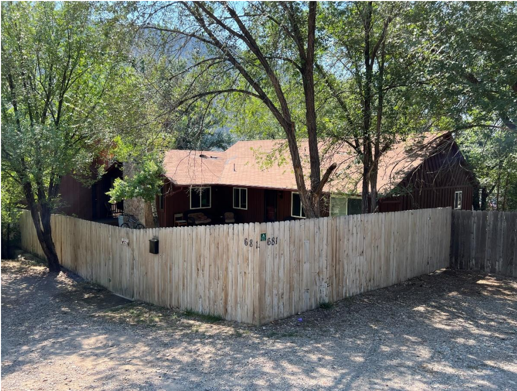
Photo Number: 5GF.5942_1 Description: Looking at the primary (east) and north elevations of the residence. Date: 9/6/2022 View: Southwest
