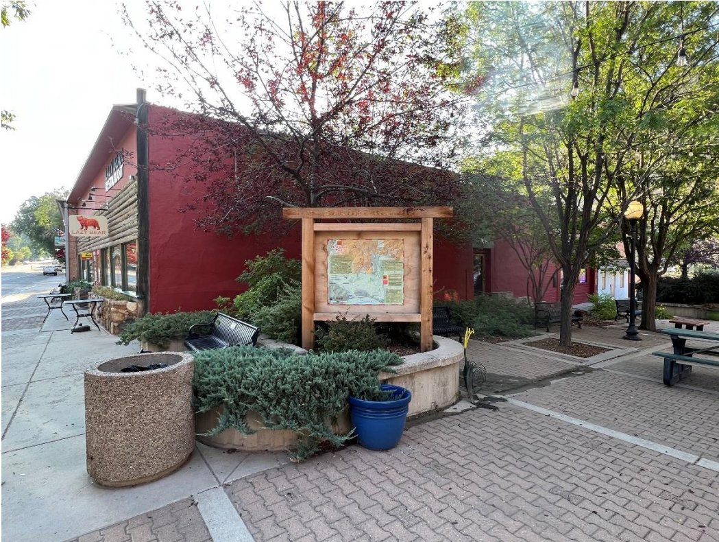
Photo Number: 5GF.2374_2 Description: Looking at the primary (north) and west elevations of the building. Date: 9/6/2022 View: Southeast
