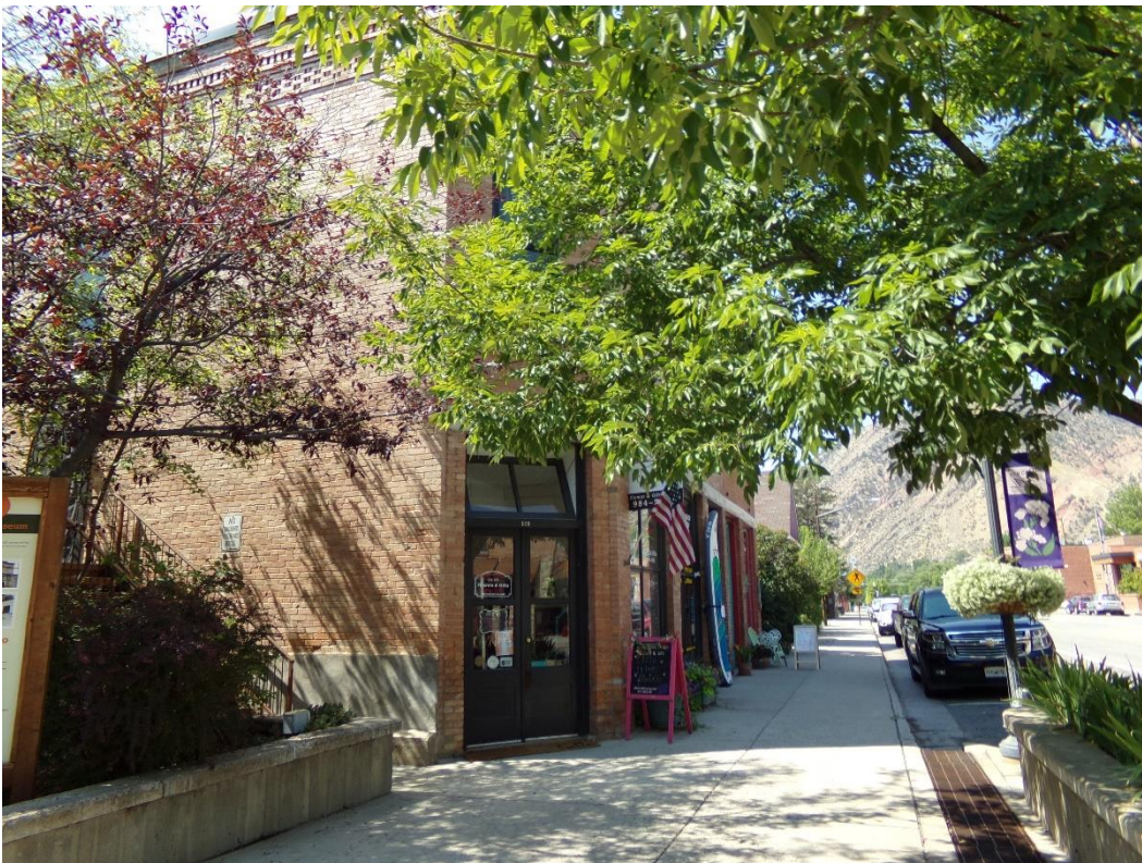
Photo Number: 5GF.2376_2 Description: Looking at the east and angled main entryway along the primary (north) elevation of the building. Date: 9/6/2022 View: West
