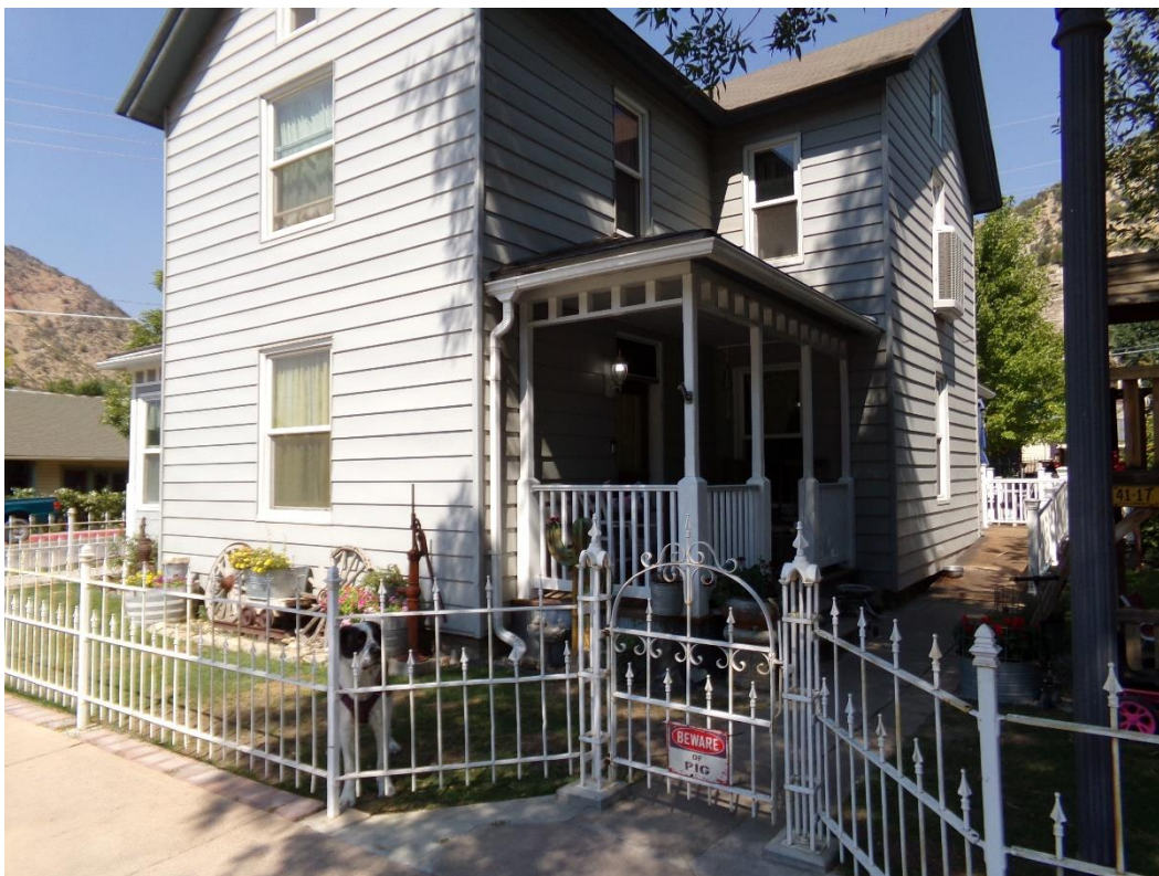
Photo Number: 5GF.5900_2 Description: Looking at the south and primary (east) elevations of the building. Date: 9/6/2022 View: Northwest
