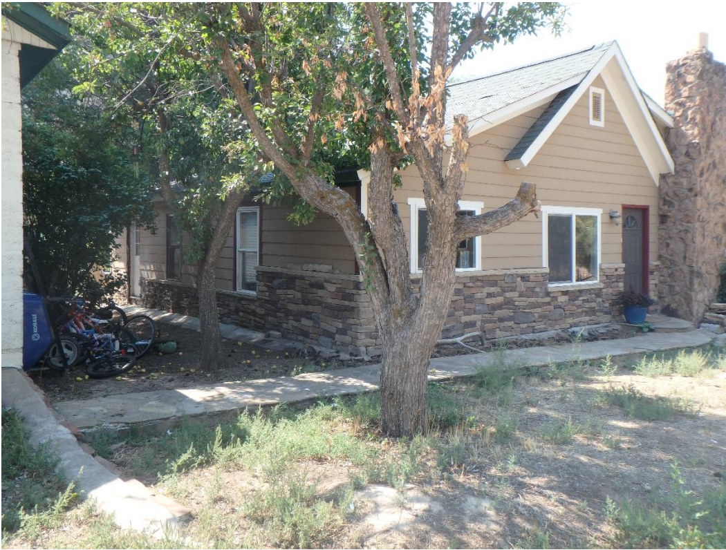
Photo Number: 5GF.5928_3 Description: Looking at the west and primary (north) elevations of the building. Date: 9/6/2022 View: Southwest
