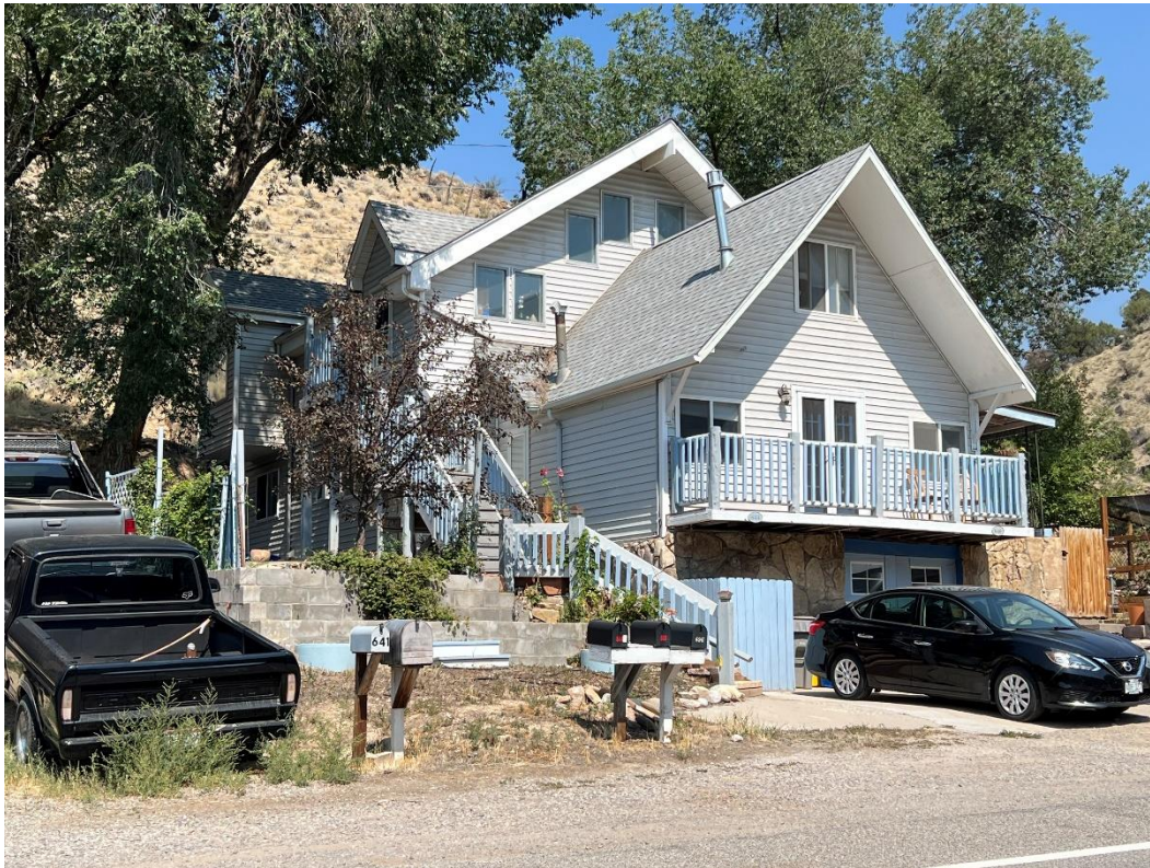
Photo Number: 5GF.5941_3 Description: Looking at the west and primary (south) elevations of the building. Note the staircase leads from the basement level to the second floor. Date: 9/6/2022 View: Northeast
