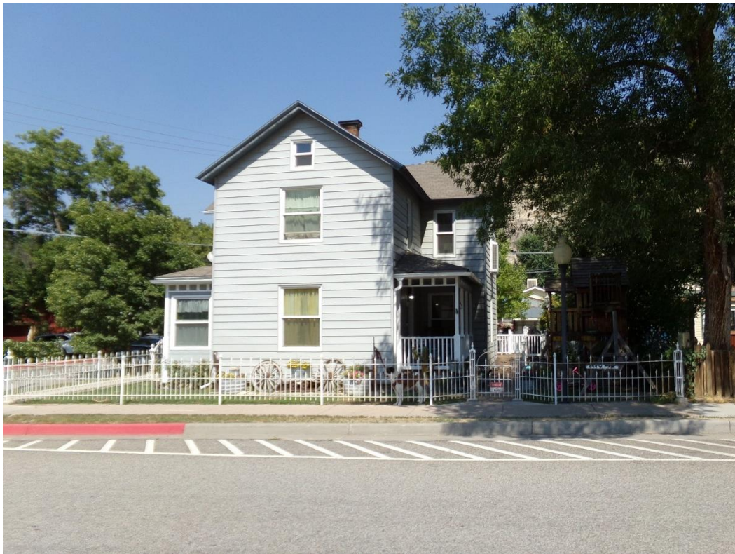
Photo Number: 5GF.5900_1 Description: Looking at the south and primary (east) elevations of the building. Note the decorative wrought iron fence in front of the residence. Date: 9/6/2022 View: Northwest
