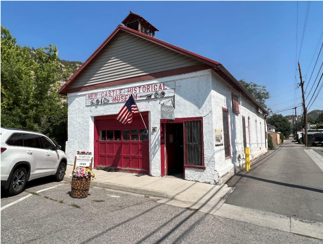
Photo Number: 5GF.1665_1 Description: Looking at the primary (west) and south elevations of the building. Date: 9/6/2022 View: Northeast
