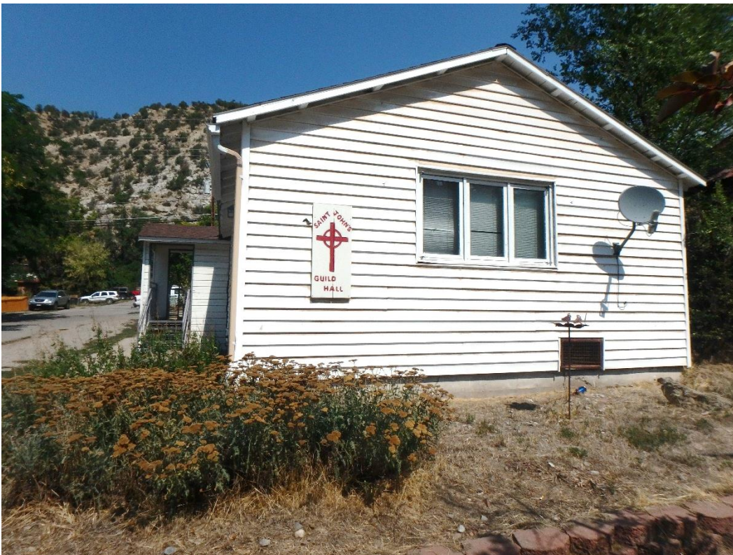
Photo Number: 5GF.5921_2 Description: Looking at the south elevation of the building. Date: 9/6/2022 View: North
