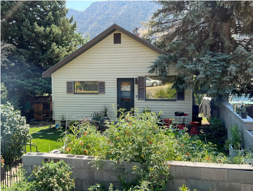
Photo Number: 5GF.5933_1 Description: Looking at the primary (north) elevation of the building. Date: 9/22/2022 View: South
