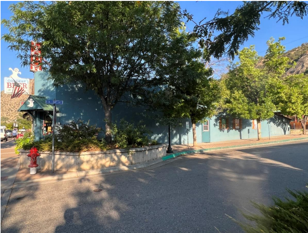
Photo Number: 5GF.2375_3 Description: Looking at the east elevation of the building. Note that a majority of the elevation is observed by landscaping features added between 1996 and 2005. Date: 9/6/2022 View: Northwest
