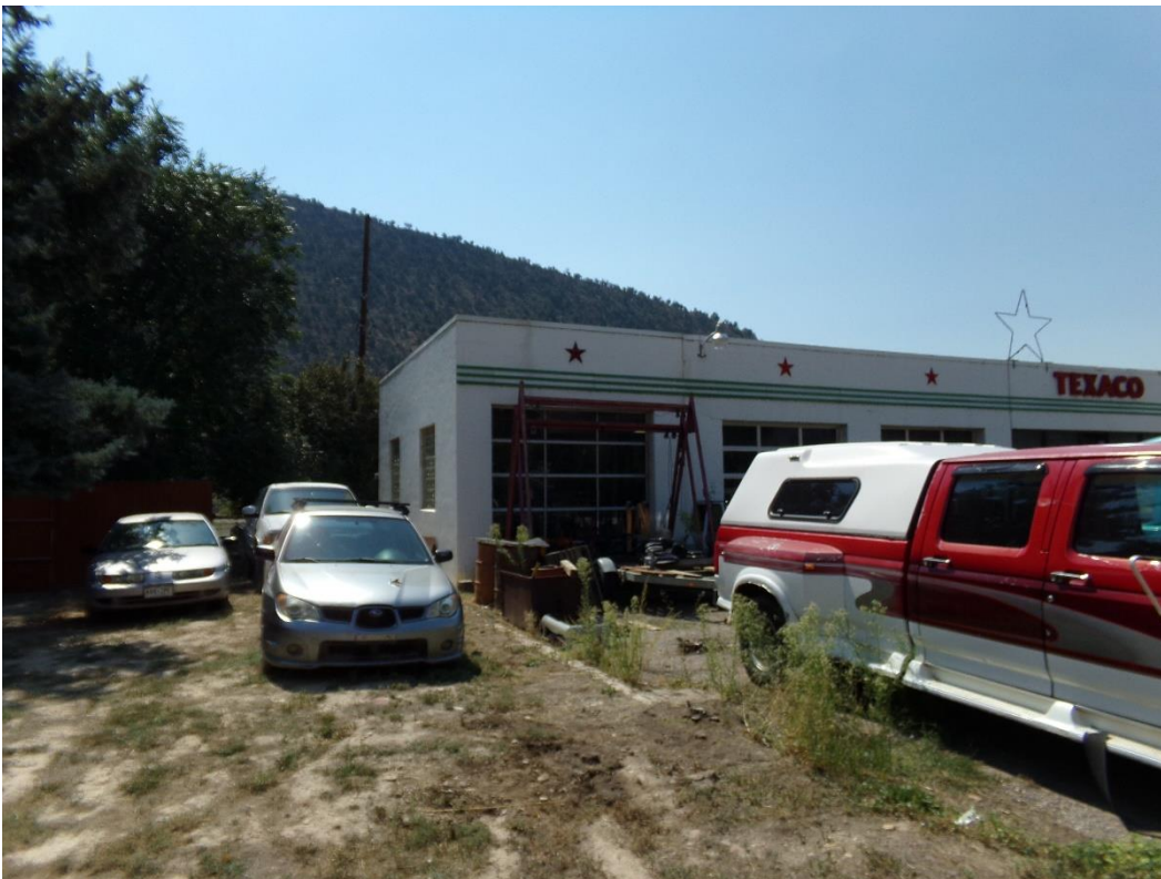
Photo Number: 5GF.5903_4 Description: Looking at the east and primary (north) elevations of the building. The third bay on the far left is likely an addition. Date: 9/6/2022 View: Southwest
