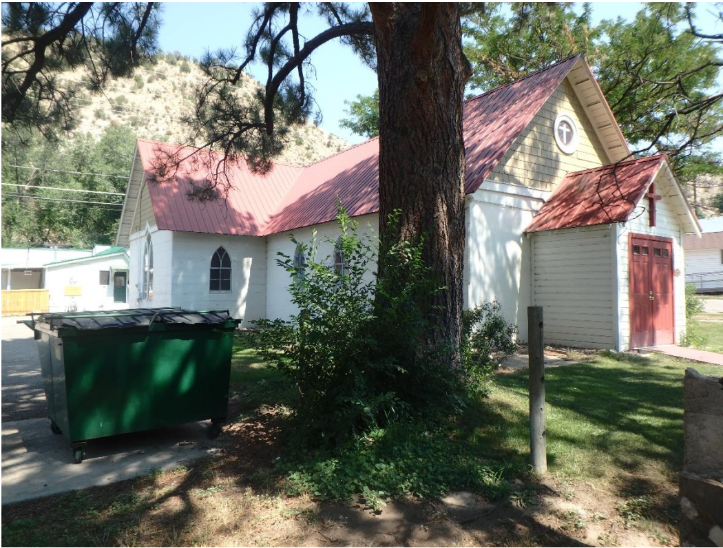
Photo Number: 5GF.2368_3 Description: Looking at the west elevation and primary (west) elevation of the building. Date: 9/6/2022 View: Northeast
