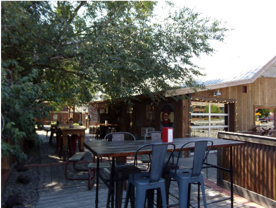
Photo Number: 5GF.5909_3 Description: Looking at the east and primary (north) elevations of the building. Date: 9/6/2022 View: Southwest
