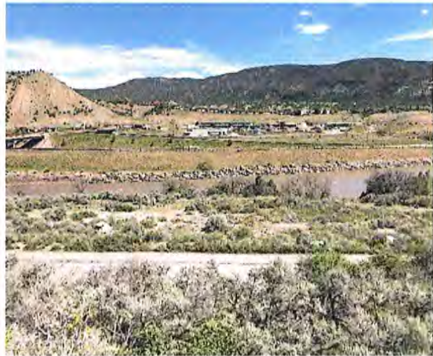
Rockfall Boulders on Subject Parcel
