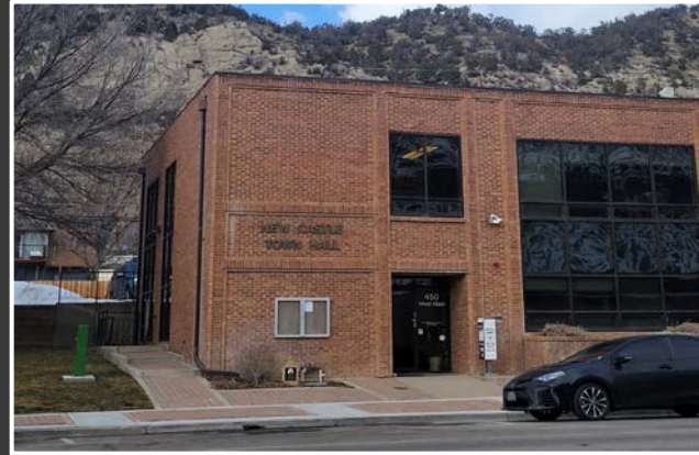
Town Hall Roof
