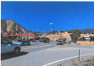
10. View to the North at existing intersection.
