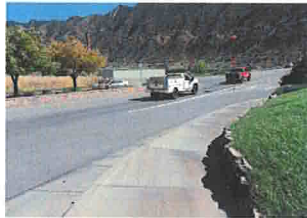
2. View of the intersection facing South.
