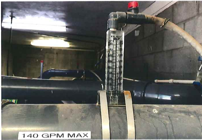
Image 57: Flow Meter for Slide
