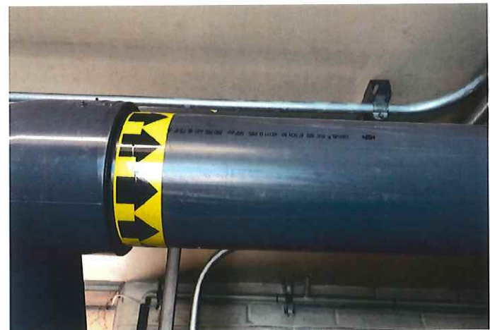
Image 12: Example of Circulation Pipe Labeling
