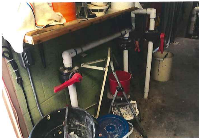
Image 29: Automatic Fill System Piping
