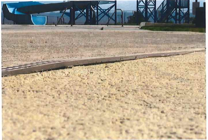
Image 28: Drain Grating Lifting in Deck
