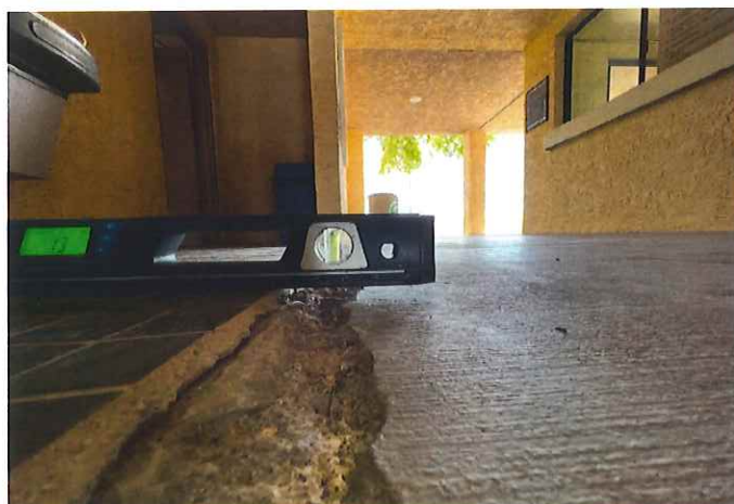
Image 43: Spalled Concrete Near Drinking Fountain
