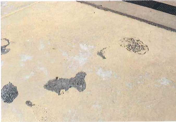
Image 27: Missing Deck Coating Around Swimming Pool
