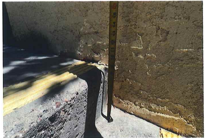
Image 34: Risers Exceed Maximum Code Allowable Height
