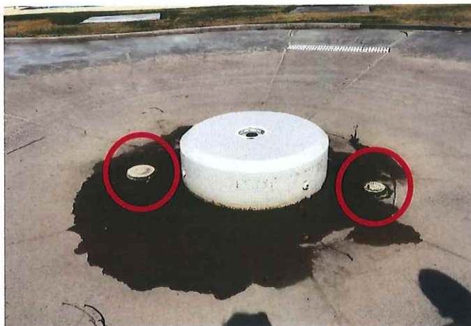
Image 11: Main Drains in Wading Pool
