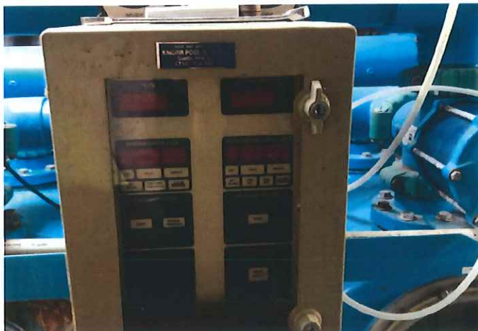
Image 55: Swimming Pool Filter Controller
