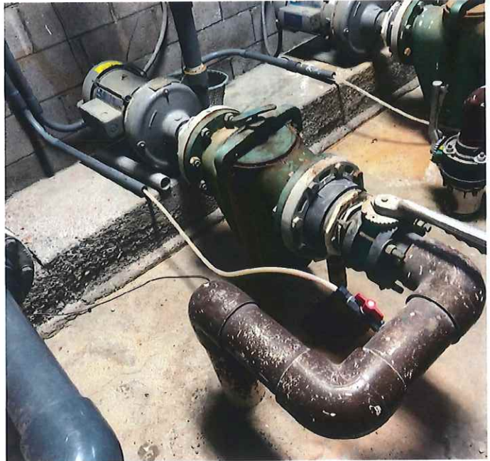
Image 3: Wading Pool Suction Piping, Pump and Motor
