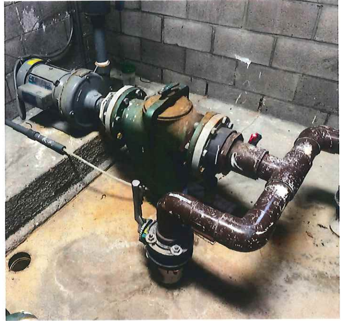
Image 4: Slide Pool Suction Piping, Pump and Motor
