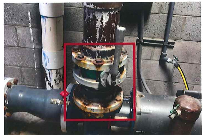
Image 56: Corroding Valves and Bolts for Slide Feature Pump
