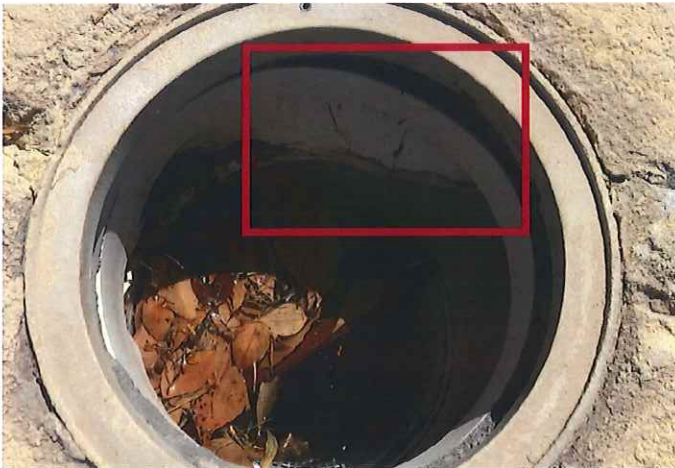
Image 65: Cracked Skimmer Box for Swimming Pool
