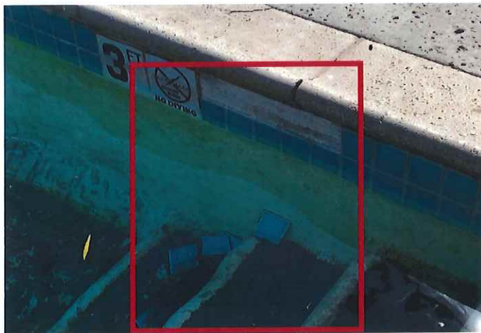
Image 17: Popped Off Tiles in Slide Receiving Pool
