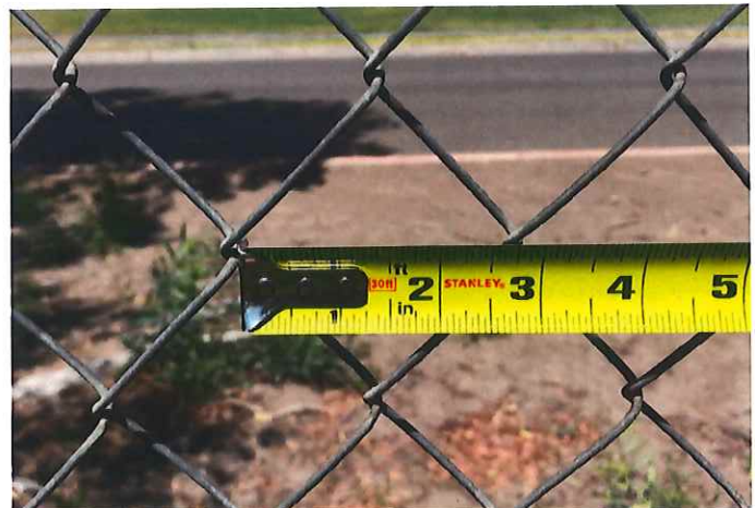
Image 24: Chain Link Fence Opening
