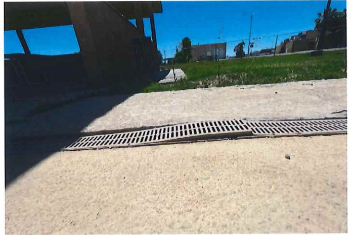
Image 46: Lifting Drains in Concrete Deck
