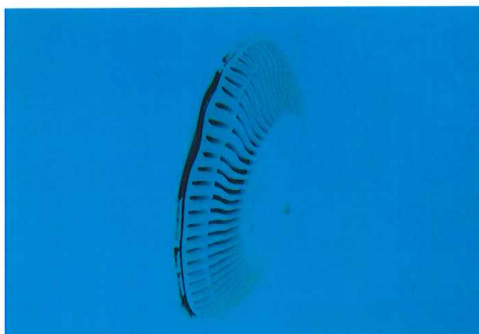
Image 19: Single Equalizer Suction Outlet in Swimming Pool
