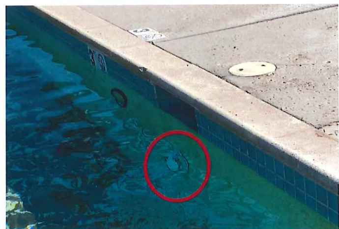
Image 20: Single Equalizer Suction Outlet in Swimming Pool
