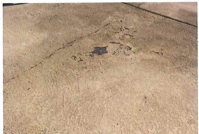
Image 26: Missing Deck Coating Around Swimming Pool
