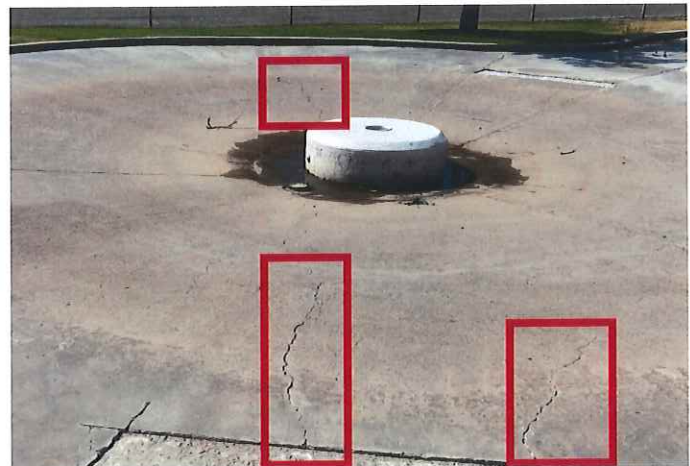
Image 18: Cracks in Wading Pool Concrete
