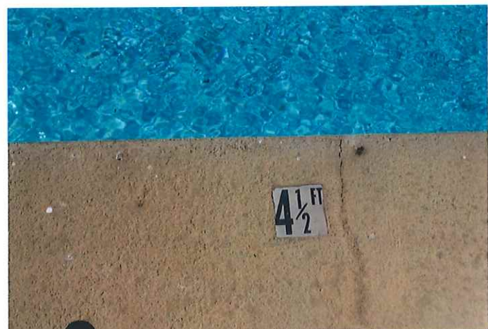
Image 14: Depth Marker with Fraction for Swimming Pool
