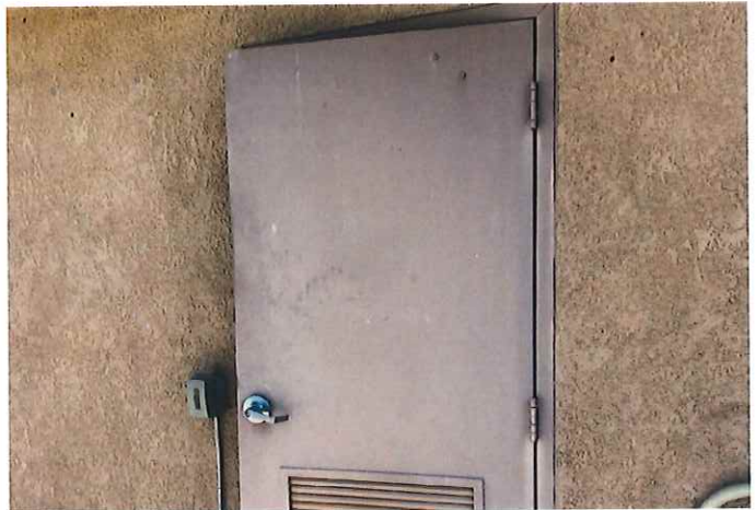
Image 22: Chlorine Room Door Missing NFPA Signage
