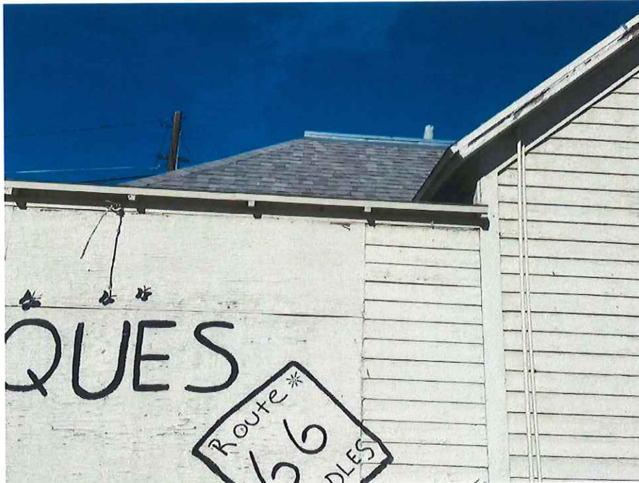
Photograph 9: Close-up of the rear east elevation illustrating the use of plywood to enclose a former open porch.
