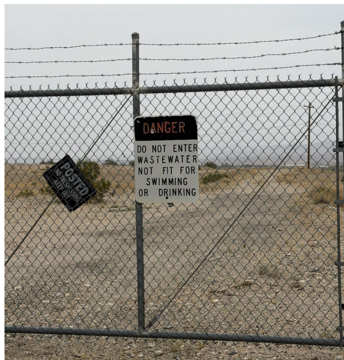
Figure 18. Evaporation/percolation pond area properly fenced and proper signage observed.
