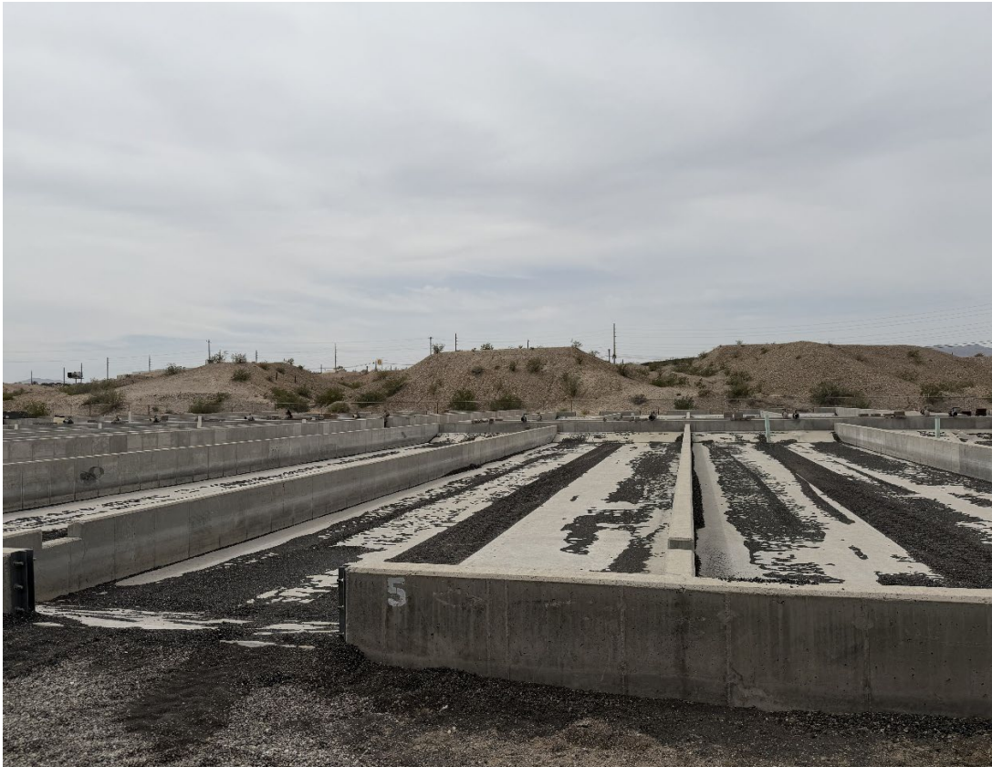
Figure 16. Sludge drying beds. There are a total of twenty-four sludge drying beds onsite.
