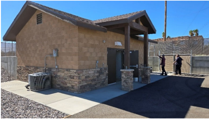
New Booster Station
