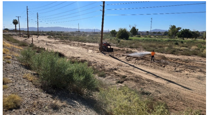
Phase 4B: Pipe Replacement – Under Construction
