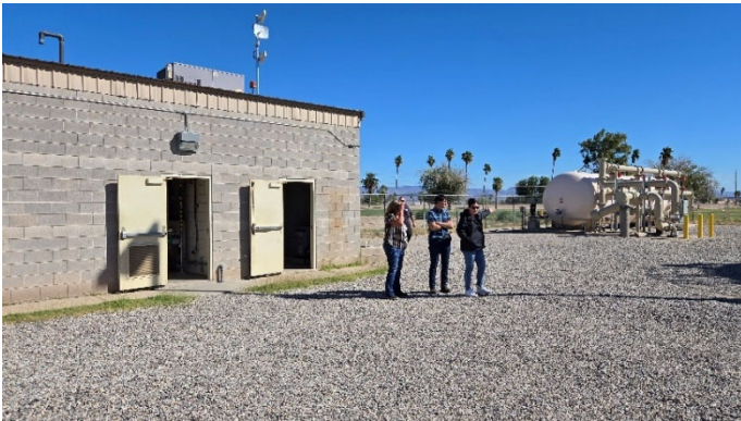
New Facility (filter shown in the background)
