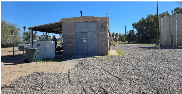
New Treatment Facility
