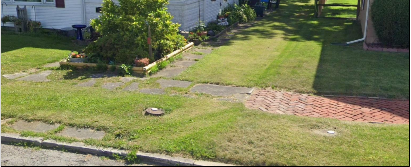
IMAGE: A sidewalk on North Third Street. The street has a sidewalk with partially complete segments, narrow width, and brick pavers.
