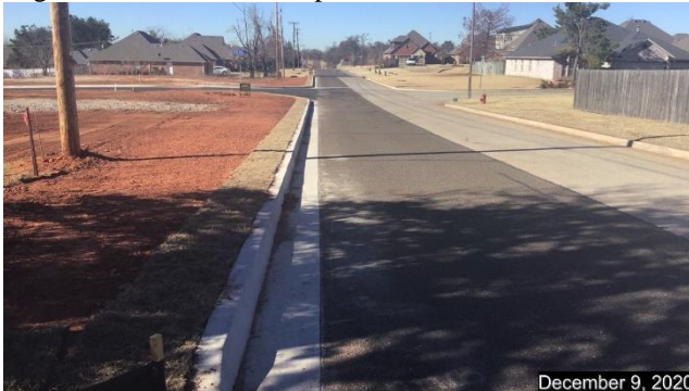
Looking west along S.E. 10 th Street
