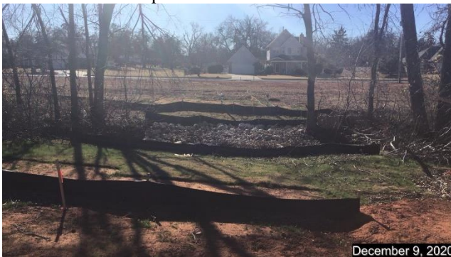
Area where sewer crossed undeveloped natural drainage
