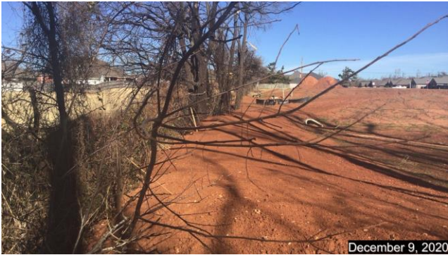
Looking north along west boundary of detention pond
