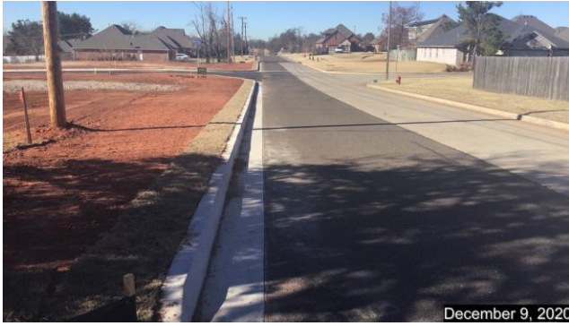
Looking west along S.E. 10 th Street
