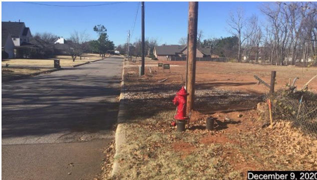
Looking west along S.E. 12 th Street, fire hydrant in foreground was installed by developer.
