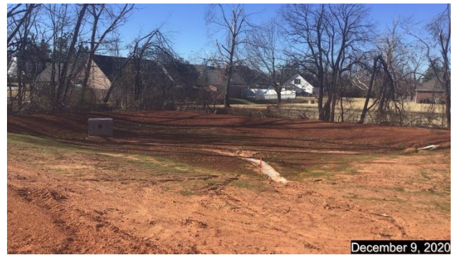
Detention pond of Ryans Ridge with paved trickle channel and weir outflow structure
