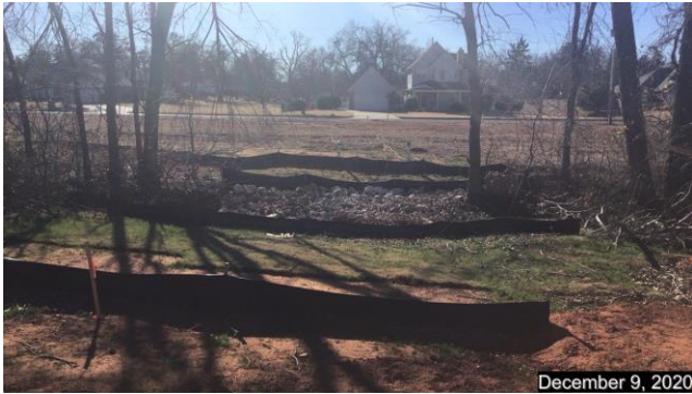
Area where sewer crossed undeveloped natural drainage
