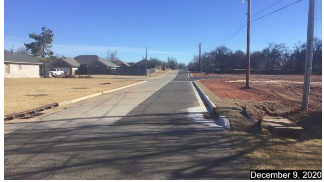
Looking east along S.E. 10 th Street
