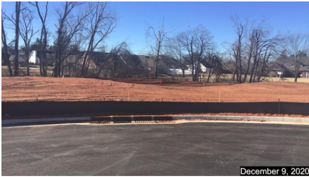
Cul-de-sac of Ryan Ridge Court, looking at inlet which flow into detention pond
