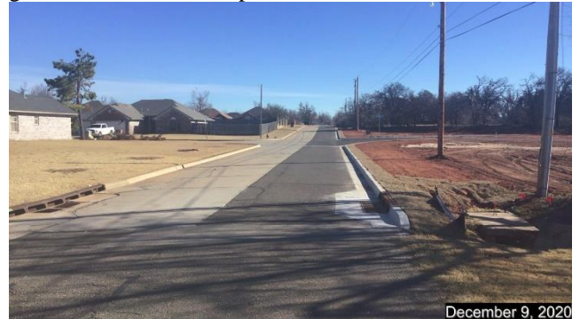
Looking east along S.E. 10 th Street
