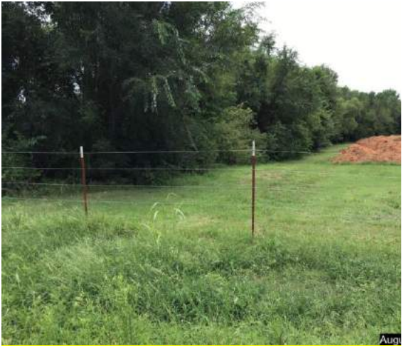
Water flows from the 24" cross drain across this property to the south to intersect with the drainage along the south.
