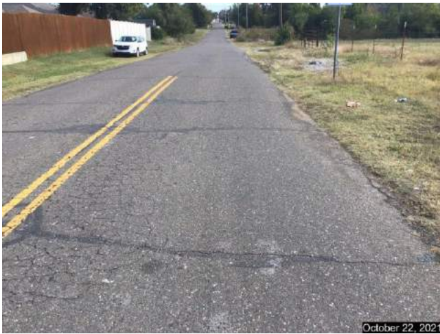
Looking east on SE 10 th Street. No Curb and Gutter or sidewalk. Note the poor condition of roadway surface.
