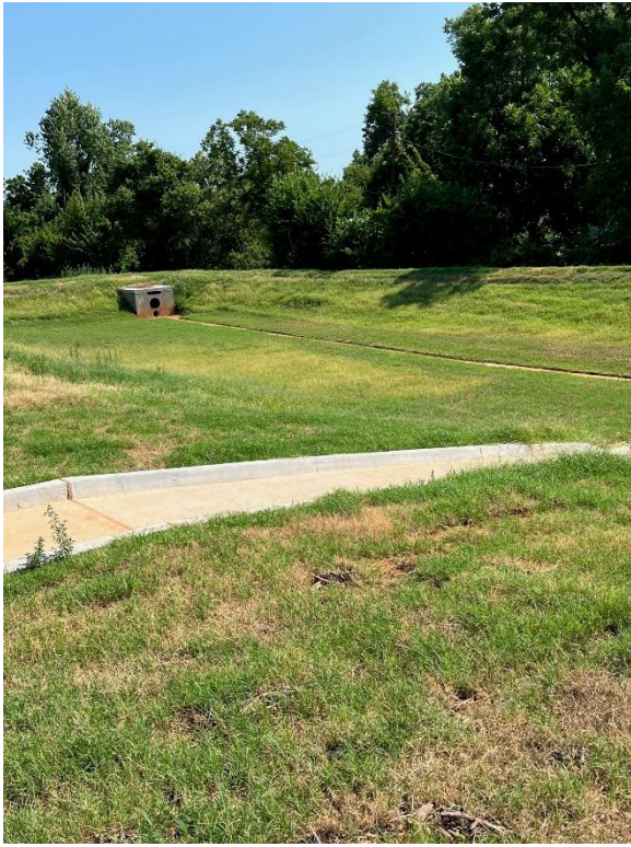
Detention Pond Improvements
