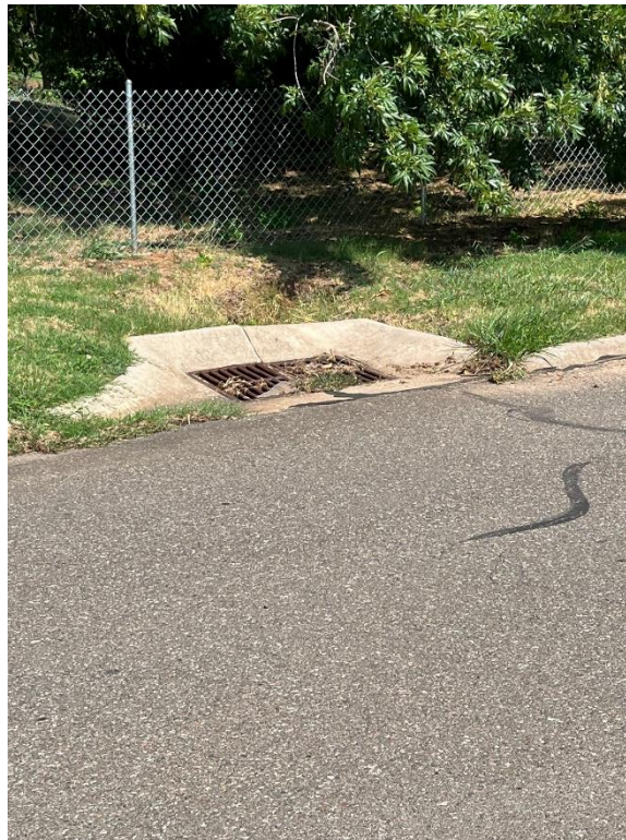
Drainage structure the detention will tie to.
