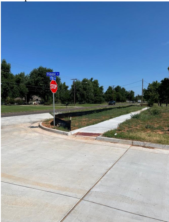
Improvements along Post Road
