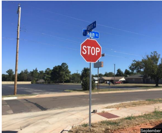
Sign at Main Street and Spirit Drive complete
