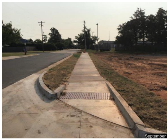
Looking east from the intersection of Spirit Drive and Main Street.
