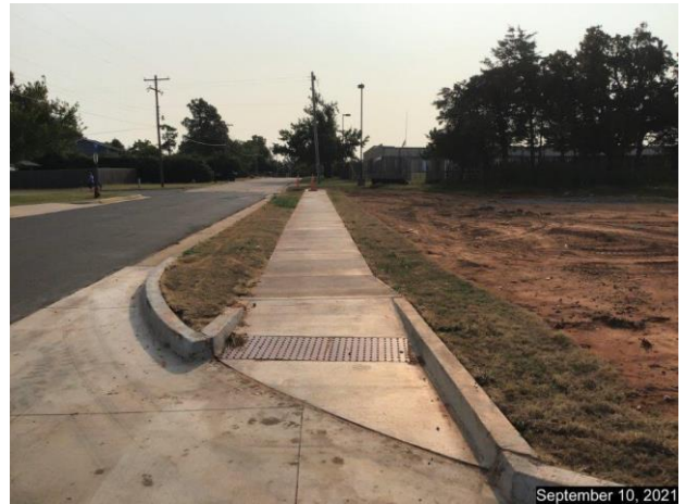
Looking east from the intersection of Spirit Drive and Main Street.
