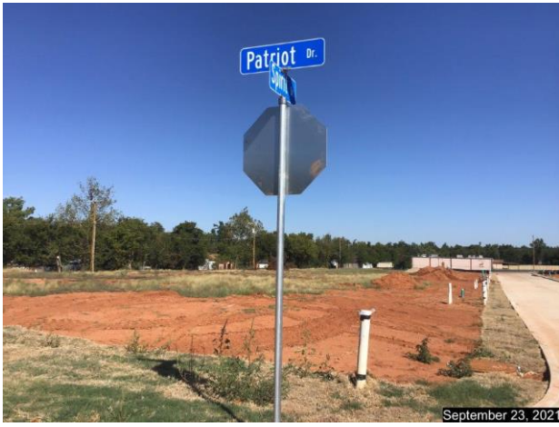
Sign at Patriot Drive and Spirit Drive complete
