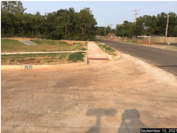
Looking west from the intersection of Spirit Drive and Main Street. Detention pond in view.
