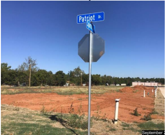
Sign at Patriot Drive and Spirit Drive complete
