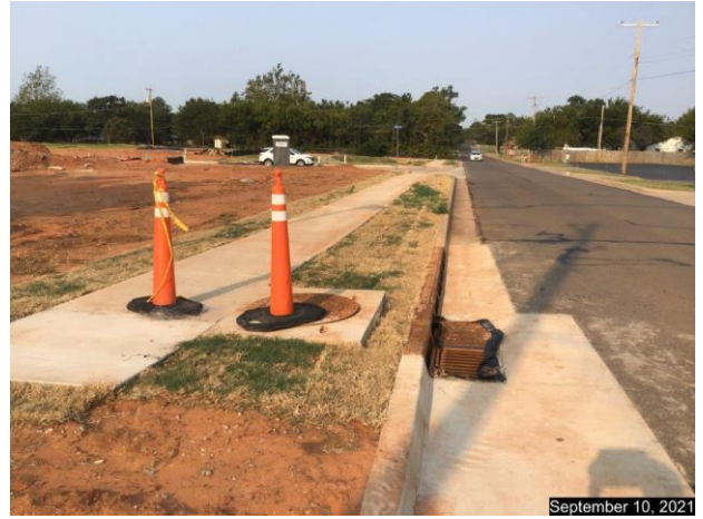
Looking west along Main Street from the NE corner of the development
