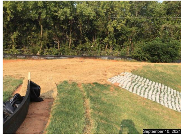
View of detention pond looking west. The area will accept sheet flow from 2 lots only with the concrete flex mat serving as scour protection.
