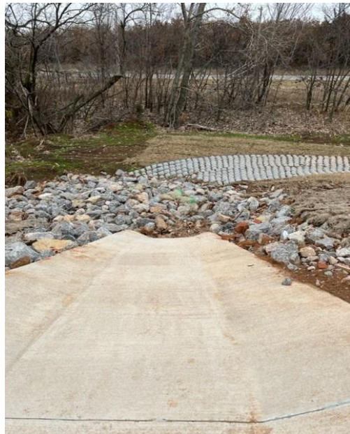
Southeast detention pond outflow
