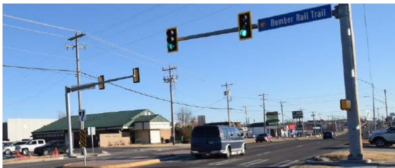
Figure 6 - Future Bomber Rail Trail Crossing Near the 700 Block of S Air Depot Blvd.
