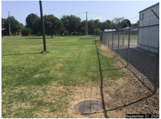
At the west property line looking east along the existing Sanitary Sewer which bisects the site
