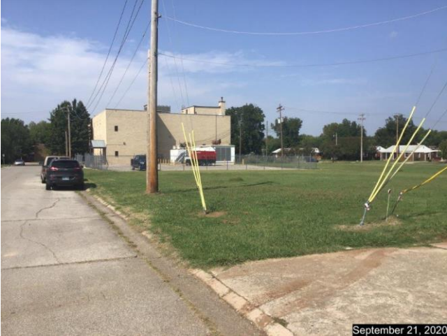
At SE corner looking NW
