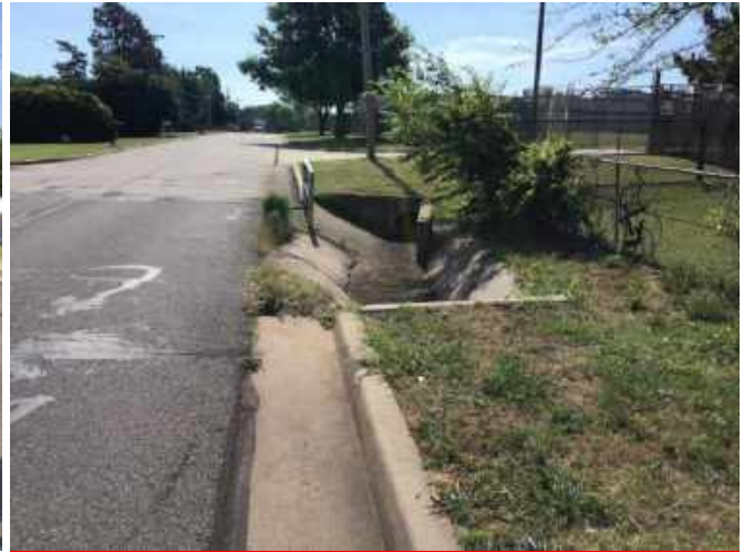
Looking east on E Main Street. Open paved ditch / inlet at Northeast corner.
