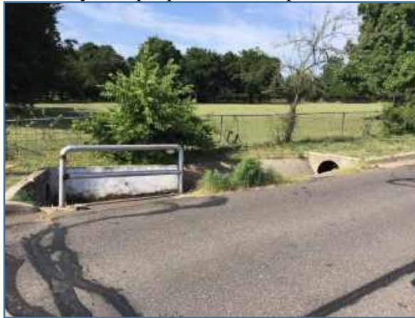
Open ditch / inlet to be improved with development. Entirely enclosed with new inlet
