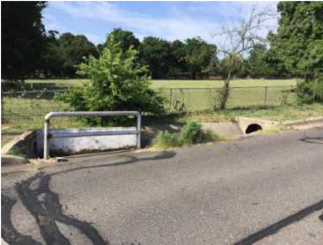
Open ditch / inlet to be improved with development. Entirely enclosed with new inlet
