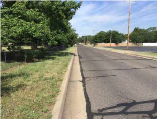
Looking west on E Main Street. Curb and Gutter existing but no sidewalk.
