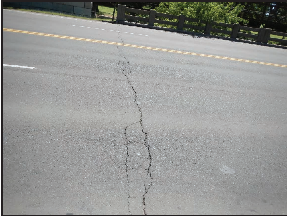
Photo 2. Asphalt Roadway Approach at East Abutment
