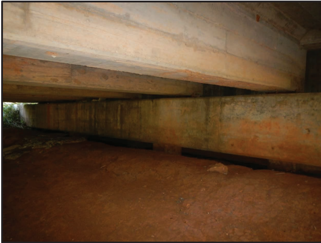
Photo 8. East Abutment Elevation (Looking East)
