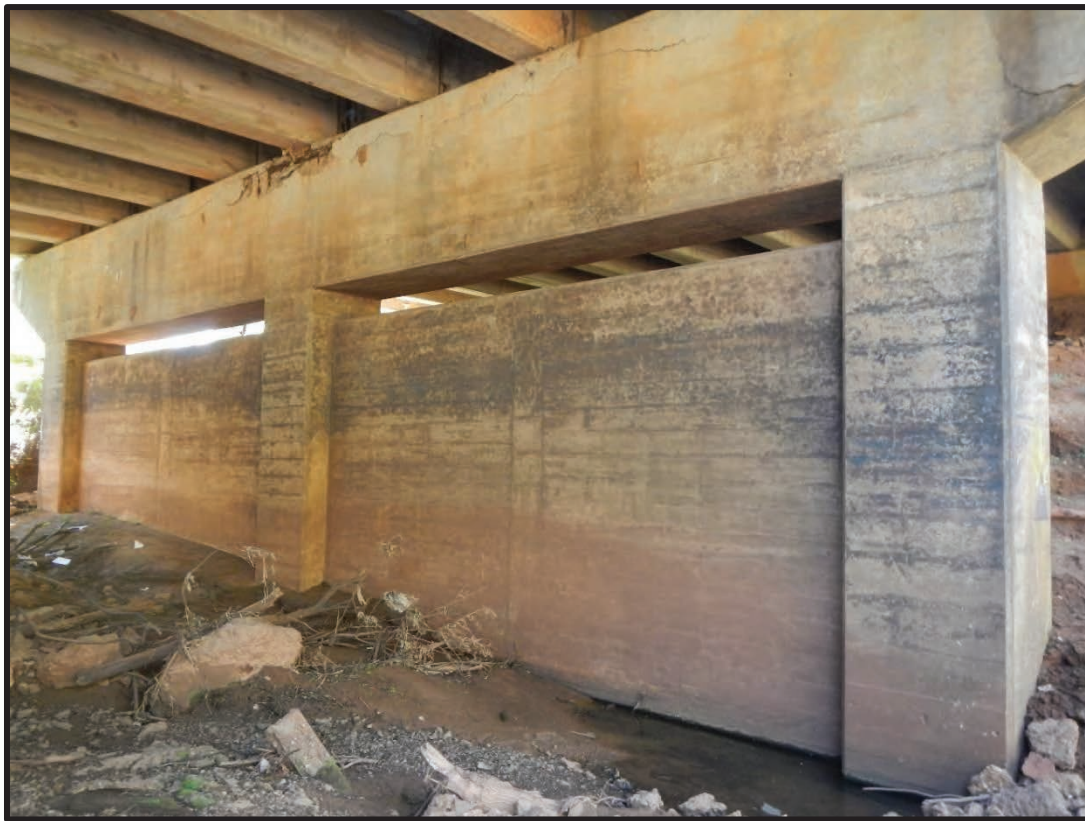
Photo 13. East Pier Elevation (Looking West)
