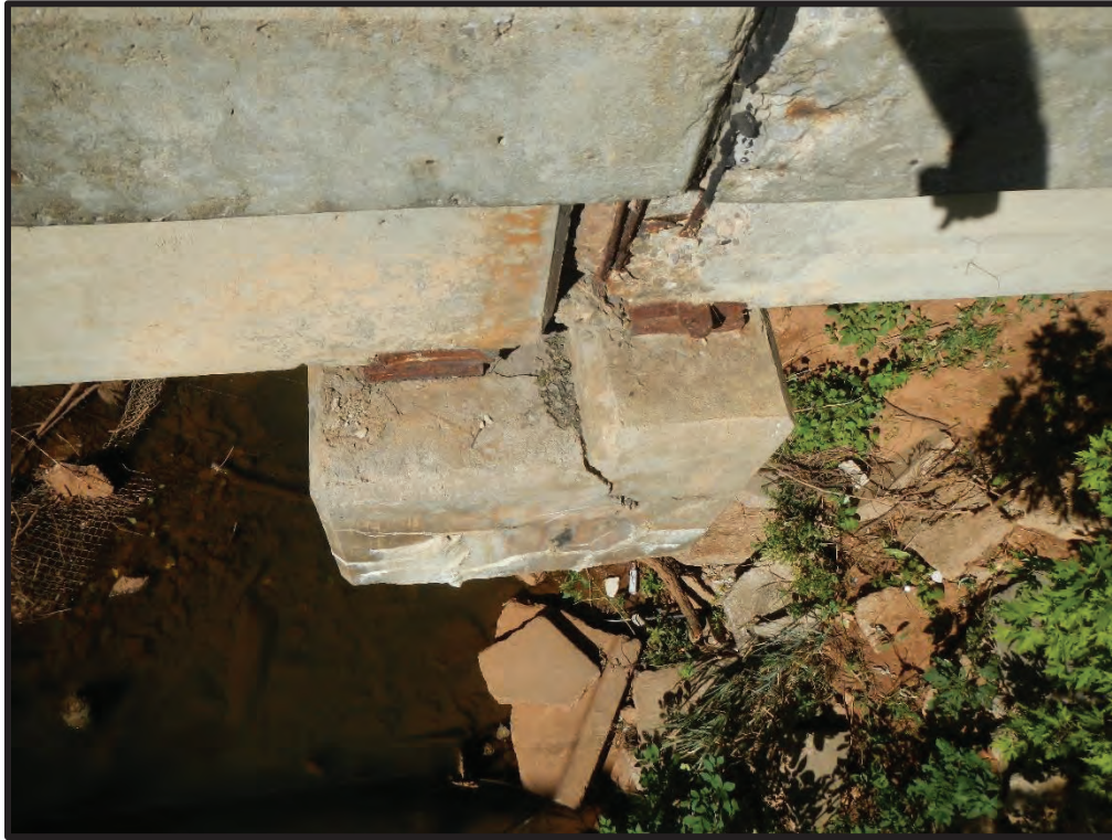
Photo 19. Spalled Girder-End
