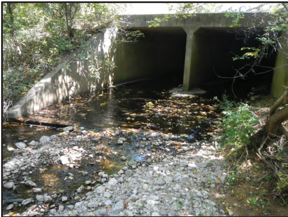
Photo 40. Typical Riprap Outlet End
