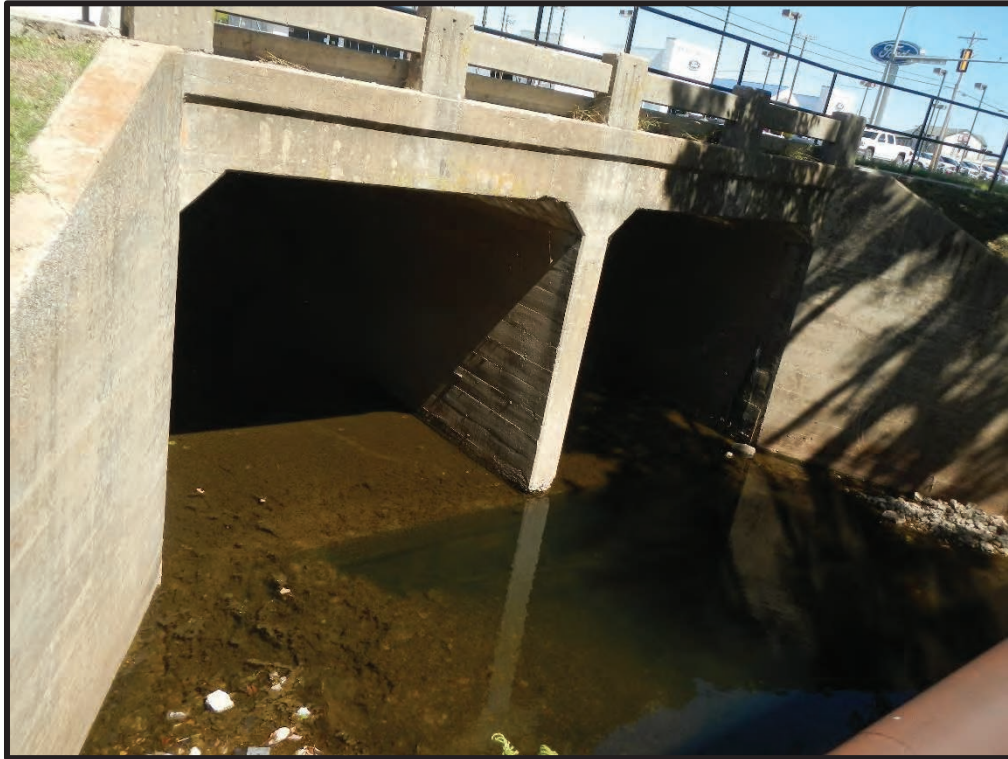
Photo 29. View of Bridge (Looking North)
