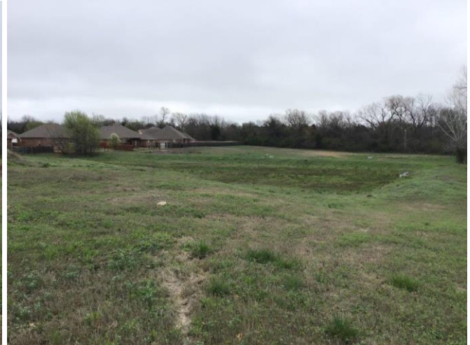
View of west detention pond
