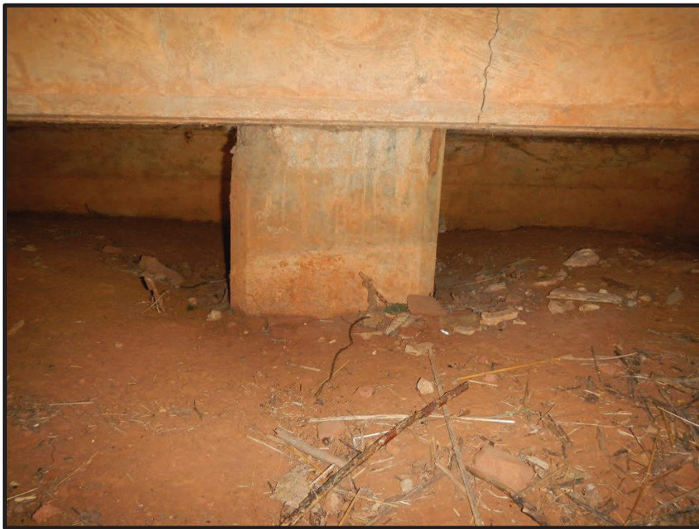
Photo 12. Close Up of Exposed Concrete Pile
