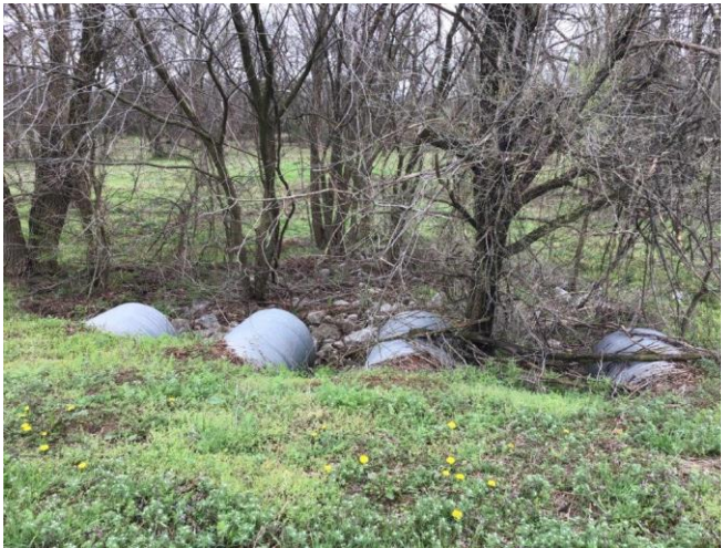
Outfall of west pond looking downstream
