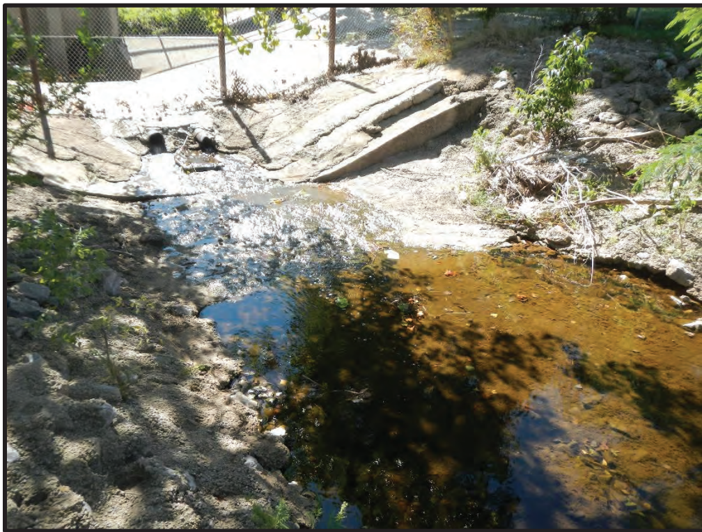
Photo 34. Typical Riprap at Inlet
