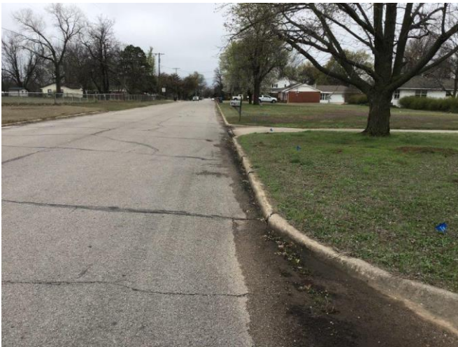
Looking south on Saint Paul Road. New proposed road, Allison Way would intersect just on the opposite side of mailbox.
