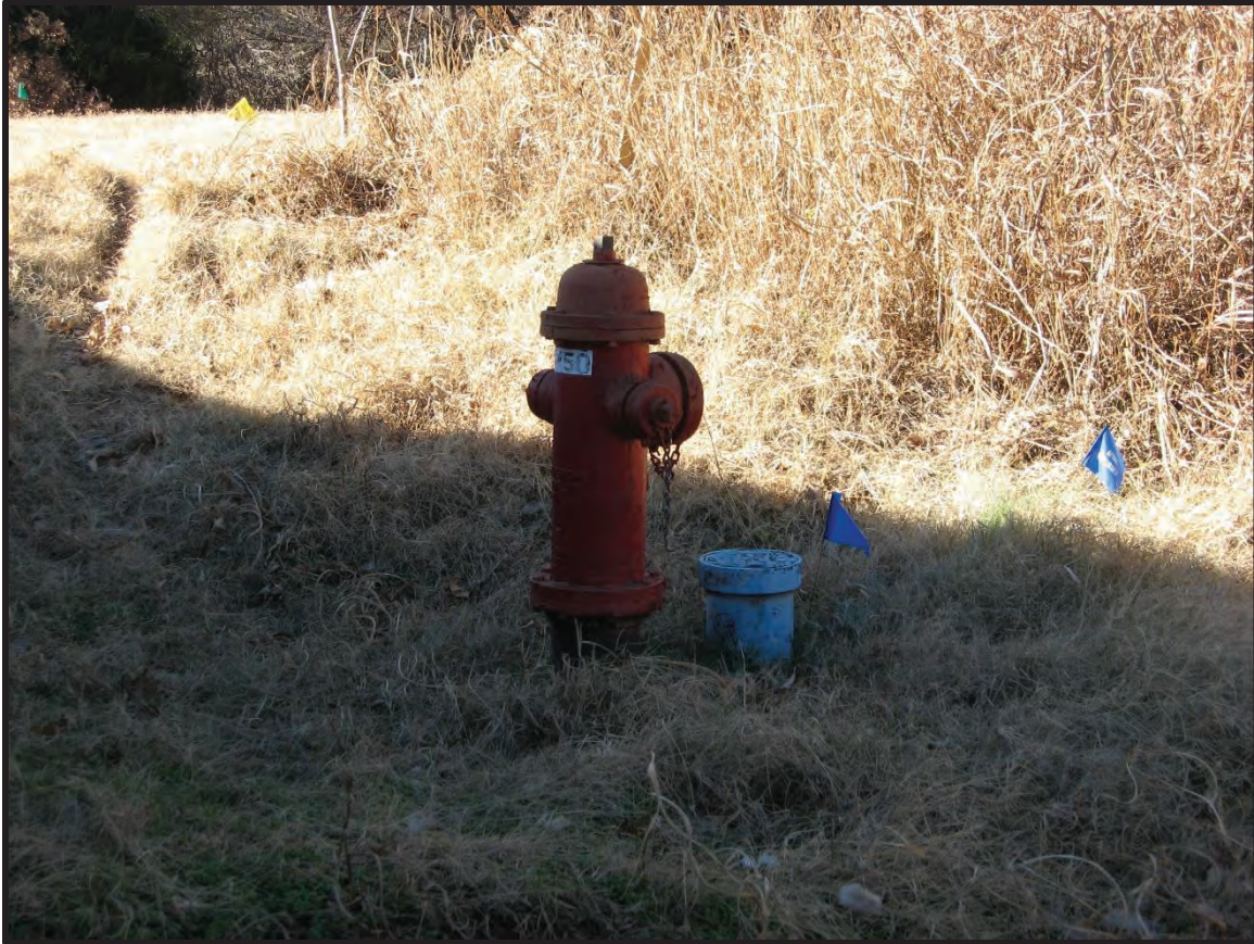
Photo 25. Fire Hydrant and Water Line at Northwest Corner of Bridge
