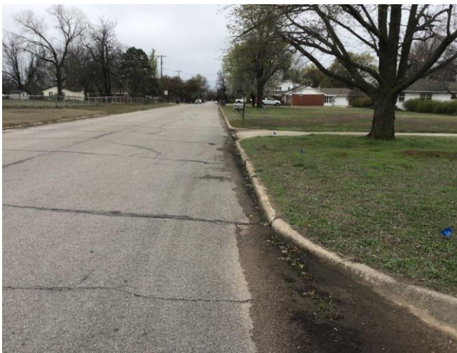
Looking south on Saint Paul Road. New proposed road, Allison Way would intersect just on the opposite side of mailbox
