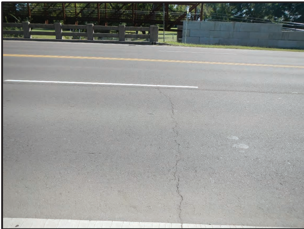
Photo 3. Asphalt Roadway Approach at West Abutment
