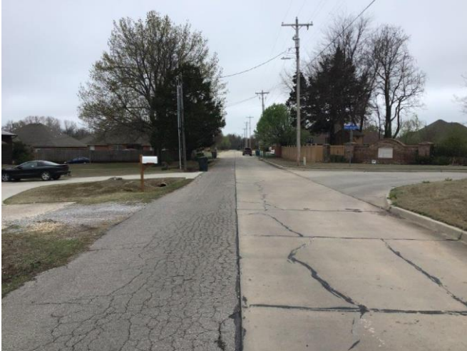
Looking south on Davidson Dr. Example of half street improvements on one side eventually being improved by another half street improvement further south.
