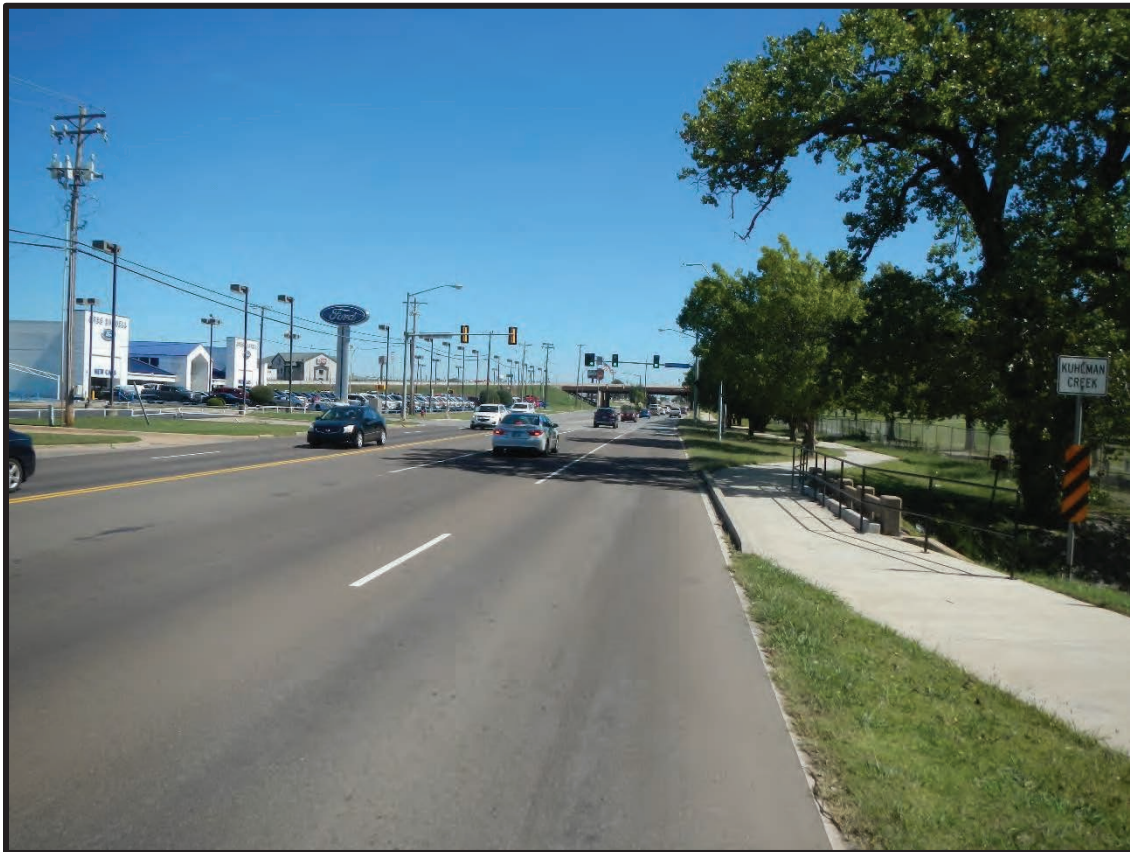
Photo 26. View of Bridge (Looking East)
