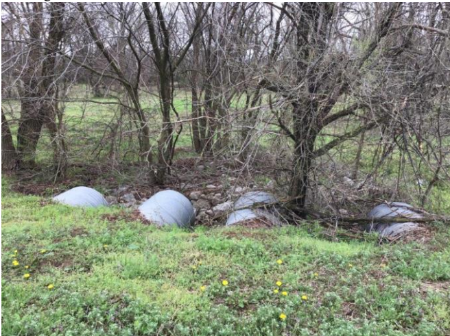
Outfall of west pond looking downstream
