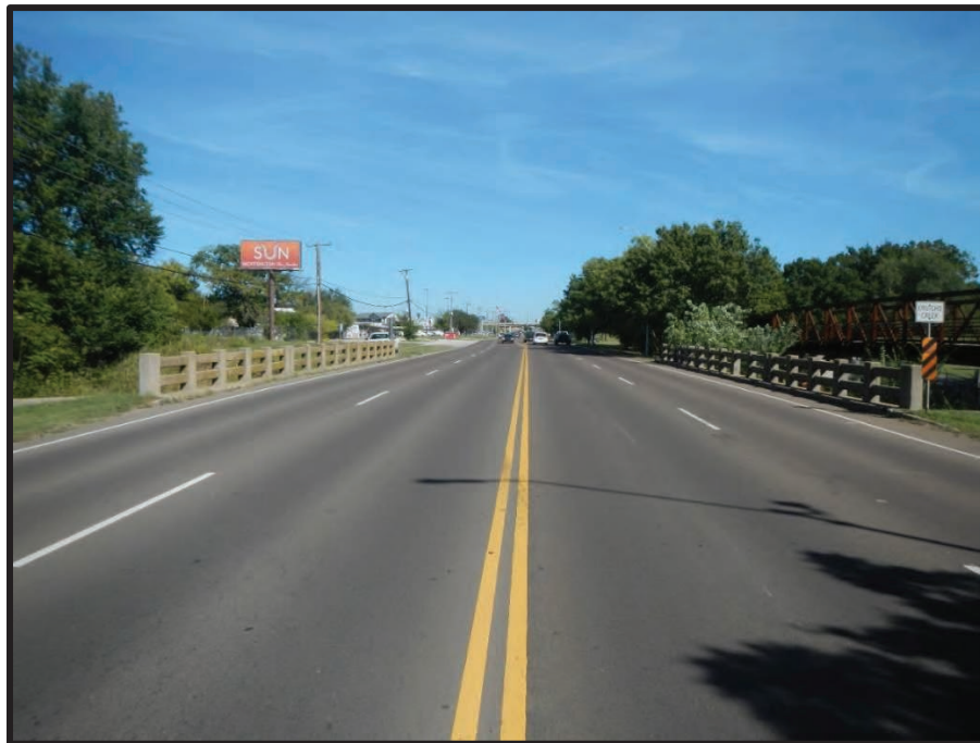
Photo 1. View of Bridge Looking East
