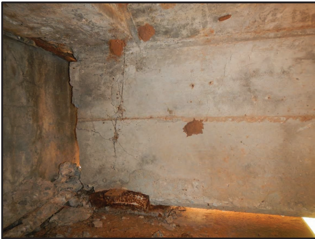
Photo 22. Close Up of Typical Bearing and Girder-End
