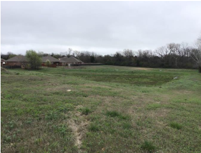
View of west detention pond
