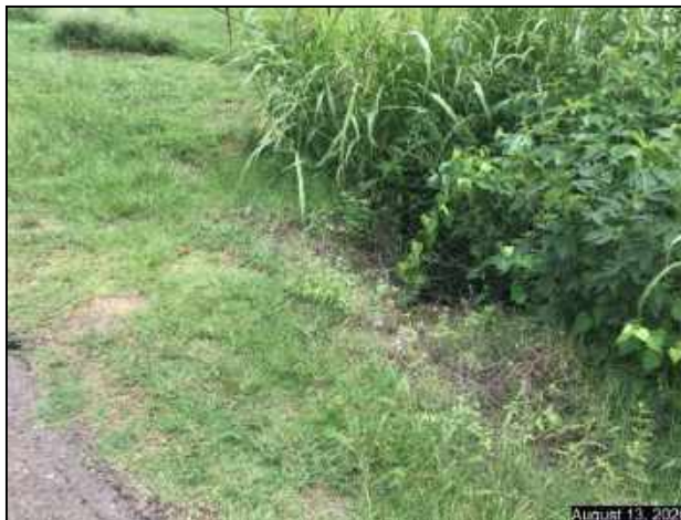
South side of SE 10 th Street, outflow of 24" cross drain opposite inlet.
