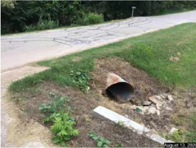
Crossdrain downstream where water flows under SE 28 th Street to the north northeast
