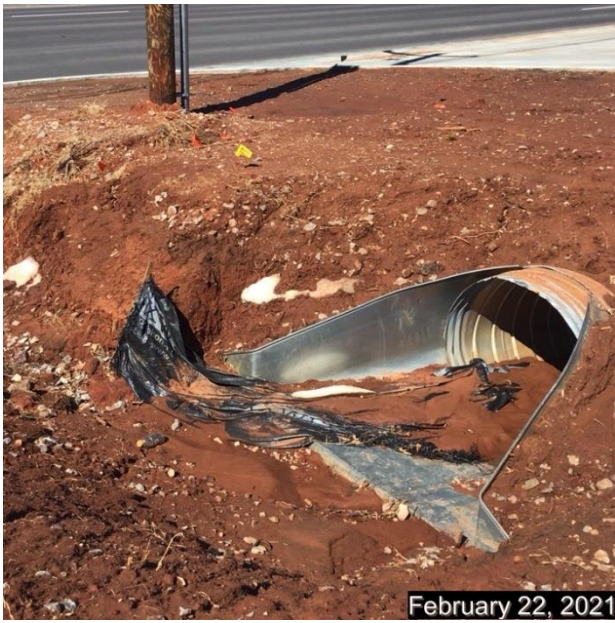
Upstream end of drainage culvert going under newly constructed driveway for Lot 1
