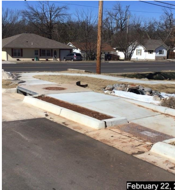
Sidewalk on northern end of property
