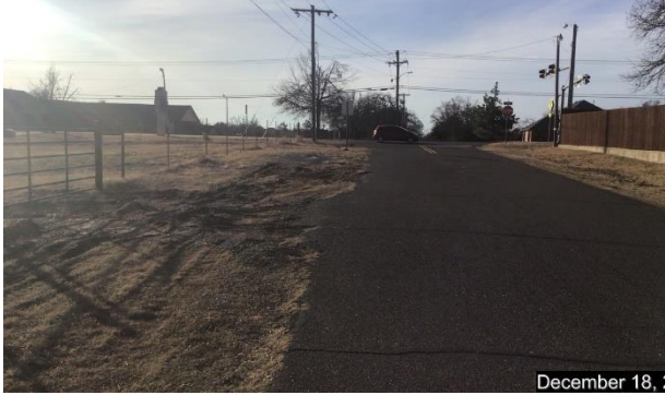
Westbound S.E. 10 th Street
