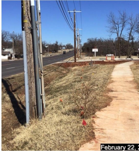
Looking north along N Douglas Boulevard from midway
