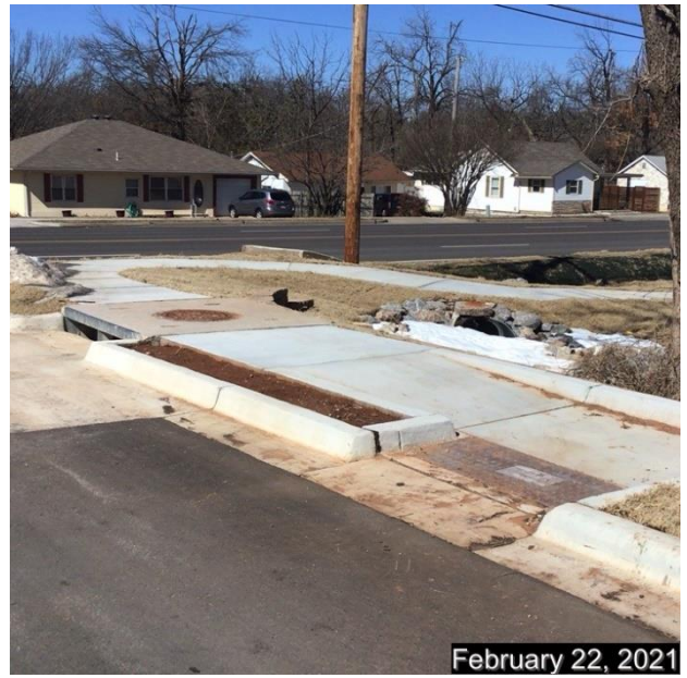
Sidewalk on northern end of property
