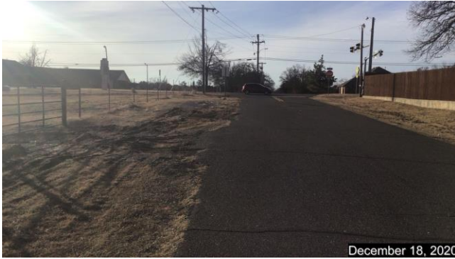
Westbound S.E. 10 th Street
