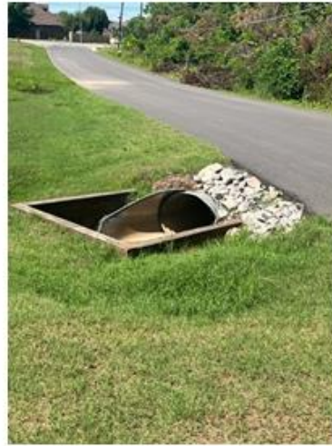
Pipe crossing upstream
