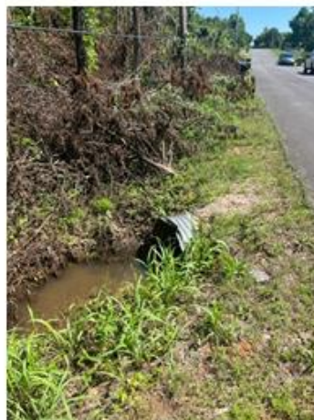
Pipe crossing downstream
