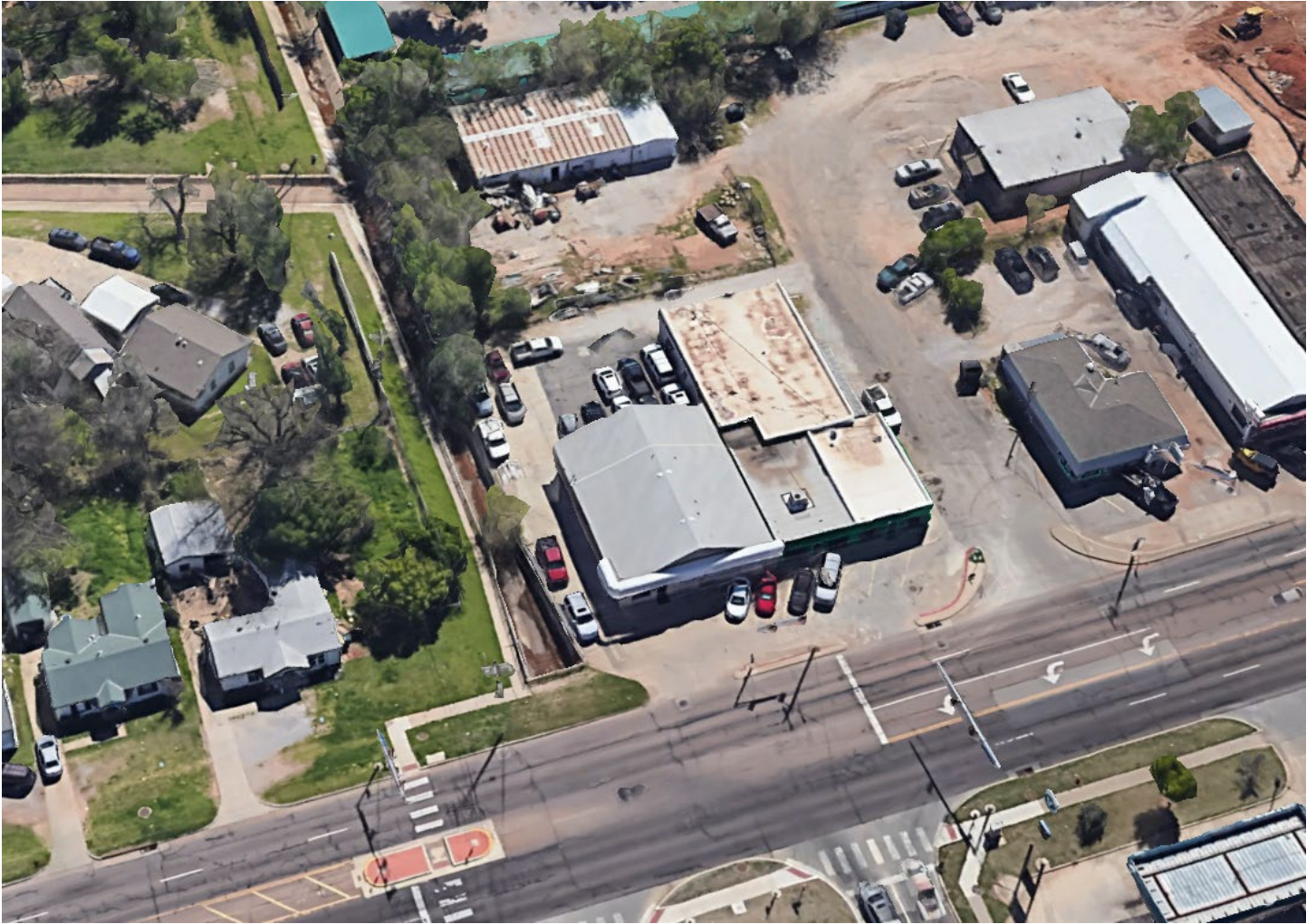
Google Earth Image of 2224 S. Air Depot Boulevard
