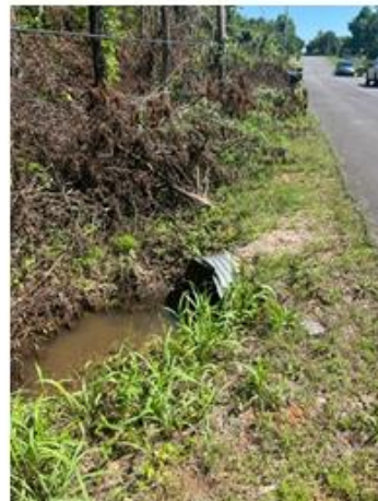
Pipe crossing downstream
