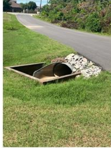
Pipe crossing upstream
