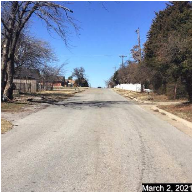
Looking north from intersection of NE 5 th Street and Oakview Drive showing curb and gutter along east side at 600/602 Oakview which was required as part of their SUP, PC-1773.
