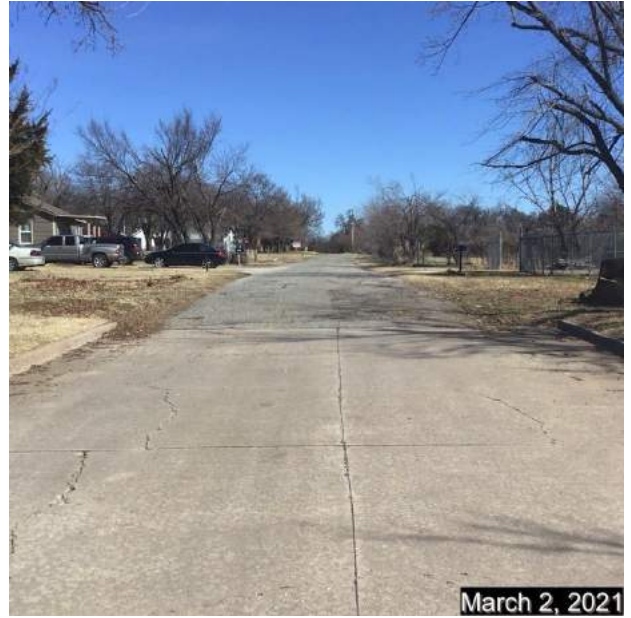
Looking east from western edge of subject plat. Subject plat is on the south side (right of picture) Shows NE 5 th Street in a city standard leading into substandard configuration along subject plat.
