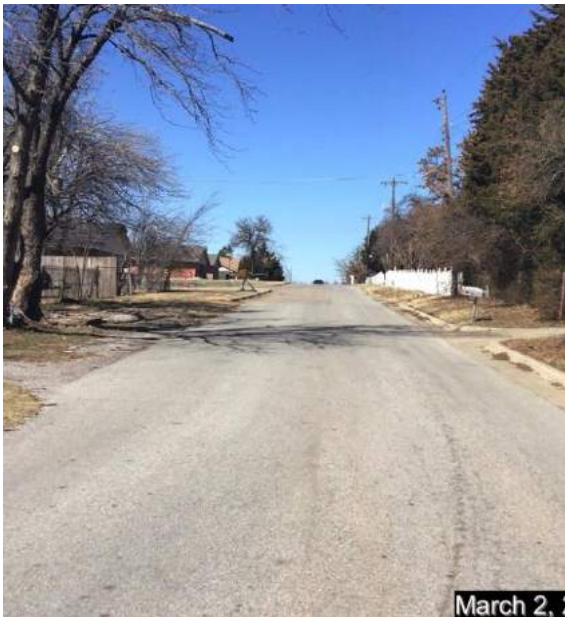
Looking north from intersection of NE 5 th Street and Oakview Drive along Oakview Drive showing substandard street but curb and gutter existing along east side
