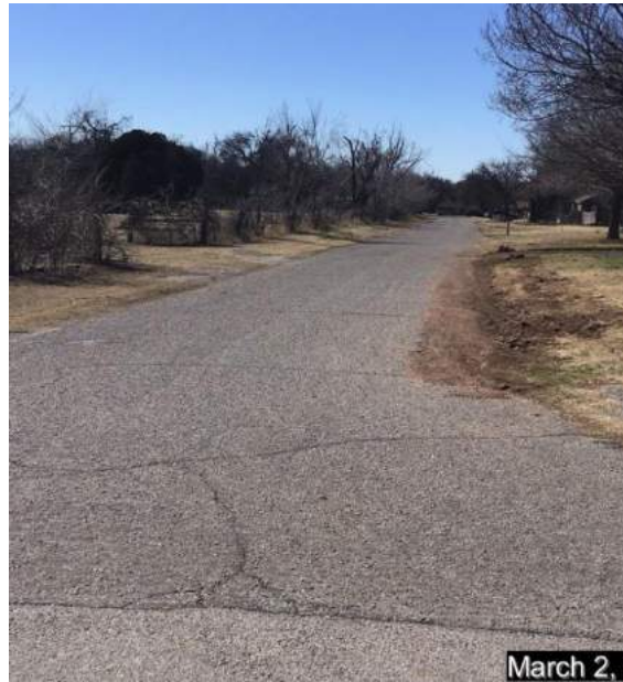
Looking west from intersection of NE 5 th Street and Oakview Drive along NE 5 th Street showing substandard street. Subject plat is on the south side (left in picture)
