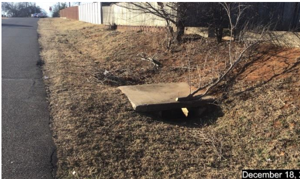
Drainage inlet on north side of S.E. 10 th Street which drains to the south
