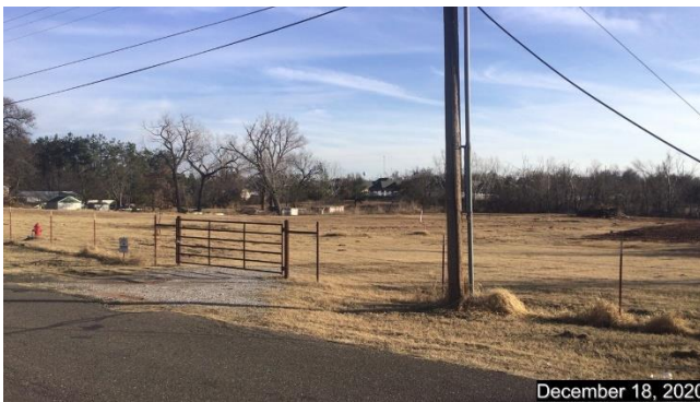
Eastern portion of proposed development, showing waterline which is not yet accepted by City
