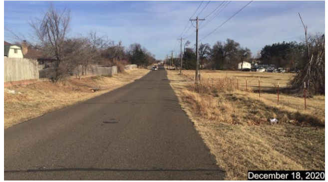
Eastbound S.E. 10 th Street
