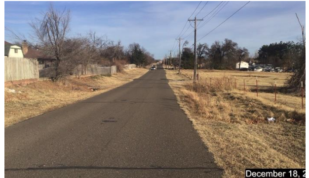
Eastbound S.E. 10 th Street
