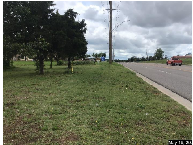
Looking south from the S Post Road grade goes uphill
