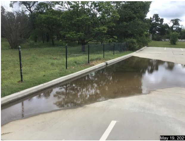
Detention area of church parking lot showing outfall onto subject property
