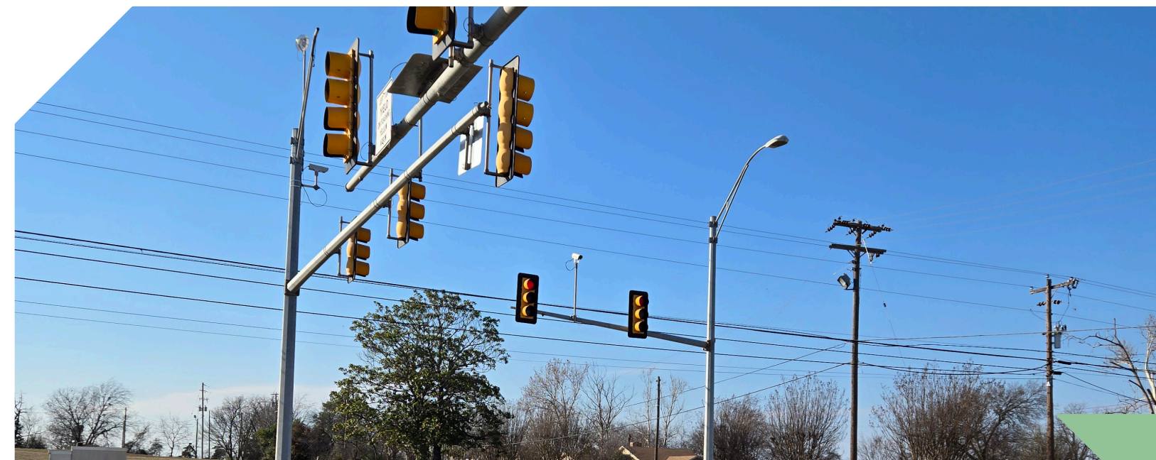
Intersection at Highway 37 & Tiger Boulevard
