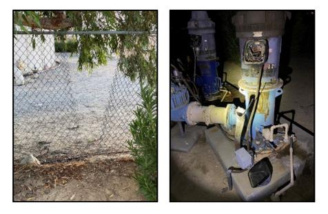
Rehabilitation of Well 33 and reservoir overflow has begun. Brushing and bailing are complete and the chemical rehabilitation process began in December 2022. The focus intake pumping is currently underway during the first week of January 2023.
