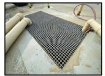
Staff repaired the effluent discharge piping for the west clarifier at Desert Crest WWTP. The west tank is back to fully operational if we ever needed to use it.
