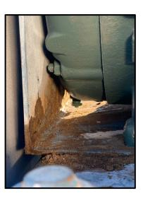
Staff replaced the south cyclone rubber liner that feeds a grit separator. The rubber liner inside had worn down from grit over the years.
