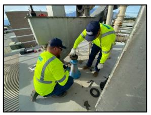
Staff replaced the floats for the sump pump that receives the discharge filtrate from the belt press, and it is now back to normal operation. A cross beam was installed to be able to cut the grating for the pit in half, allowing easier access for maintenance into the pit.
