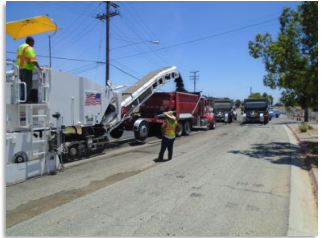
City of Calimesa | Citywide Pavement Rehabilitation
