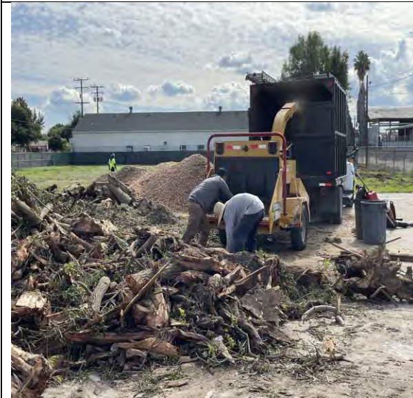
N.R.Development crew mobilized and commenced demolition operation
