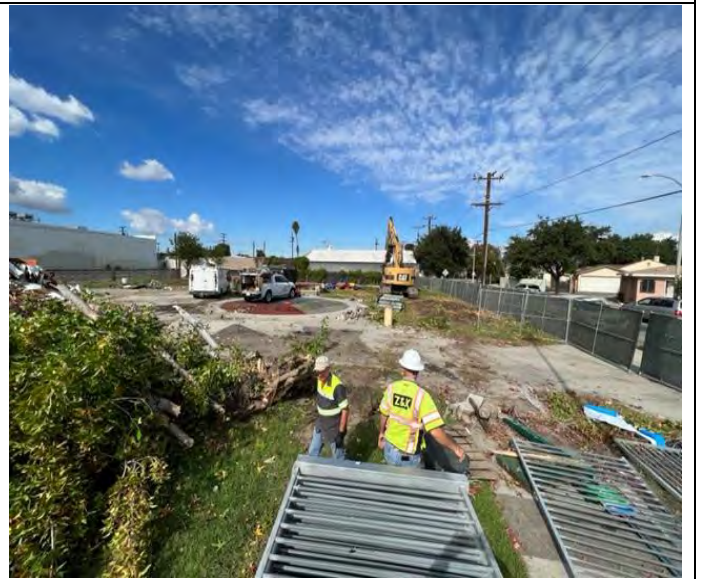
N.R.Development crew mobilized and commenced demolition operation
