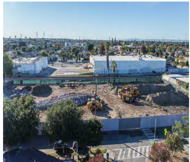
N.R. Development crew mobilized and continued demolition operation
