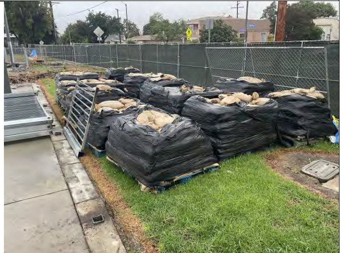
BMPs stored on site prior to commencement of Demolition and site clearing
