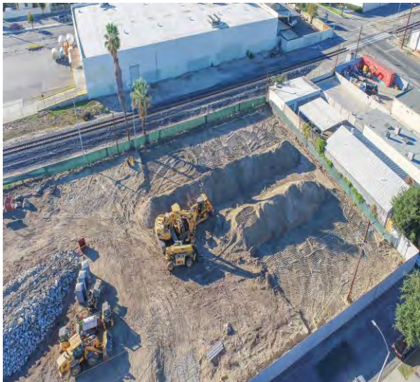
N.R. Development crew mobilized and continued demolition operation
