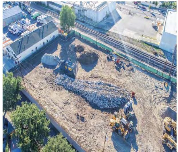
Demolition and site clearing continued on November 28 th , 2022
