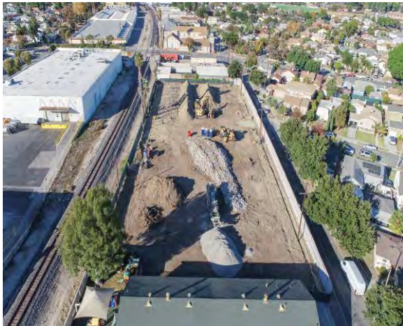
Demolition and site clearing continued on November 28 th , 2022
