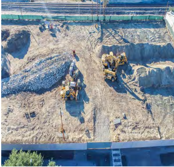
Demolition and site clearing continued on November 28 th , 2022
