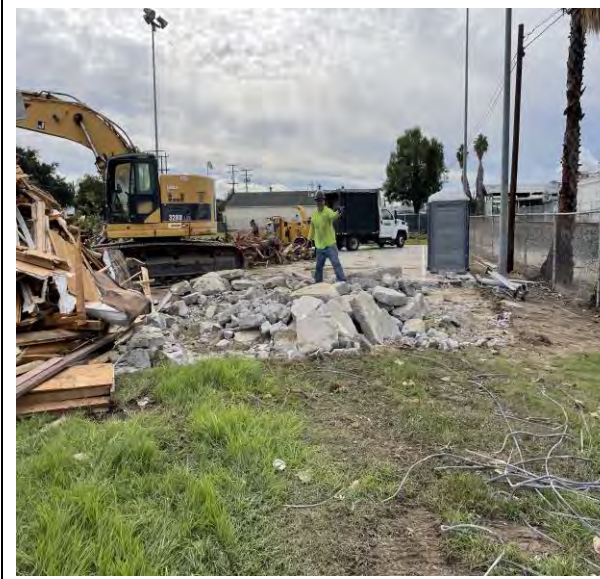
Demolition and site clearing commenced on Tuesday November 1 st , 2022
