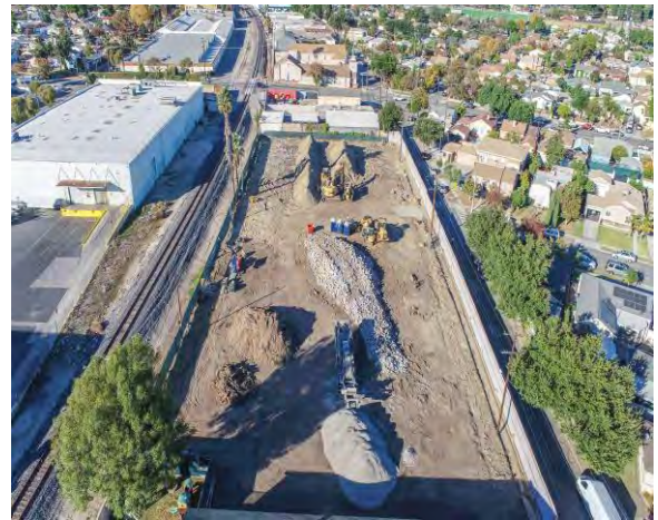
Demolition and site clearing continued on November 28 th , 2022
