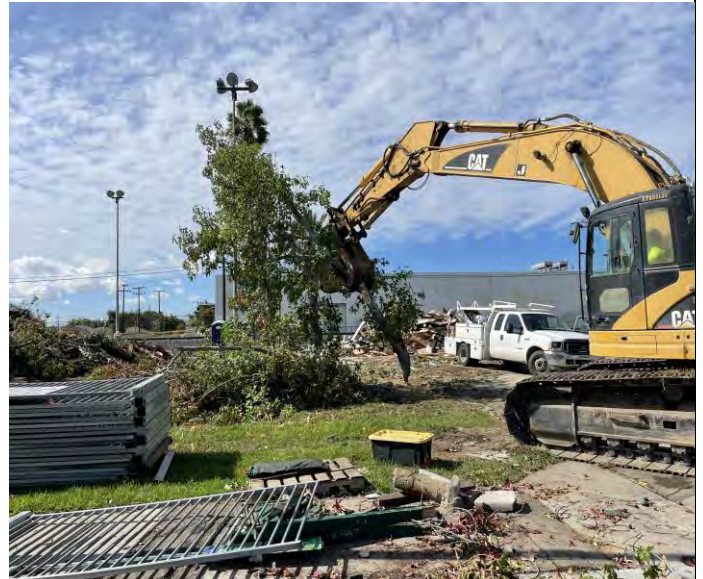
Demolition and site clearing commenced on Tuesday November 1 st , 2022
