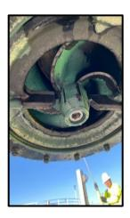
Staff inspected the south grit classifier at the Horton WWTP, which had a clogging issue preventing it from discharging grit into the grit bin. Staff pulled out a decent size rag out of the classifier. Staff is working on getting replacement augers for both the north and south grit classifier. These augers are original and have been in service for over 20 years.
