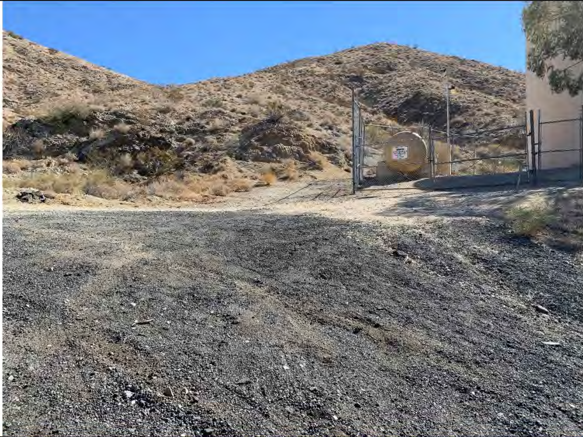
Photo 3. Looking east at the northern edge of the existing reservoir tank and the general location of the new tank.
