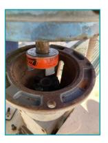
Staff inspected and cleaned the sprayers for the auger monster located at the headworks. These sprayers help remove organic material from rags that enter the plant.
