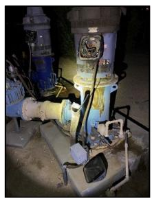
Rehabilitation of Well 33 and reservoir overflow has begun. Brushing and bailing are complete and the chemical rehabilitation process began in December 2022. The focus intake pumping is currently underway during the first week of January 2023.
