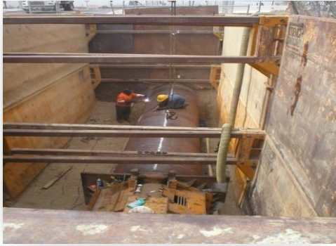
Figure 1. We thrive in creating solutions to challenging problems. The 1720 Zone West project required deep pit bore and jack construction under an active freight rail line, requiring significant permitting efforts and additional construction coordination.
