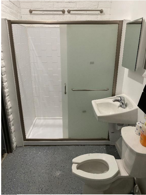
NEW SHOWER AND RESTROOM, POST CONSTRUCTION
