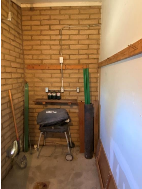
PREVIOUS UTILITY ROOM, PRE-CONSTRUCTION
