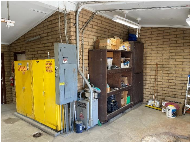
FORMER STORAGE AREA, PRE-CONSTRUCTION
