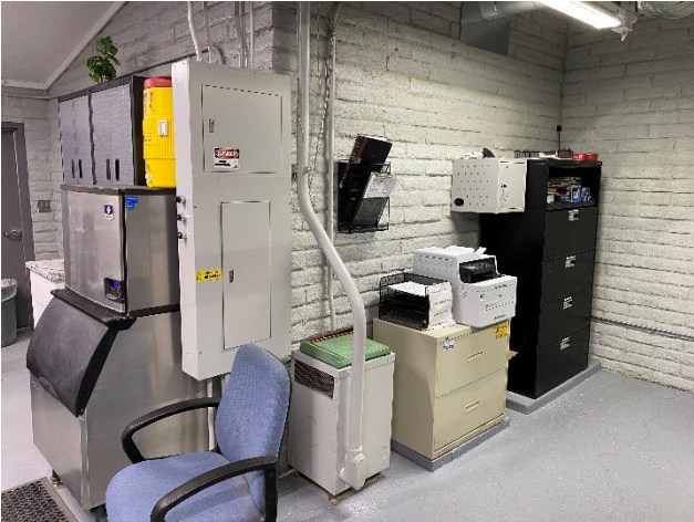
NEW OFFICE AREA, POST -CONSTRUCTION
