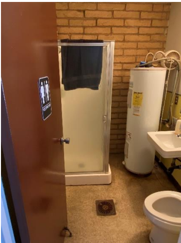
PREVIOUS SHOWER AND RESTROOM, PRE-CONSTRUCTION
