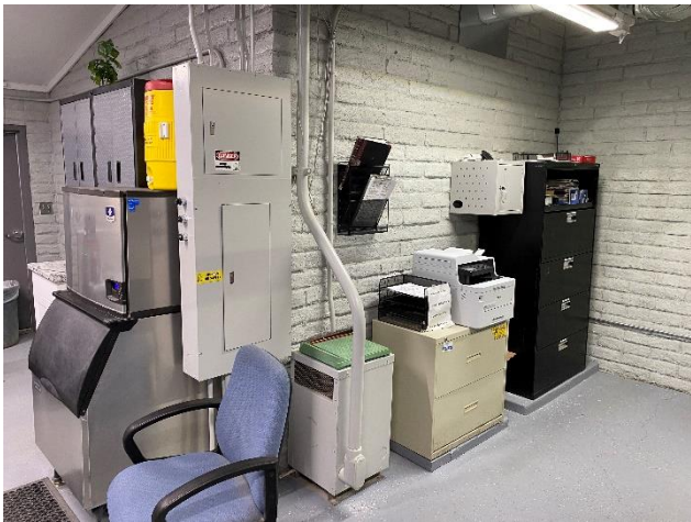
NEW OFFICE AREA, POST -CONSTRUCTION
