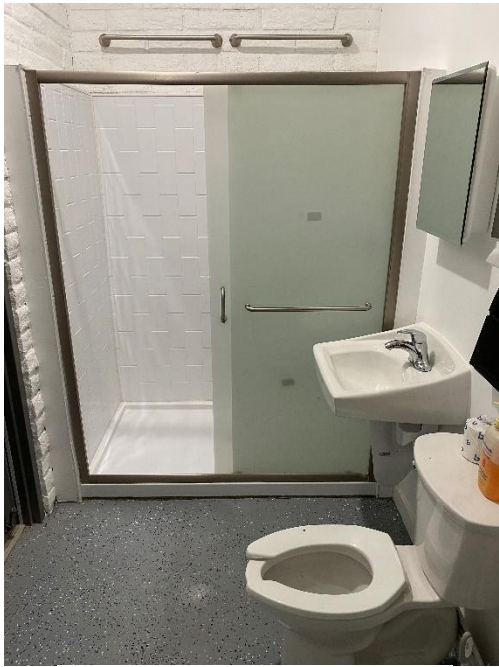
NEW SHOWER AND RESTROOM, POST CONSTRUCTION
