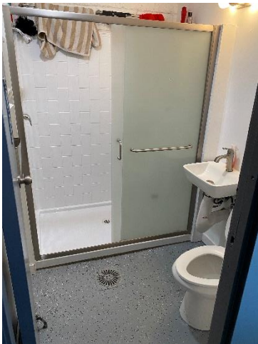
NEW SHOWER AND RESTROOM, PRE-CONSTRUCTION
