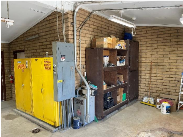
FORMER STORAGE AREA, PRE-CONSTRUCTION
