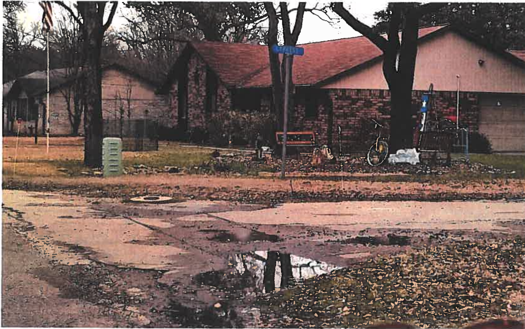
Figure 9. Intersection of Cypress Court and Hackberry Court
