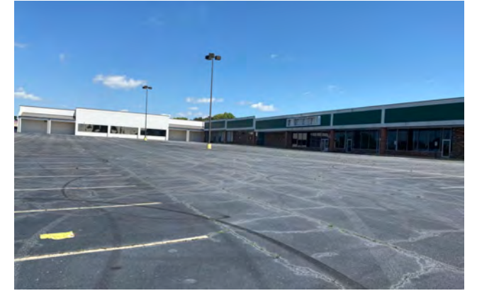
View of Existing Building Looking North
